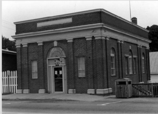
Bank of Louisa, Mineral Historic District
