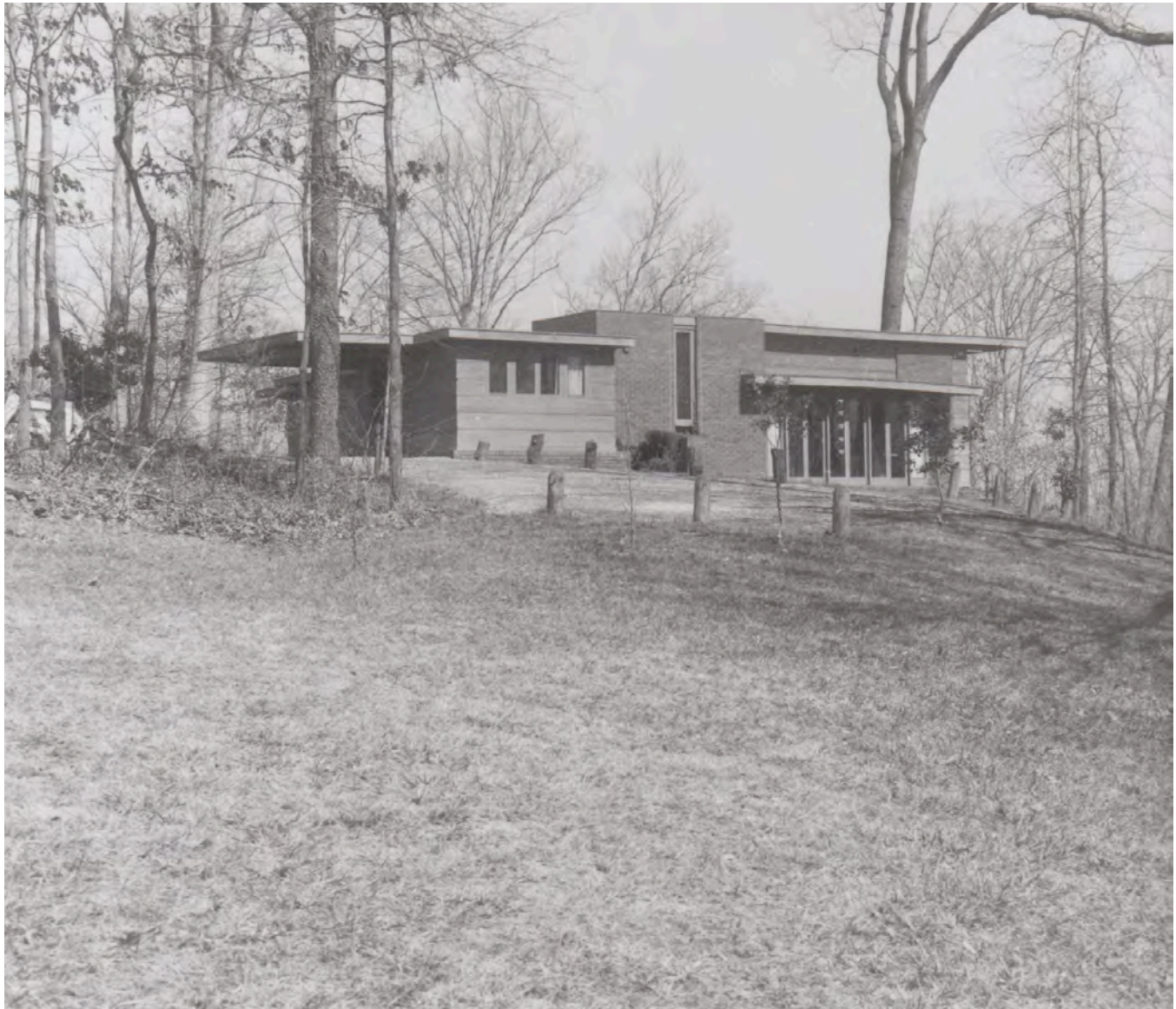
Figure 29. Pope-Leighey House following relocation to Woodlawn, circa 1970
