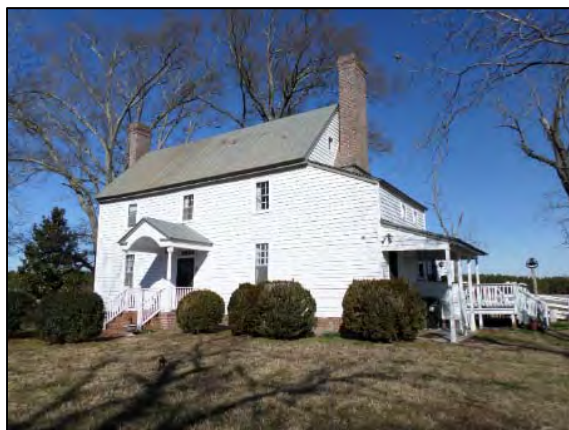
The Vineyard, South façade
