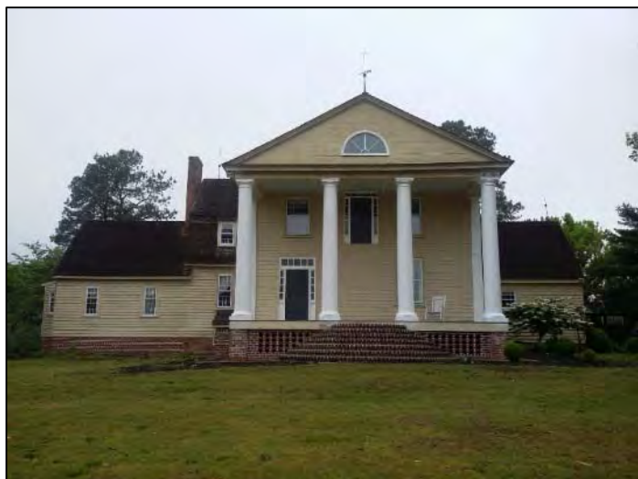
Marlborough, East facade
