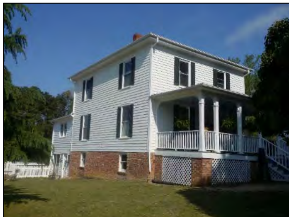
The Institute, East Façade
