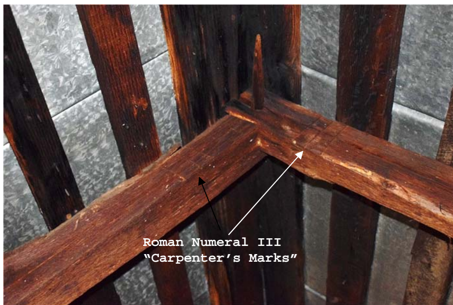
Figure 3: Attic Carpenter's Marks
