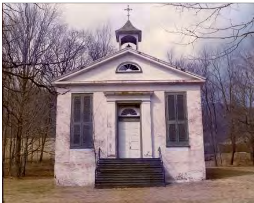
6. The Warm Springs Episcopal Church, constructed in 1851 near the site of the Warm Springs pools, as it appeared prior to being renovated as a residence. The belfry was moved to the church from the ca. 1842 courthouse. (Courtesy of the Bath County Historical Society)
