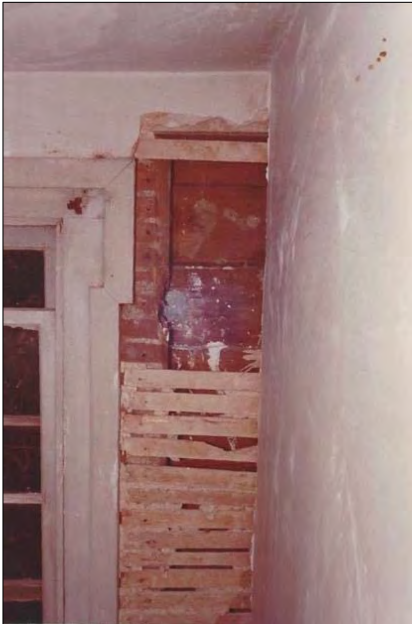
Historic Photo 5 of 5 Detail of corner, second-story bedroom: damaged post and lath, hole in weatherboarding caused by 1865 shelling.
