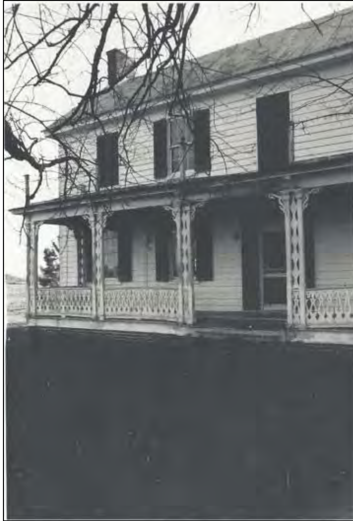
Historic Photo 1 of 5 View of Greenfield façade and 1873 porch
