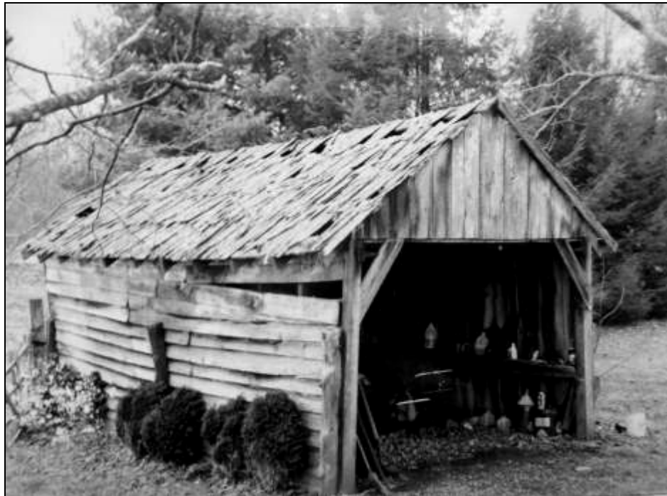
10. Early Twentieth-Century Garage Formerly Located In West Side Yard. Source: Susan Bull Ryan.
