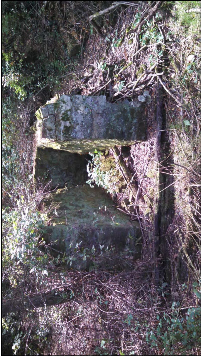
Figure 26. Spring House, Masonry walls.
