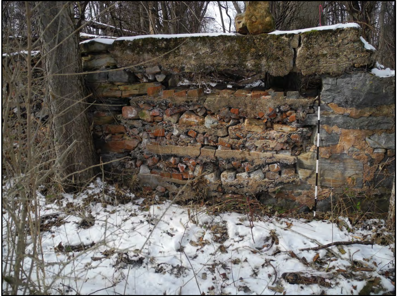
Figure 18. Barn Site, Brick and mortar-filled opening in front (east) wall (scale = 1 meter).
