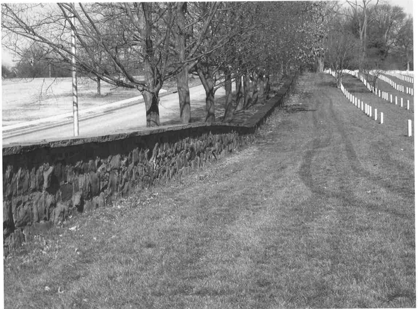
Photo 20. View north along Seneca sandstone boundary wall.
