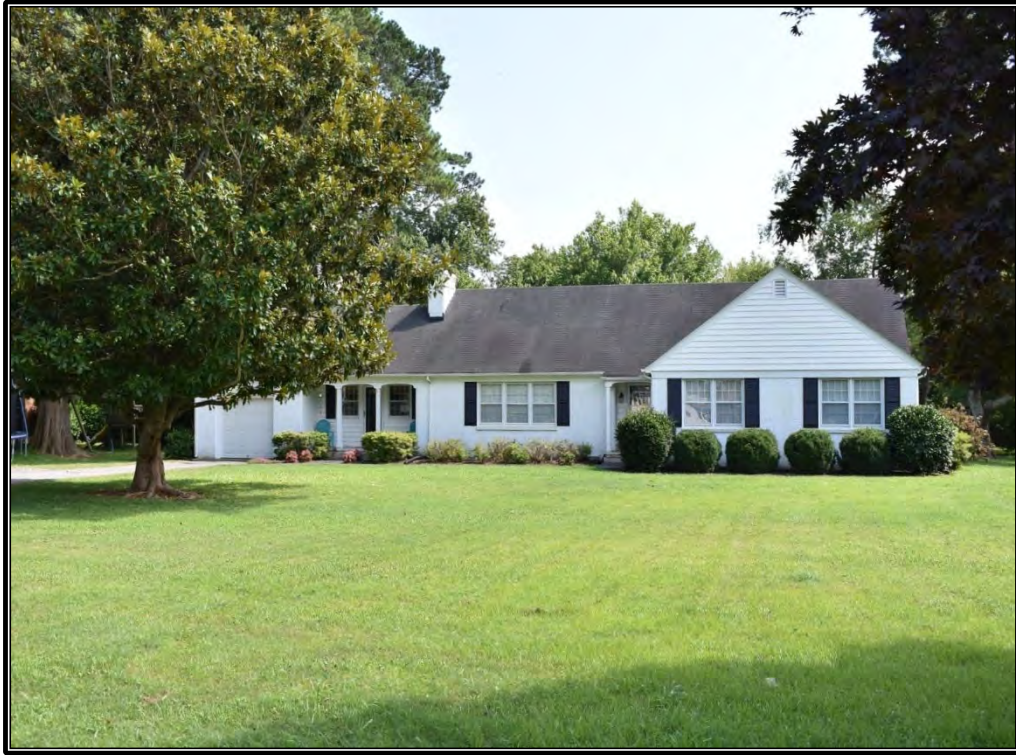
Figure 62. Ranch House (1960), 1505 Bayshore Drive East (134-5518)
