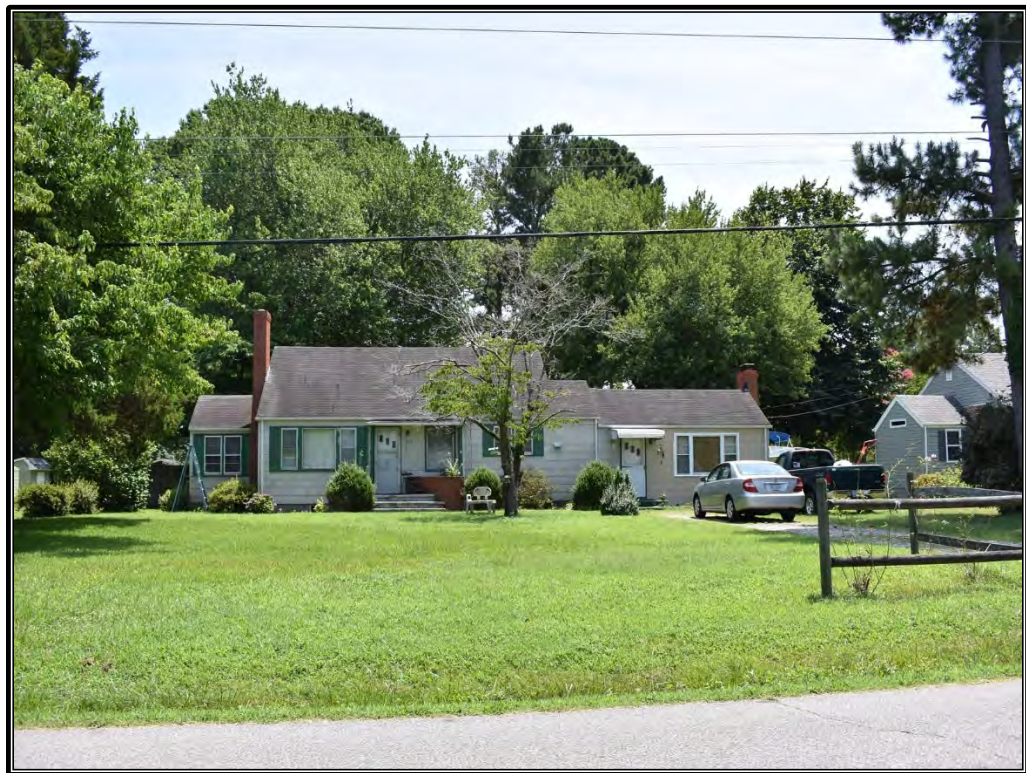
Figure 39. Minimal Traditional house (1950), 1154 Old Kempsville Road (134-5510)
