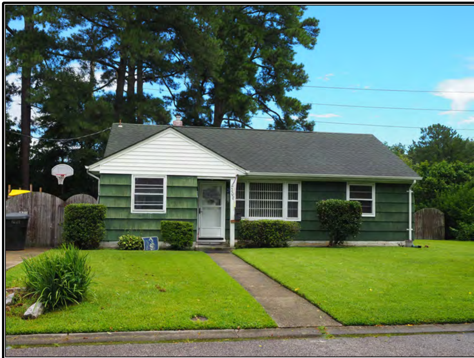
Figure 106. Single-family residence with wood shingles and windows featuring horizontal muntins (1958), 208 N. Lynnrivier Drive (134-5581)
