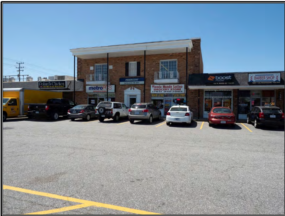
Figure 10. London Bridge Shopping Center (c. 1951-1971), 315 N Great Neck Road (134-5422)
