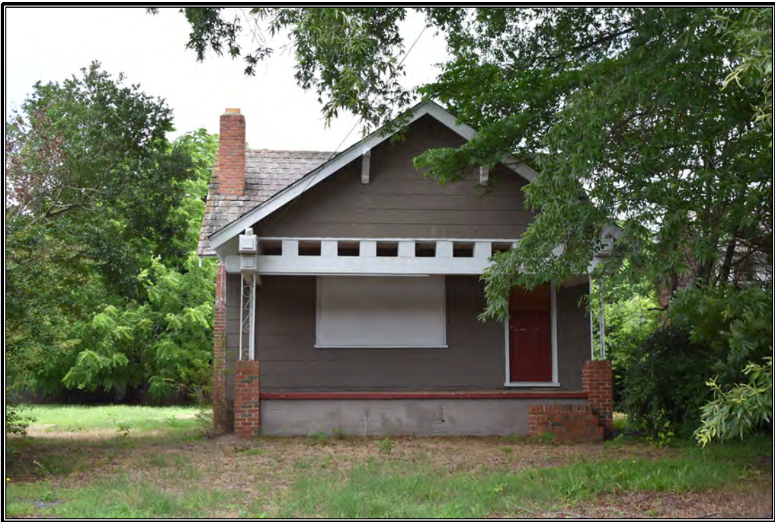
Figure 74. Bungalow (1940), 4772 First Court Road (134-5542)
