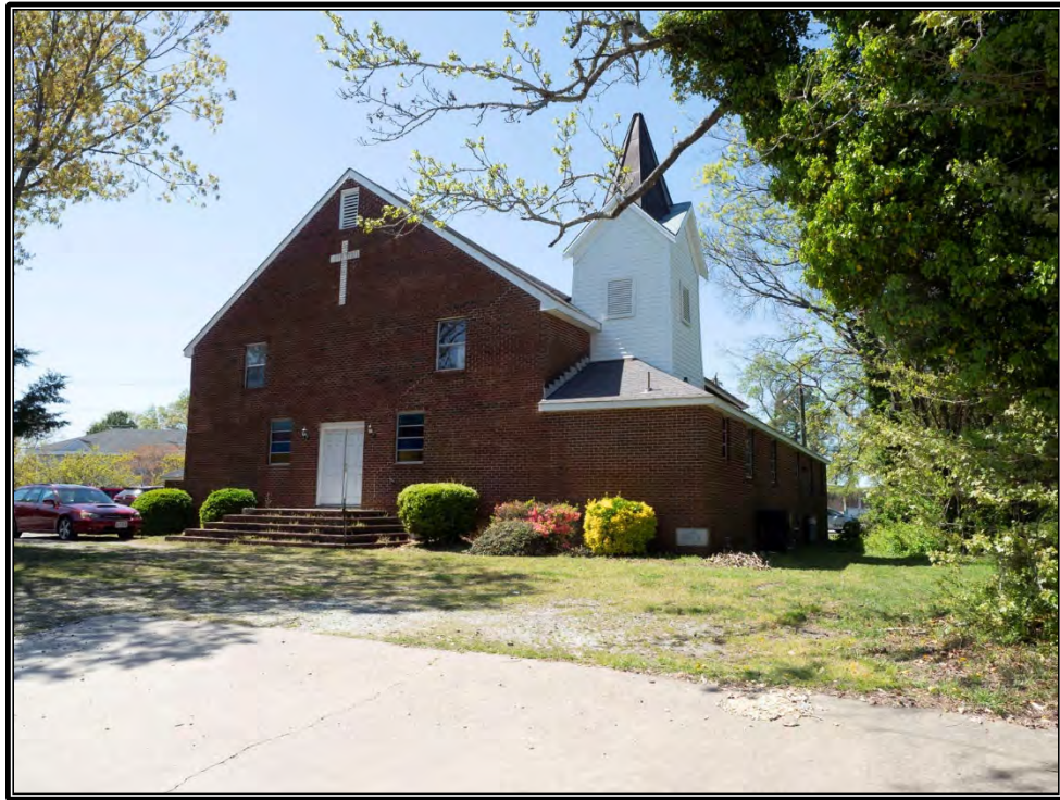
Figure 21. Morning Star Baptist Church (c. 1892), 4800 First Court Road (134-0970)
