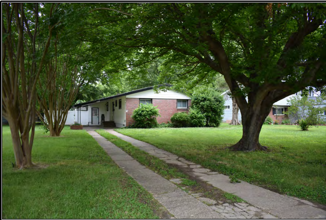
Figure 97. Contemporary Style House with Carport (1954), 5520 Forest View Drive (134-5462)
