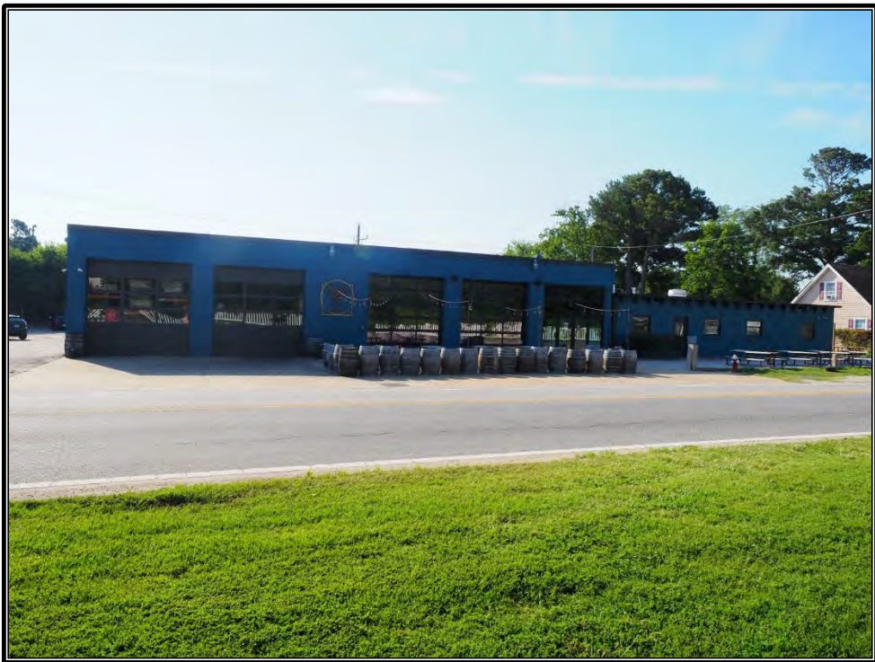
Figure 18. Former Chesapeake Volunteer Fire Department (c. 1962), 2444 Pleasure House Road (134-5478)
