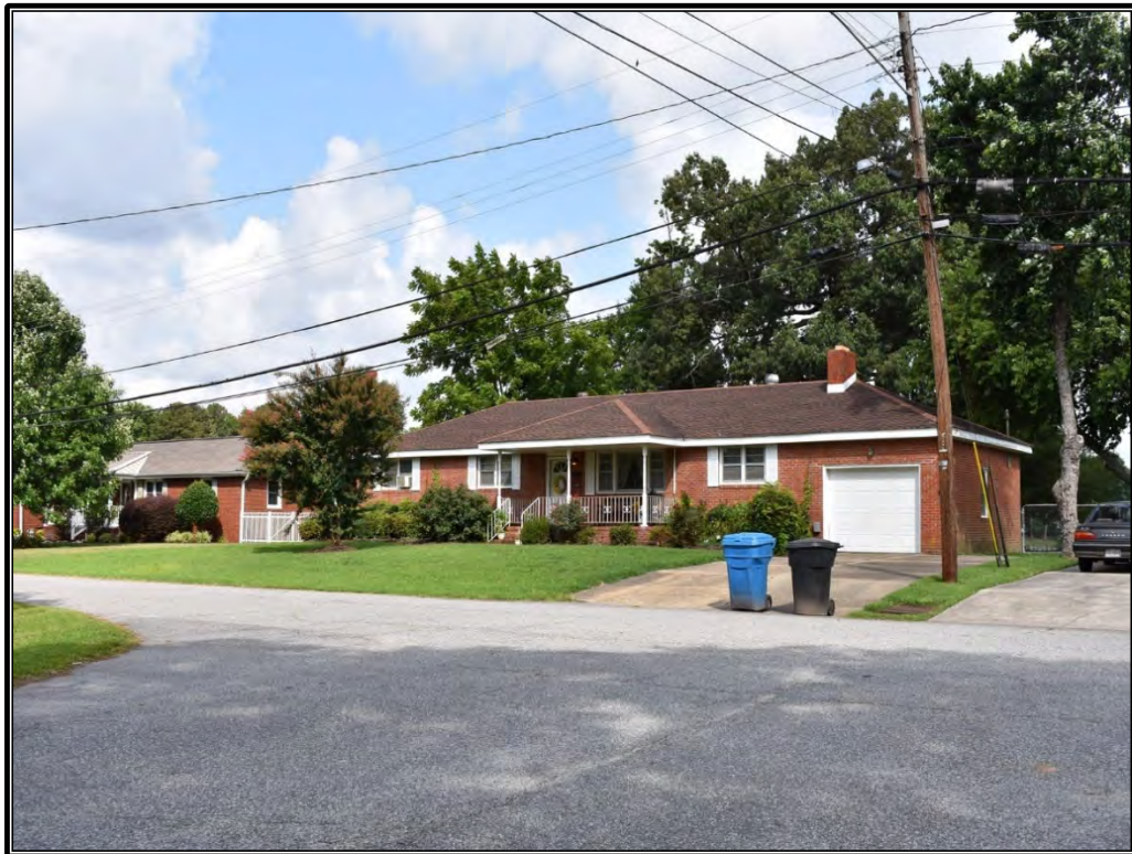
Figure 131. Ranch-style House (1963), 5148 Overland Road (134-5440)
