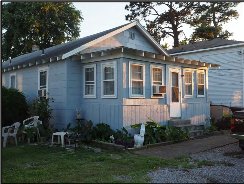
Figure 91. One-story, gable front vernacular cottage, 4601 Lookout Road (134-5476)
