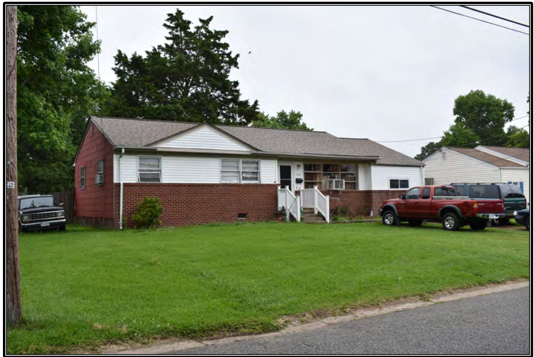
Figure 110. Minimal Traditional House (1960), 5556 Shadowwood Drive (134-5528). This example is clad with three materials, retains its historic wooden windows, and features a picture window at the front. The garage bay (right) has been modified.
