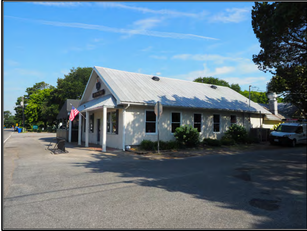
Figure 90. Commercial Building, now Hell's Kitchen Restaurant, 4600 Lookout Road (134-5475)
