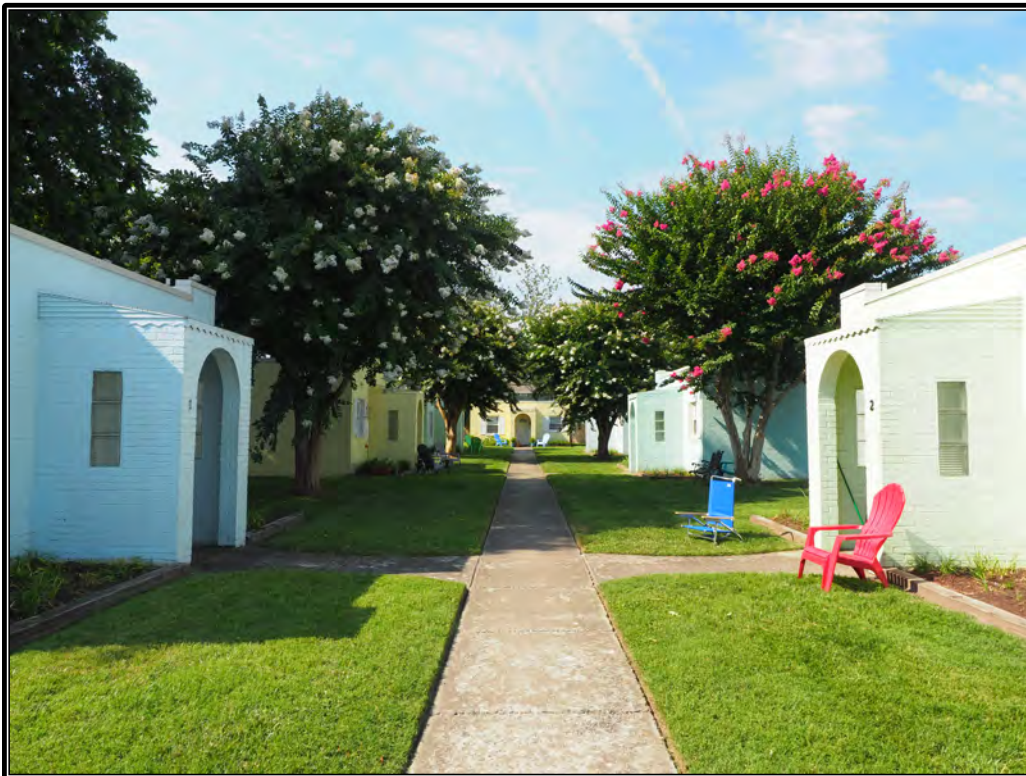
Figure 93. Brick cottages, 4489 Lookout Road (134-5479)
