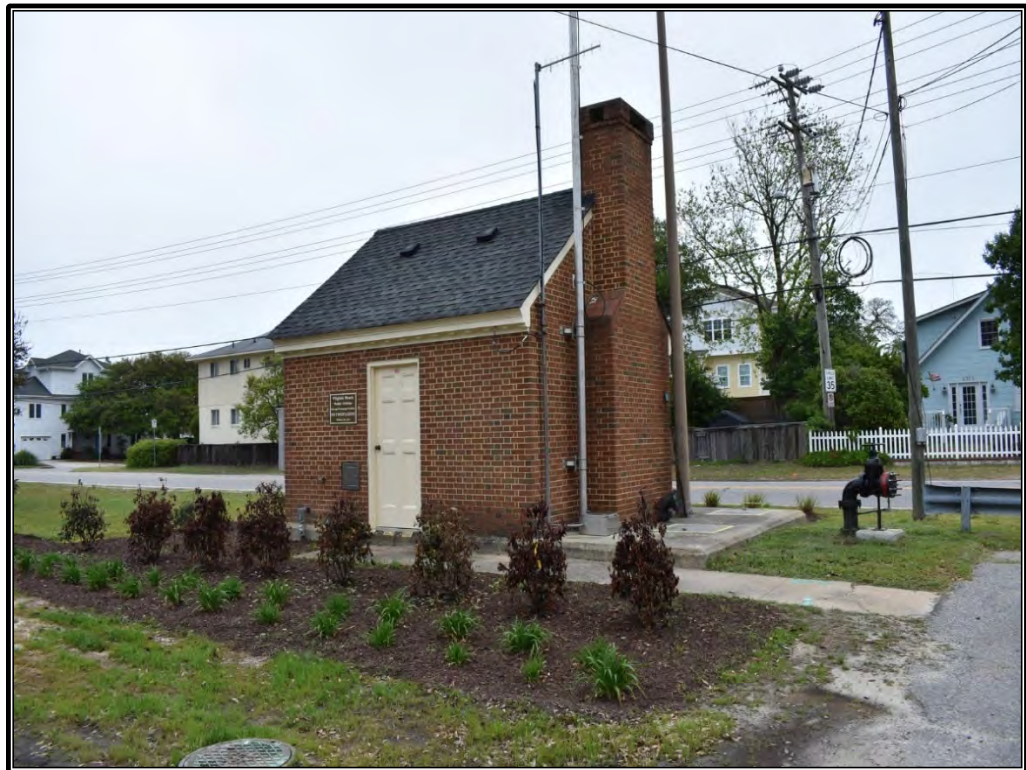
Figure 16. City Pump Station (c. 1965), 4802 Atlantic Avenue (134-5400)
