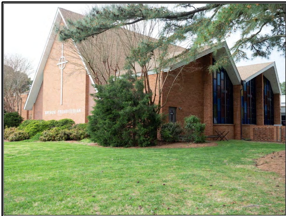
Figure 22. Bayside Presbyterian Church (c. 1964), 1400 Ewell Road (134-5416)
