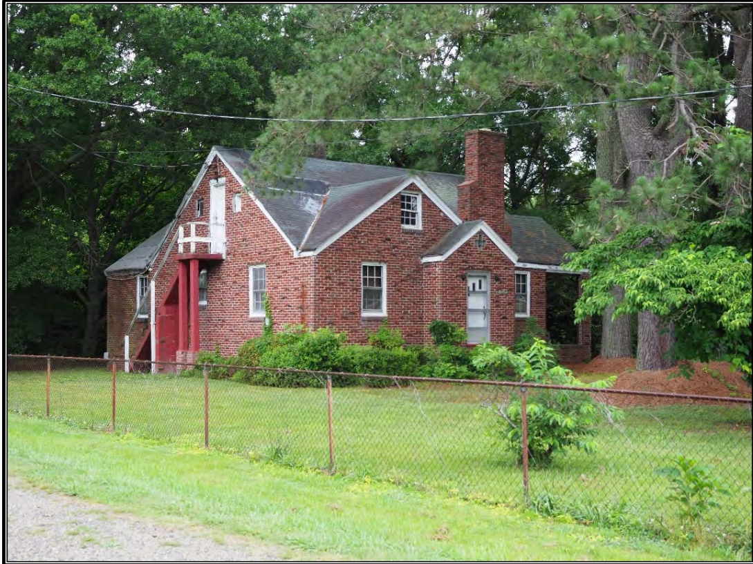
Figure 82. Minimal Traditional dwelling with skintled brick (1952), 5852 Burton Station Road (134-5463)
