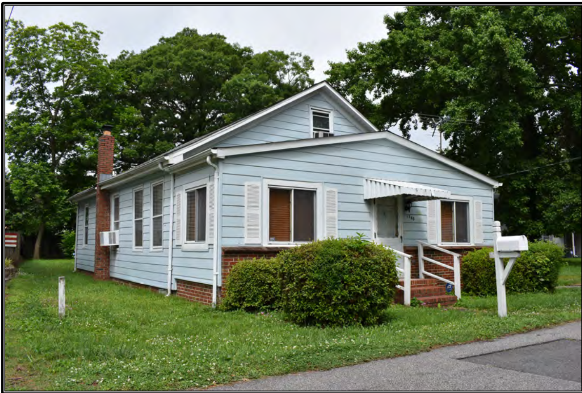
Figure 115. Vernacular Dwelling (1940), 1565 Frost Road (134-5548)
