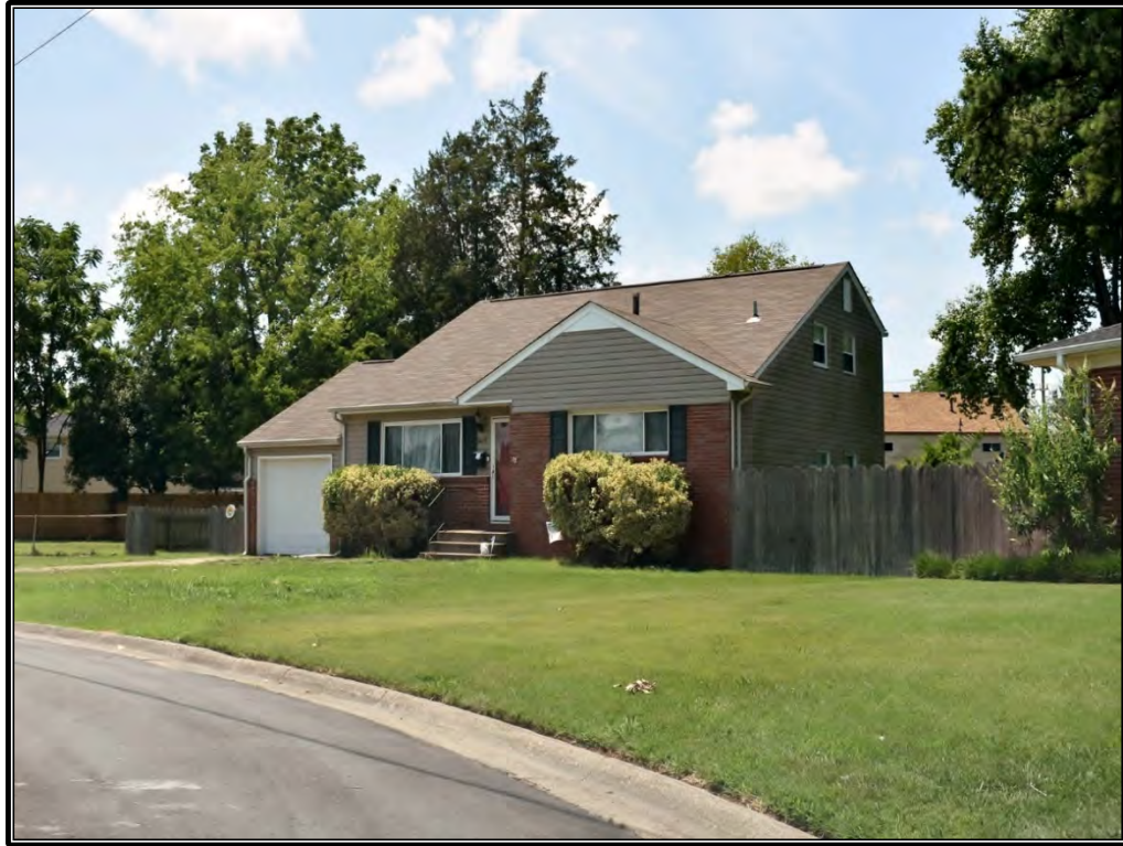
Figure 54. Minimal Traditional House (1963), 5829 S. Ottawa Road (134-5509)
