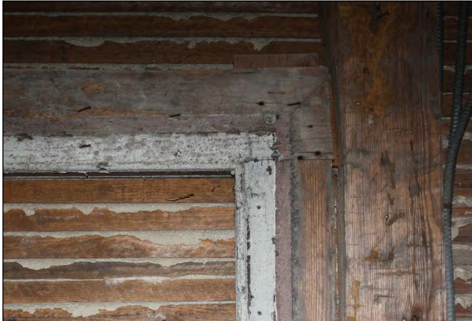
Figure 8-28. Detail of original pegged door frame.
