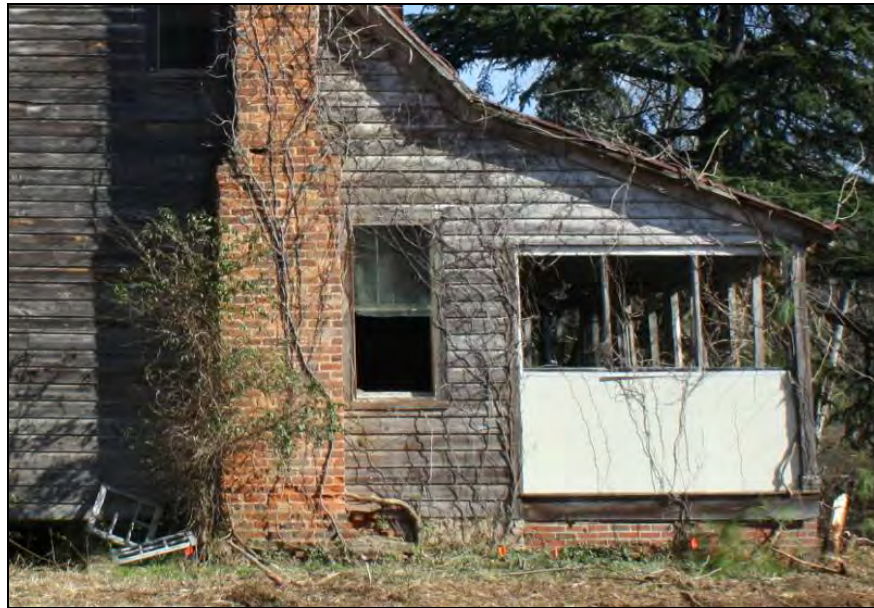
Figure 8-31. Window added to west side.
