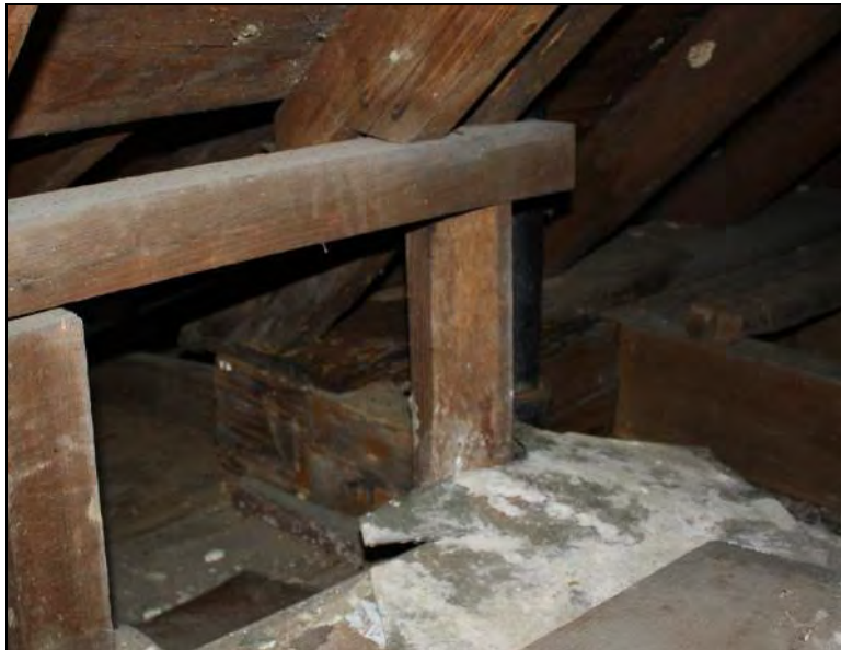
Figure 8-8. Plate and falseplate.
