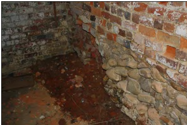
Figure 8-3. Cobbles in cellar wall
