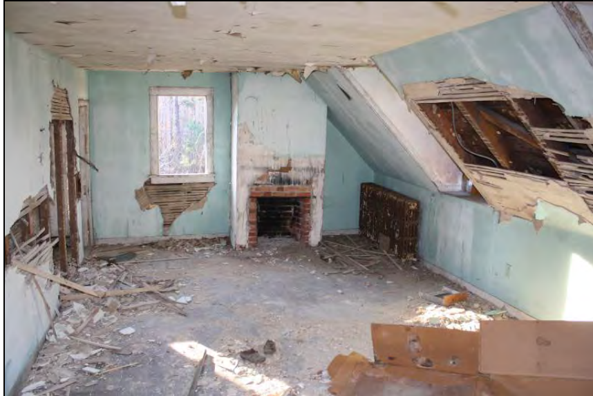
Figure 8-21. Northern bedroom with fireplace.
