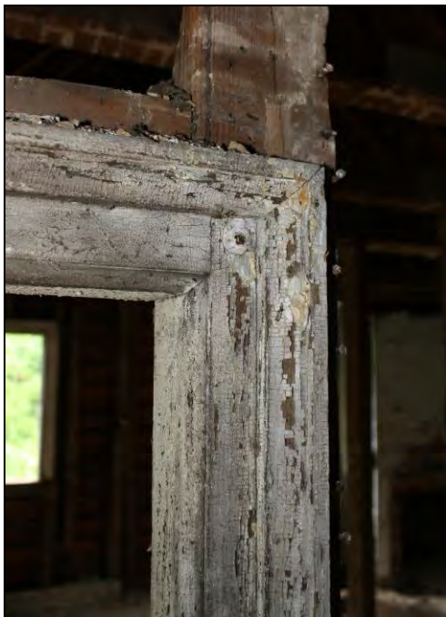
Figure 8-29. Greek Revival molding on original door frame.
