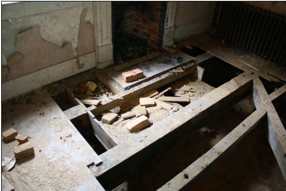
Figure 8-25. Hearth framing for first (Larger) and second (Smaller) southern end chimneys.
