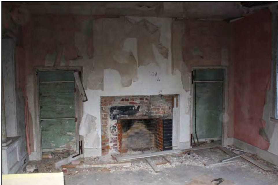
Figure 8-18. Fireplace in northern room with flanking closets.
