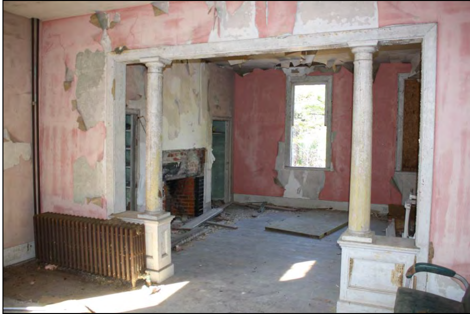
Figure 8-17. Partition wall with columns on knee walls.
