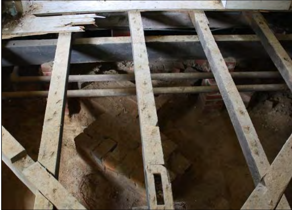
Figure 8-4. Original interior chimney base
