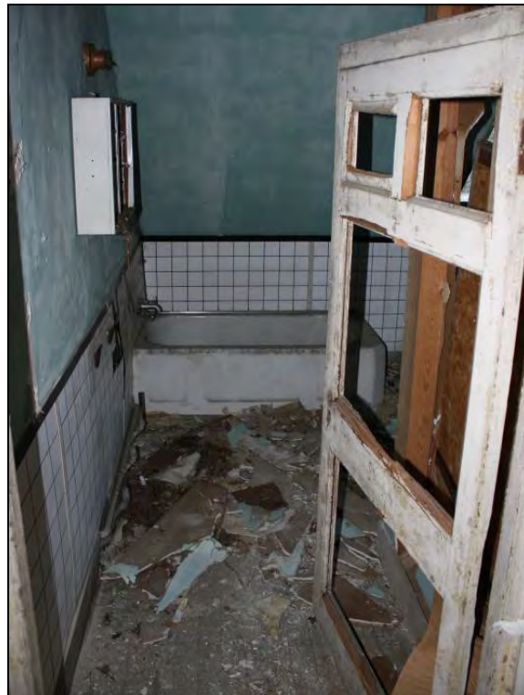
Figure 8-22. Bathroom in southeast room.
