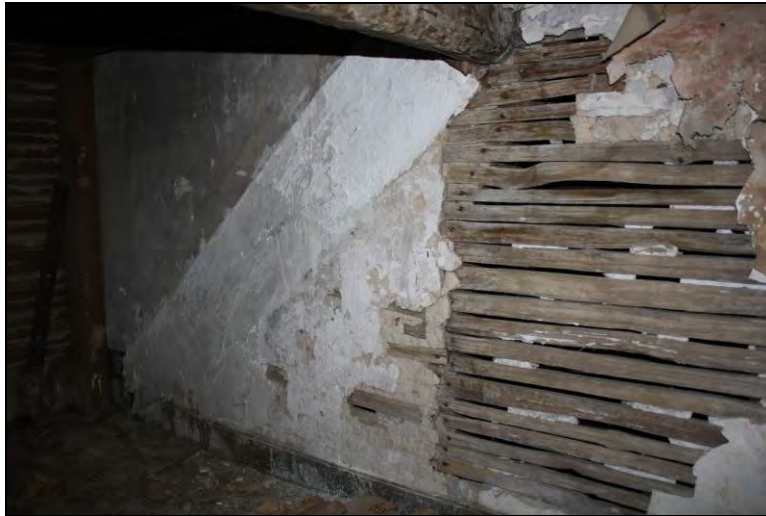
Figure 8-26. Original split pine lath under stair landing.
