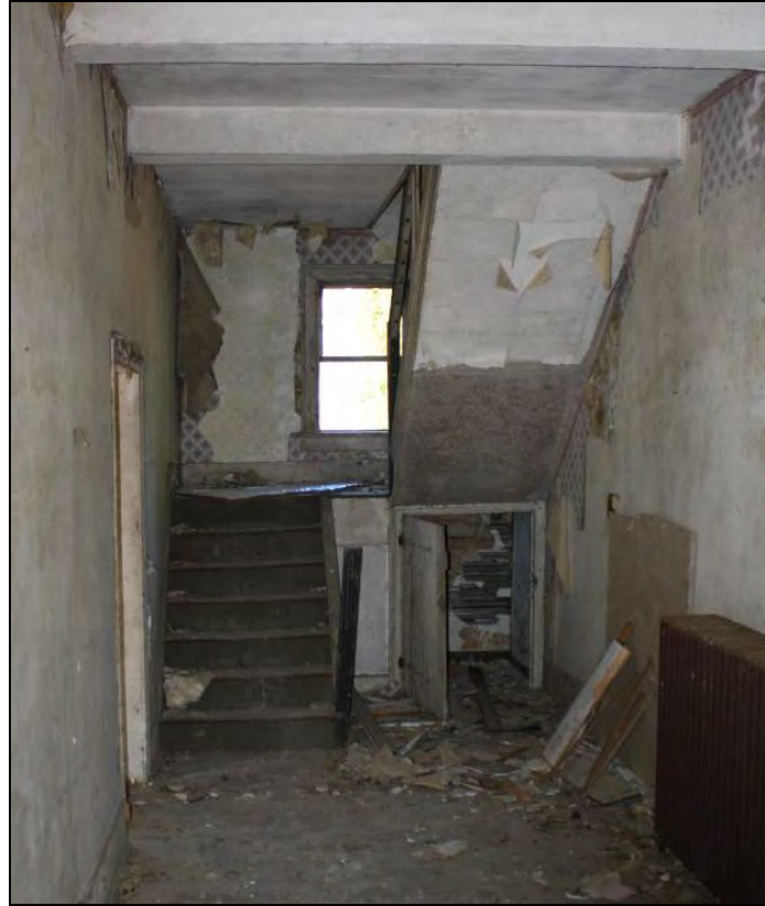
Figure 8-20. Stairway at end of side passage.
