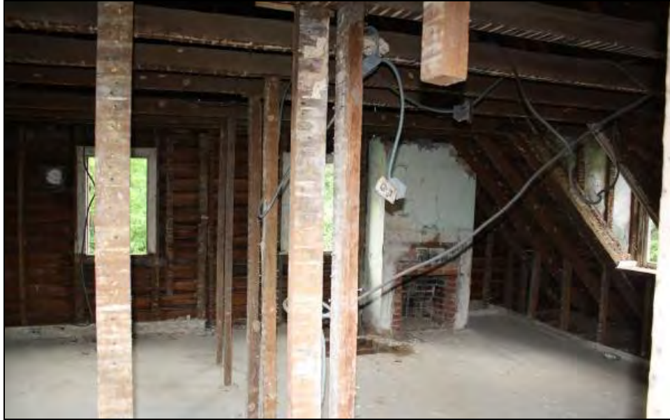
Figure 8-9. Second floor framing showing collars and knee walls.
