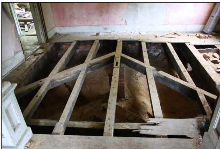
Figure 8-6. Dragon beams with later infill sub-joists.
