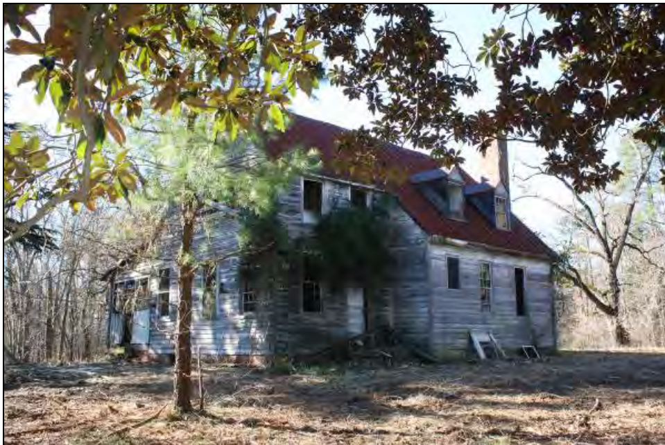
Figure 8-16. Fenestration on wing addition.
