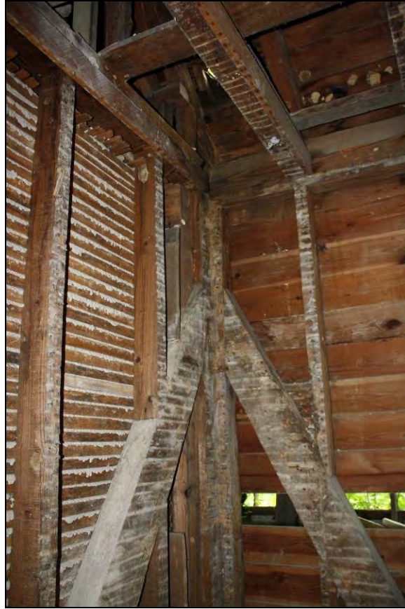
Figure 8-7. Guttered corner post and down braces.
