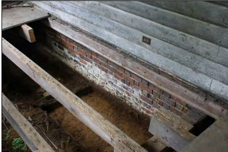
Figure 8-2. Original foundation laid in Flemish Bond
