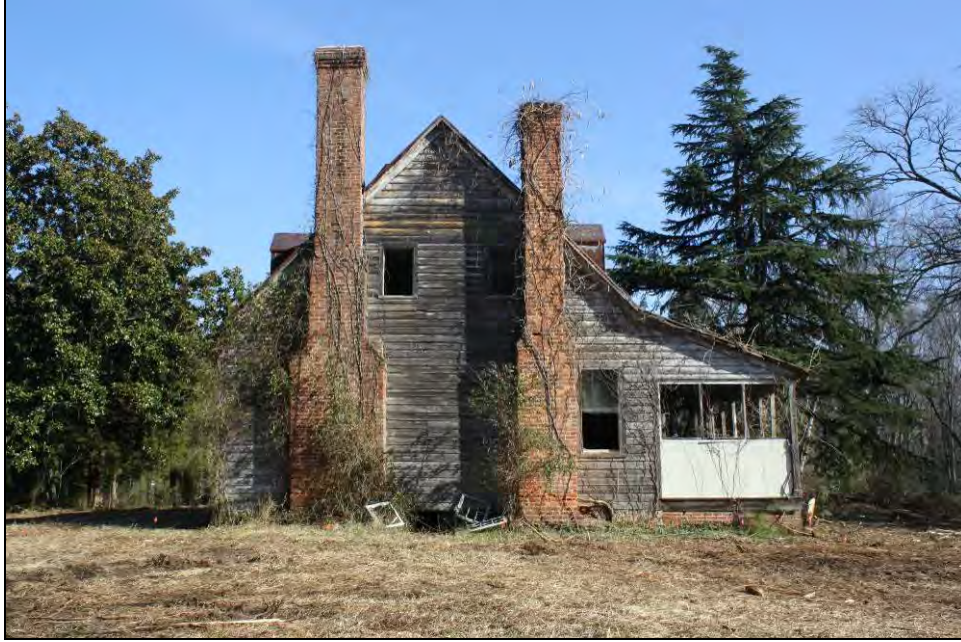
Figure 8-11. West side end chimneys.
