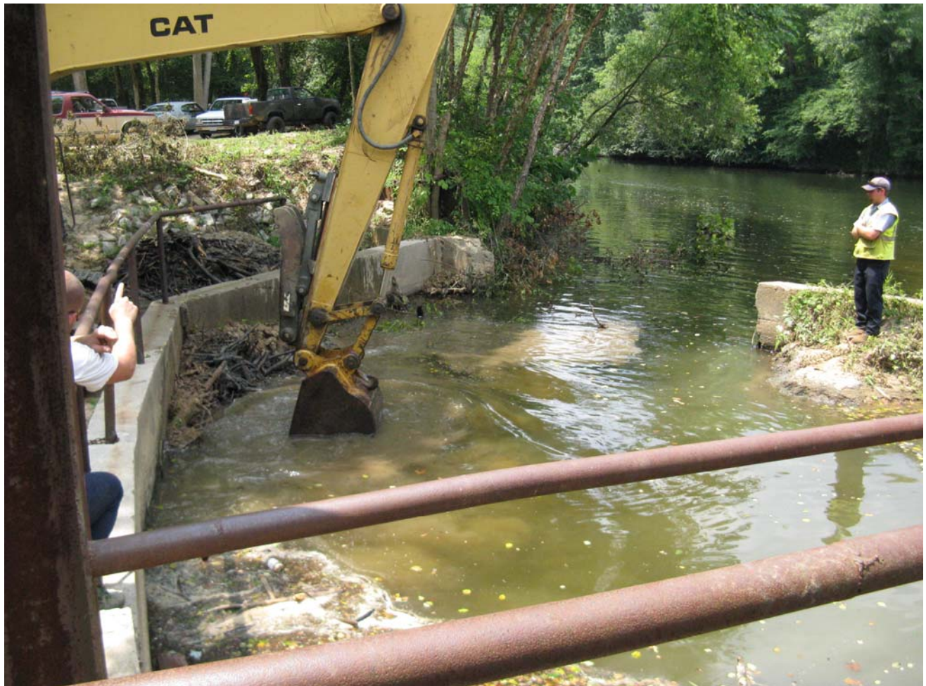
Debris Removal from Diversion Channel on Upriver Side of Dam in 2010
