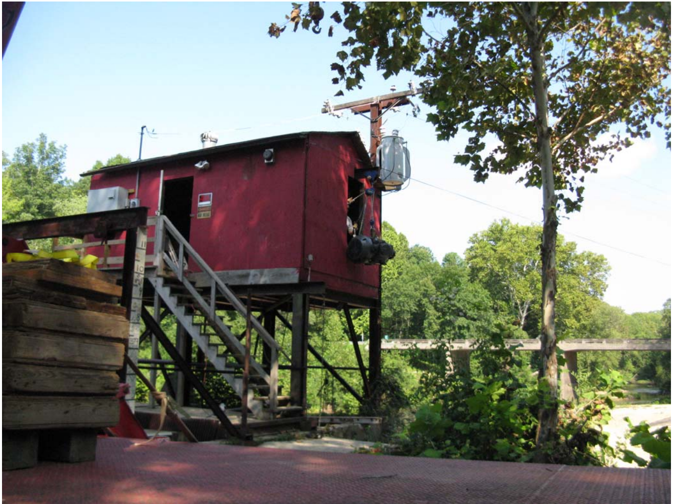
Generator being Hoisted into 1975 Powerhouse during 2010 Renovation
