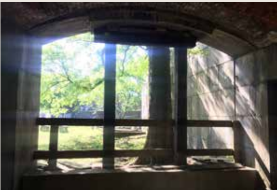
Timber bracing supporting the casement in silhouette.
