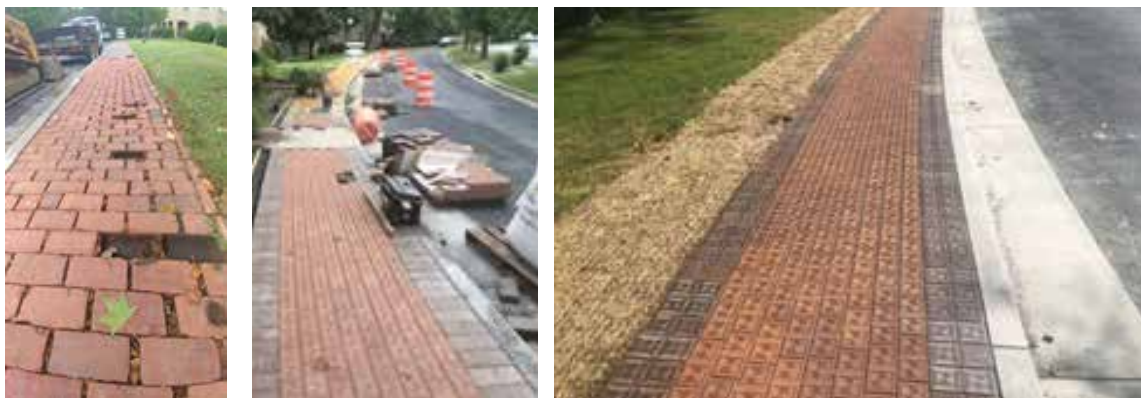
L-R: The brick walk at VMI prior to rehabilitation, during construction, and after completion.
