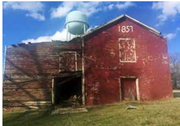
The Mule Barn at the former Powhatan Correctional Facility was demolished due to deterioration from neglect.
