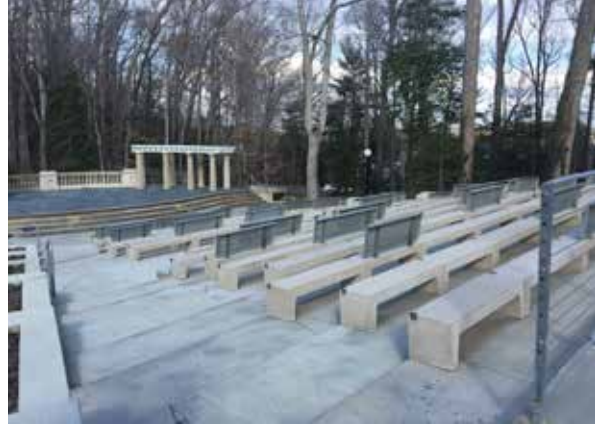
UMW's Amphitheater after restoration.
