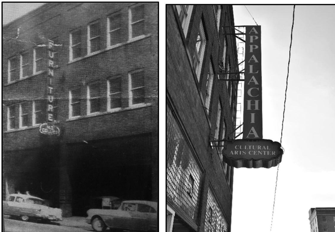
M.D. Collier Building, 320 W. Main Street. Left, original Collier sign (ca. 1950), Courtesy Appalachia Cultural Arts Center. Right, present sign on building.
