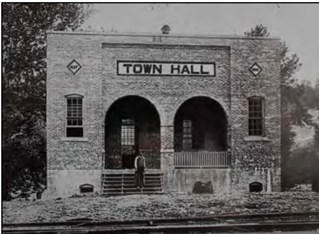
Former Appalachia Town Hall, 104 Powell Street, ca. 1920. Courtesy Lonesome Pine School and Heritage Center
