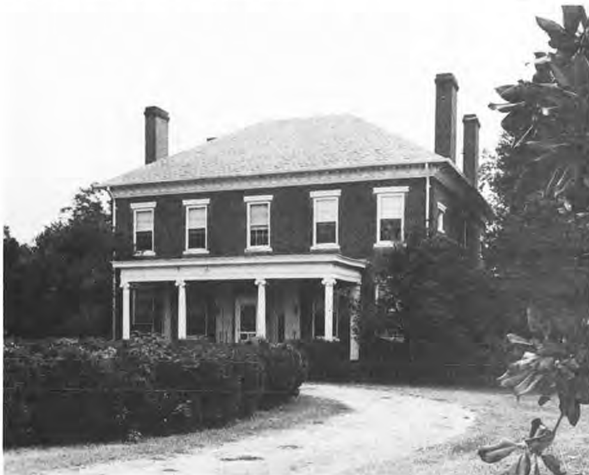
North (land) facade of mansion.
