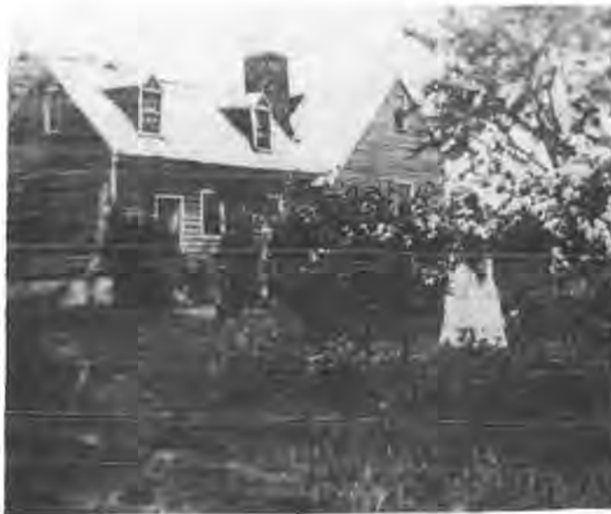
Ca. 1900 photograph: original side-hall plan house is on left.
