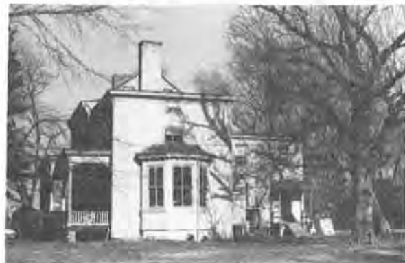
Top: west facade; north end. Bottom: original south wing; south end.
