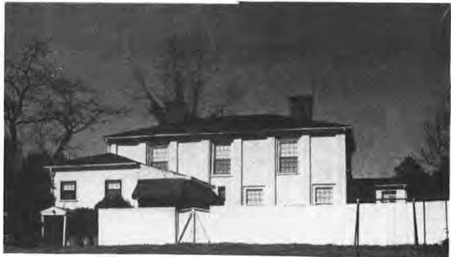
Page 132: north front. Above: east end. Right: south facade.
