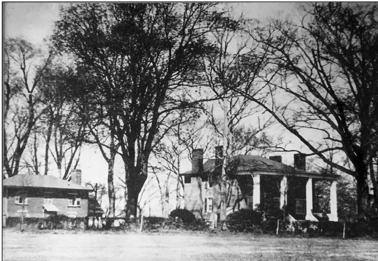
Figure 1. Early 20th century view of house and school, showing two-story porch on house, since replaced with a one-bay portico.
