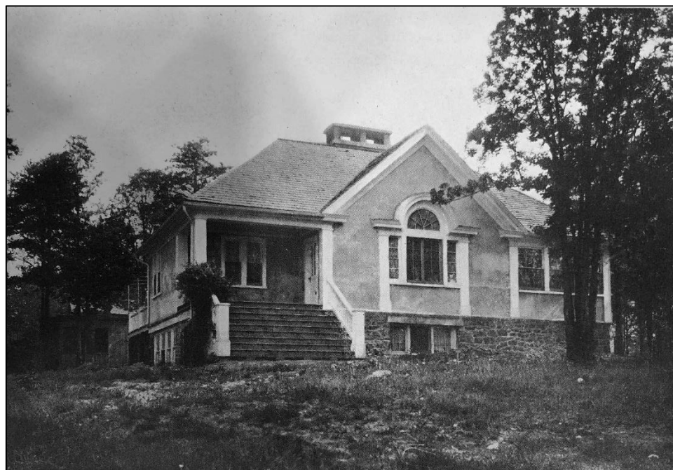
Figure 11. The original WCS building.
