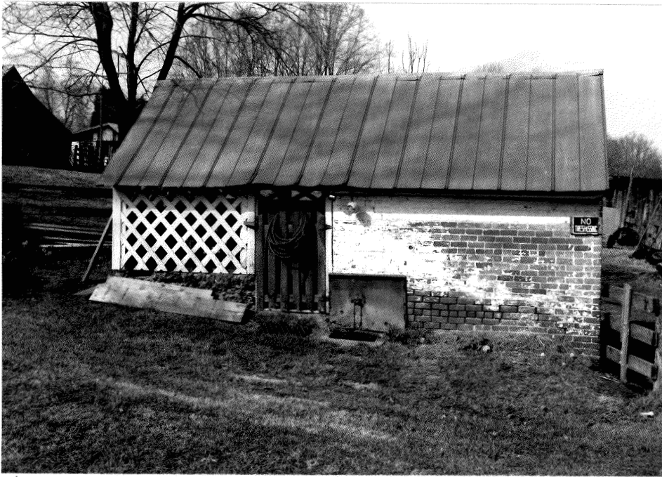
Figure 38: Photograph of Springhouse at Walnut Hill Farm, (89-196), (Tracerics, 1992)
