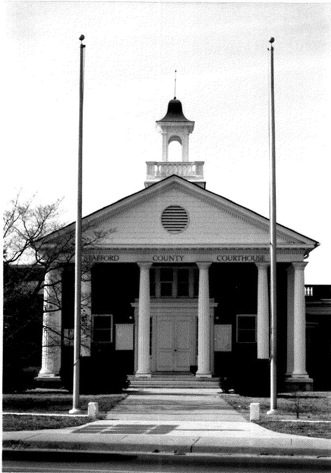
Figure 50: Photograph of Stafford County Courthouse (89-15), (Tracerics, 1992)
