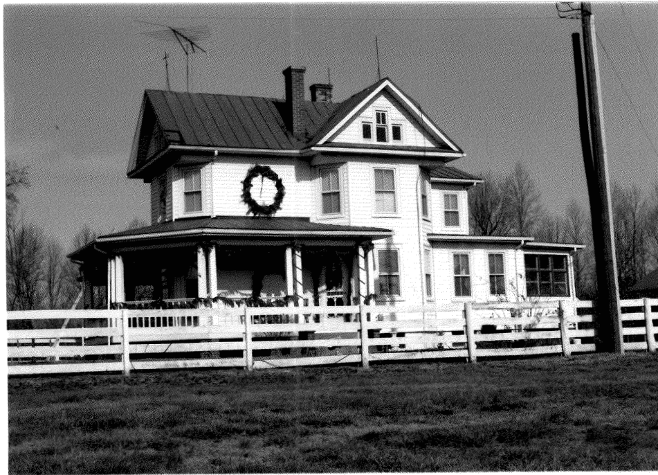
Figure 22: Photograph of House, Hartwood Road (89-127), (Tracerics, 1992)
