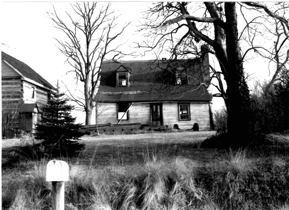
Figure 7: Photograph of Concord (89-97), (Traceries, 1991)
