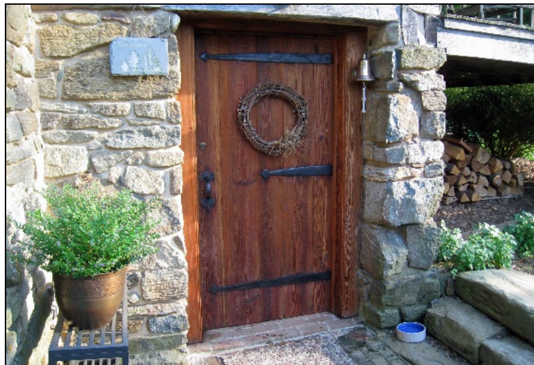
Figure 2. Basement-level entrance door on south elevation
