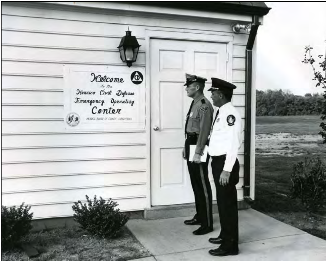
Henrico County Photographs of construction and entrance of Emergency Operating Center 1965.
