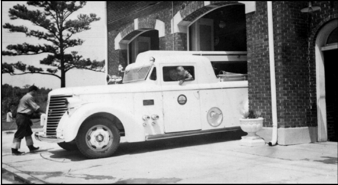
Figure 2: Fire Station No. 12, ca. 1943. Image shows difficulty maneuvering fire engine through narrow doors.
