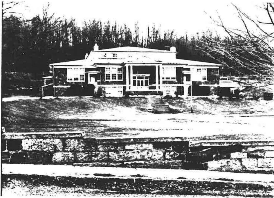
24: Highland County Courthouse, 262-0002. North elevation.
