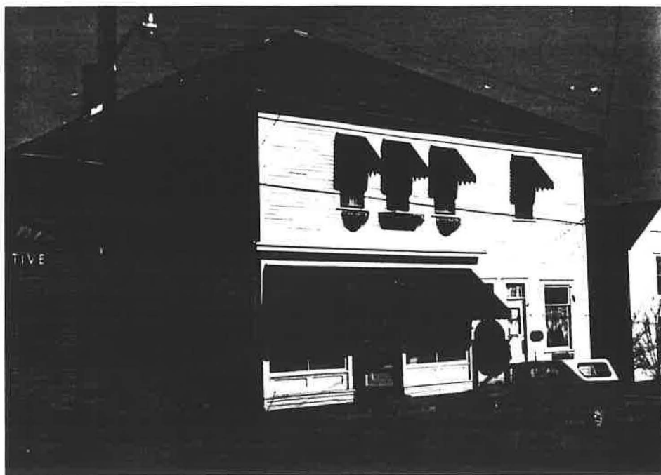
12: Lunsford and Sons Store, 262-0054. South elevation.
