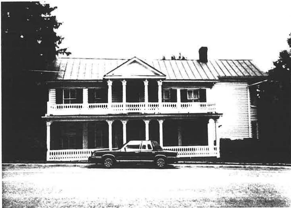
Plate 4: Almond-Strickler House, 262-0001. South elevation.
