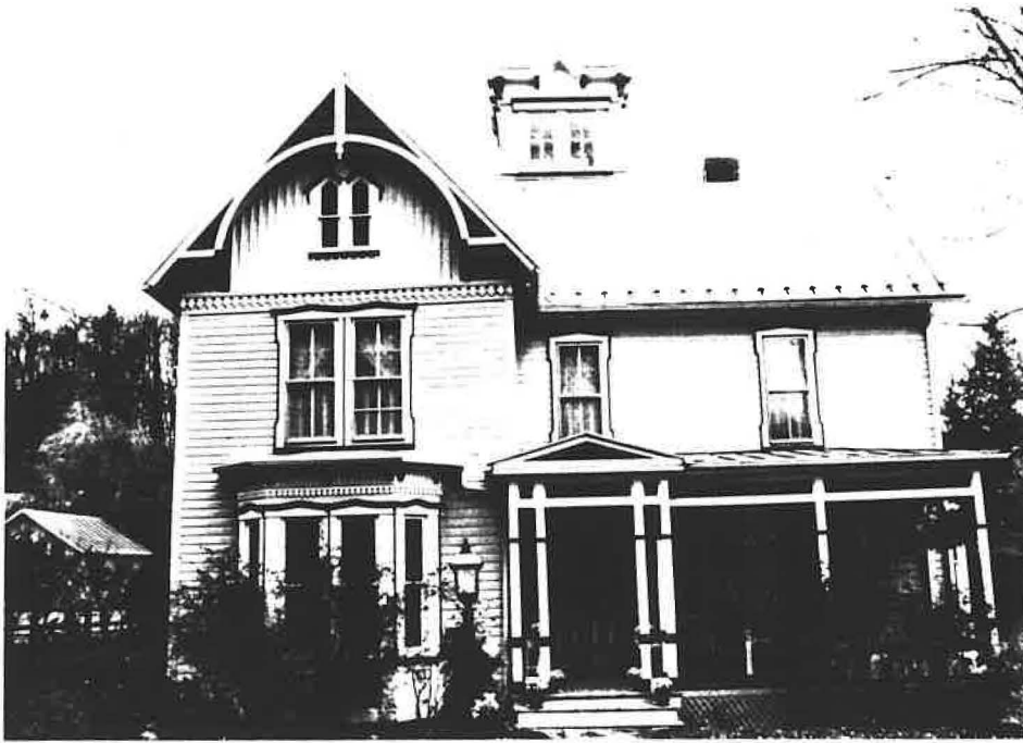
Plate 6: Lucius H. Stephenson House, 262-0011. East elevation.
