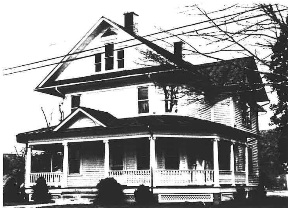
Plate 19: J. Brown Lightner House, 262-0024. West elevation.
