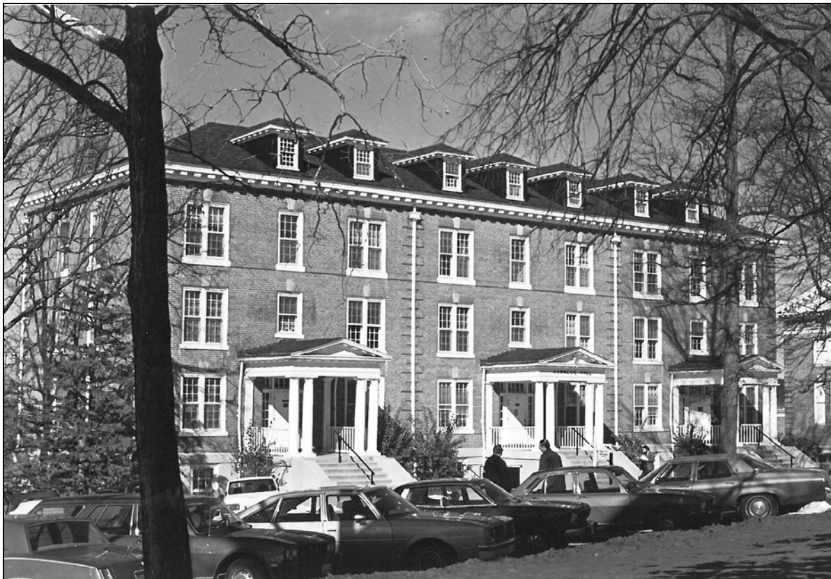
Figure 3. Carnegie Hall in 1980 (Image courtesy of the Virginia Department of Historic Resources)
