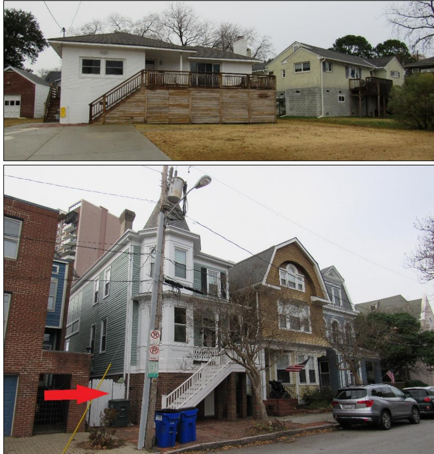
Photo 2: Elevated Houses at 1210 and 1216 Richmond Crescent of Larchmont, Looking North (Top); Elevated House at 723 Yarmouth Street (New Raised Foundation Denoted by Red Arrow) in Relation to Surrounding Buildings, Looking West (Bottom).
