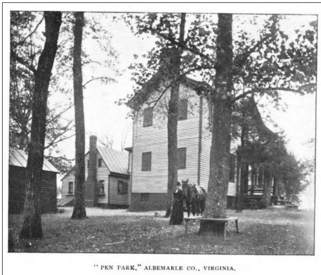
Figure #3: Pen Park residence, taken in the late nineteenth century. Note the 'H-shape' to the residence with the smaller older structure (at left) located behind the newer younger structure (at right) and hyphen connecting them.
