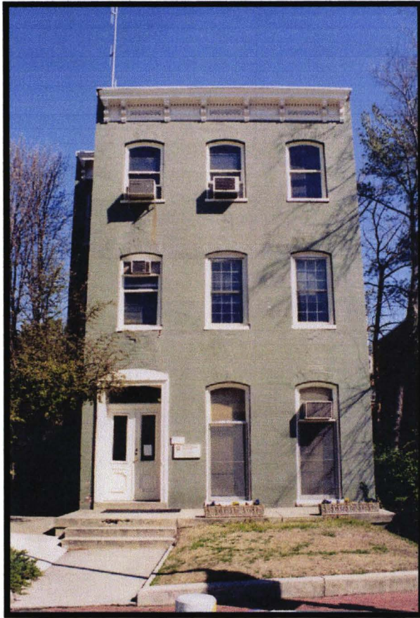
Plate 4. Adkins House facade, view to the northeast.
