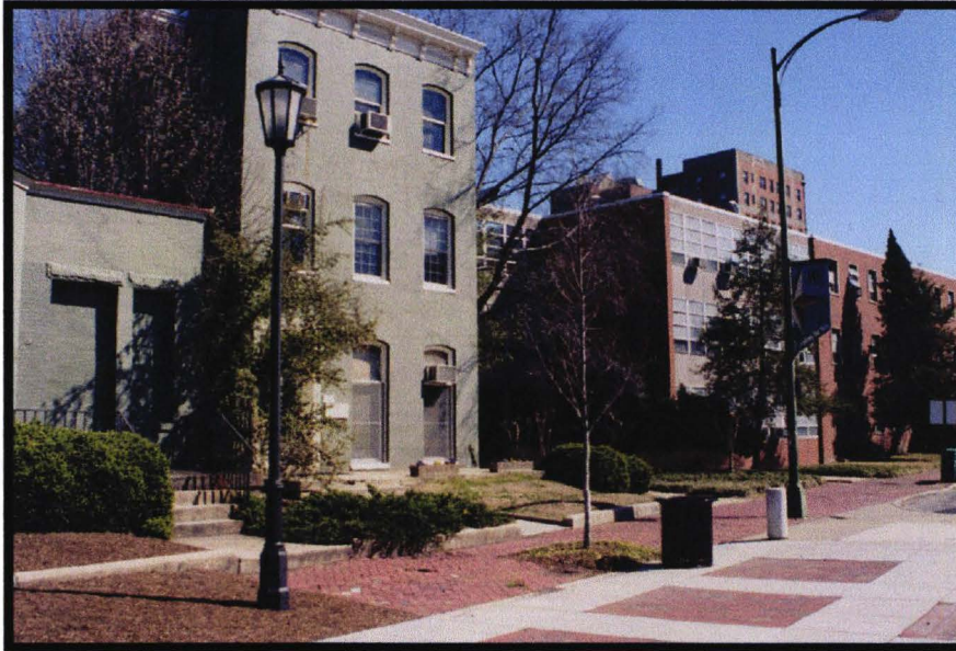
Plate 2. View of Adkins House and adjacent Life Sciences Building, view to the east.
