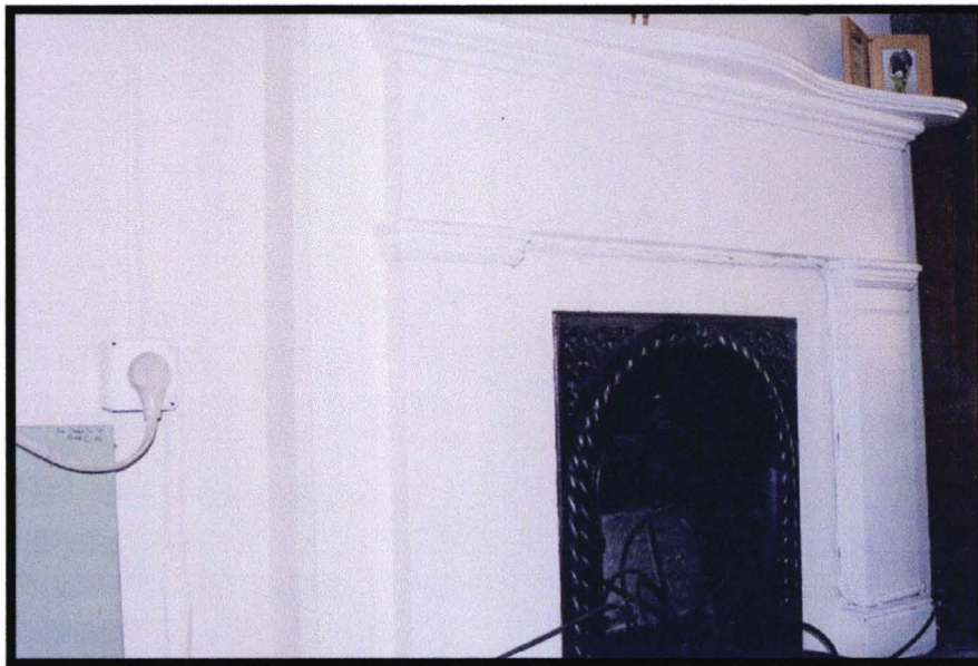
Plate 7. Adkins House, second floor mantel.
