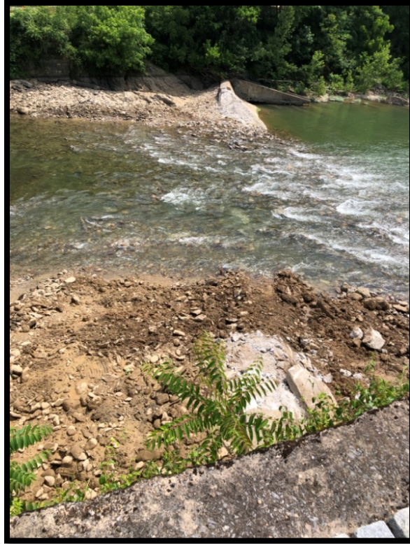
Figure 34: View from south abutment after completion of dam demolition (May 30, 2019).
