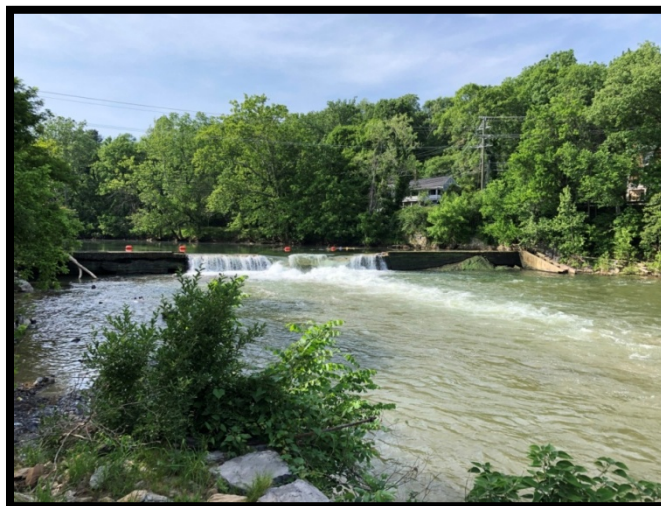
Figure 15: End of day on May 23, 2019, showing breached dam.
