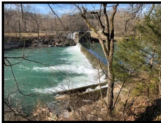
Figure 20: View fish ladder taken from downstream, north bank. (February 2019).
