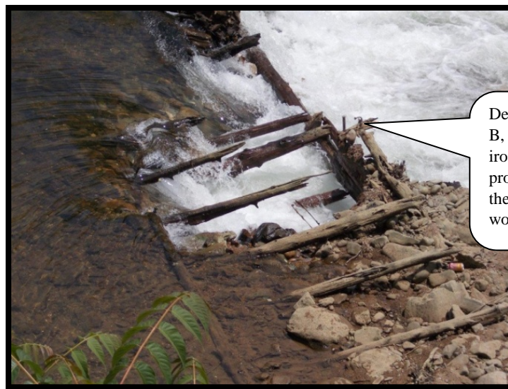
Figure 29: Remnant of Section B removed near the south end of the crib dam (May 24).
