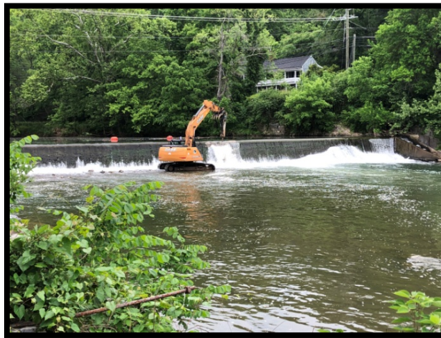
Figure 14: Beginning of removal, view from downstream (May 23).
