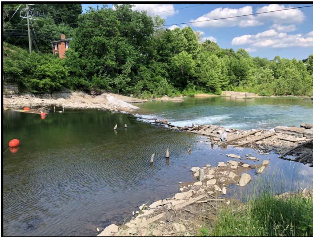
Figure 19: May 28 view from south bank, upstream of dam. By that time, water had continued to drop and more remnants of the crib dam were exposed. Some of these included vertical pinning posts for the crib dam and the structural remnant near the south bank. The vertical posts were removed as part of the crib dam removal.
