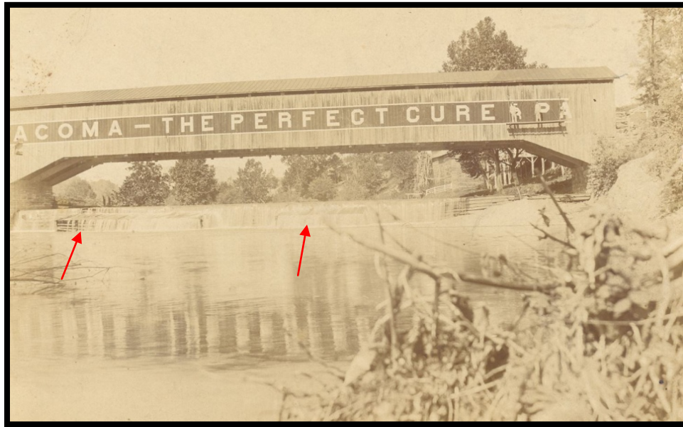
Figure 11: Ca. 1900 photo of the covered bridge and crib dam at Jordan’s Point. The applied arrows show the sloped buttresses covered in wooden planks that helped to strengthen the dam (W&L University Leyburn Library Special Collections).
