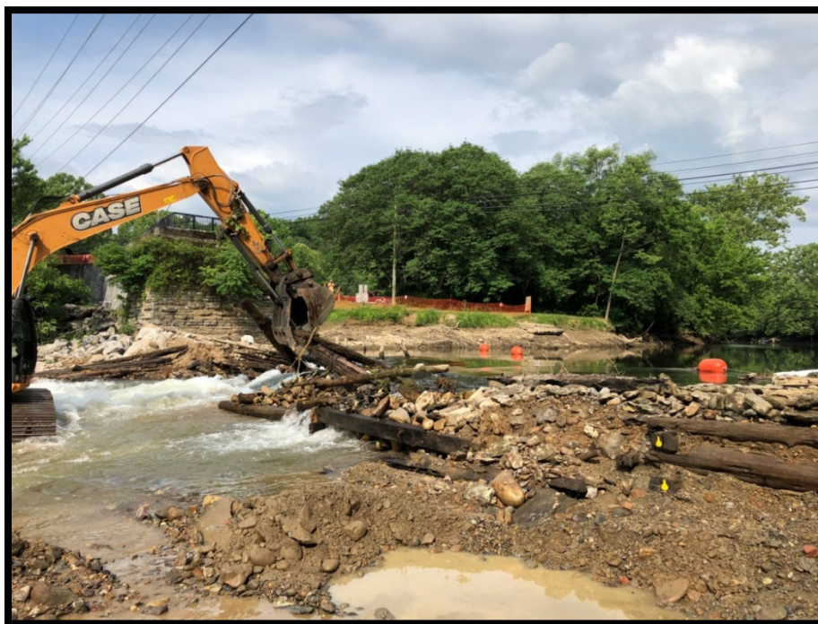
Figure 31: Removal of Sections B and C of the crib dam (May 29, 2019).
