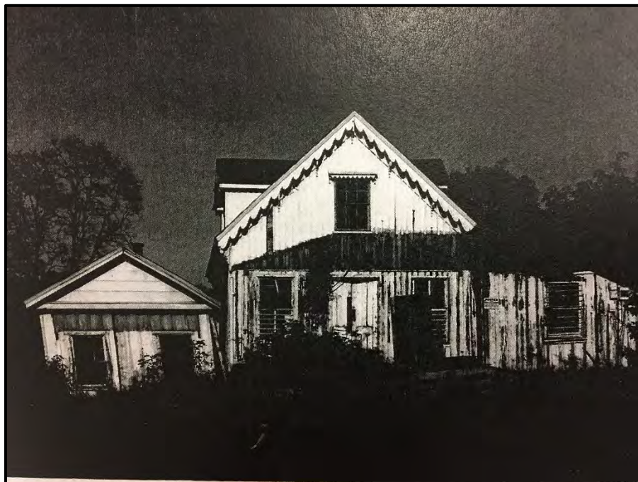
Figure 4. Howardsville Store and Post Office (VDHR #002-0207/#002-5045-0482) (Photograph taken by Ed Chappell).
