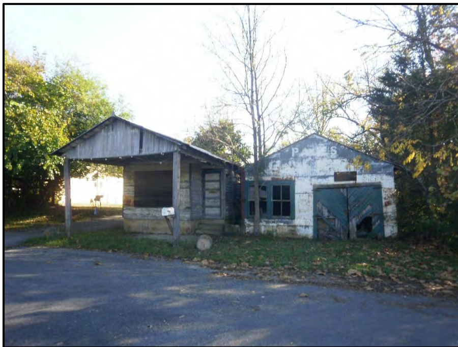
Figure 20. Pace's Store/Esmont Gas Station (VDHR #002-0433/002-5045-1125), 3127 Paces Store Road.
