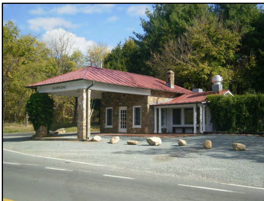
Figure 22. Colle Service Station (VDHR #002-0834/002-5045-0218), 1330 Thomas Jefferson Parkway.
