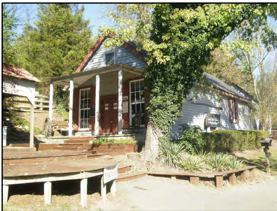
Figure 5. Hatton Store (VDHR #002-0773/#002-5045-1431), 10092 Hatton Ferry Road.
