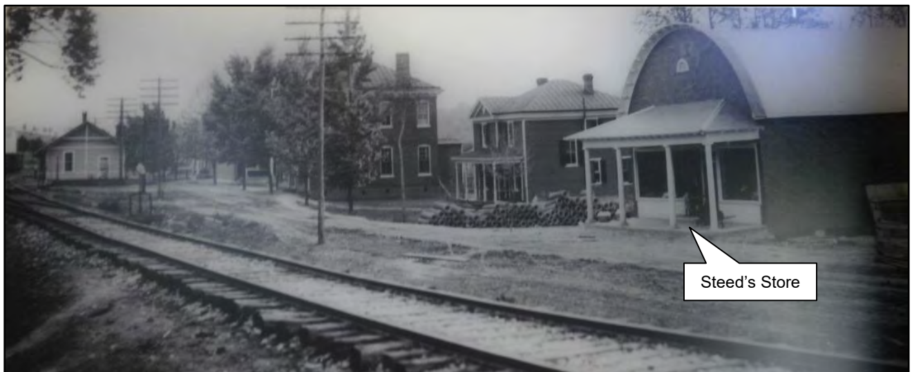
Figure 14. View of Esmont Depicting Steed's Store (Far Right; Photographer Unknown; Photograph located at the Esmont Post Office).
