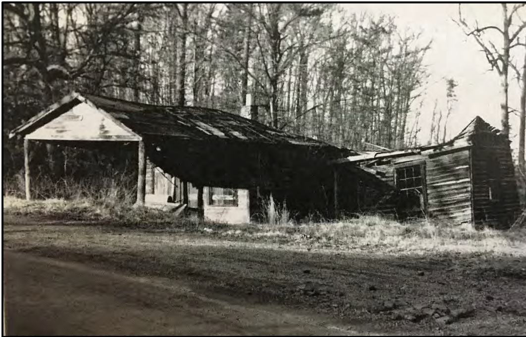
Figure 23. Charles Thompson Store (VDHR #002/0858/#002-5045-0431), 2941 Rolling Road (Photograph taken by Jeffrey O'Dell).
