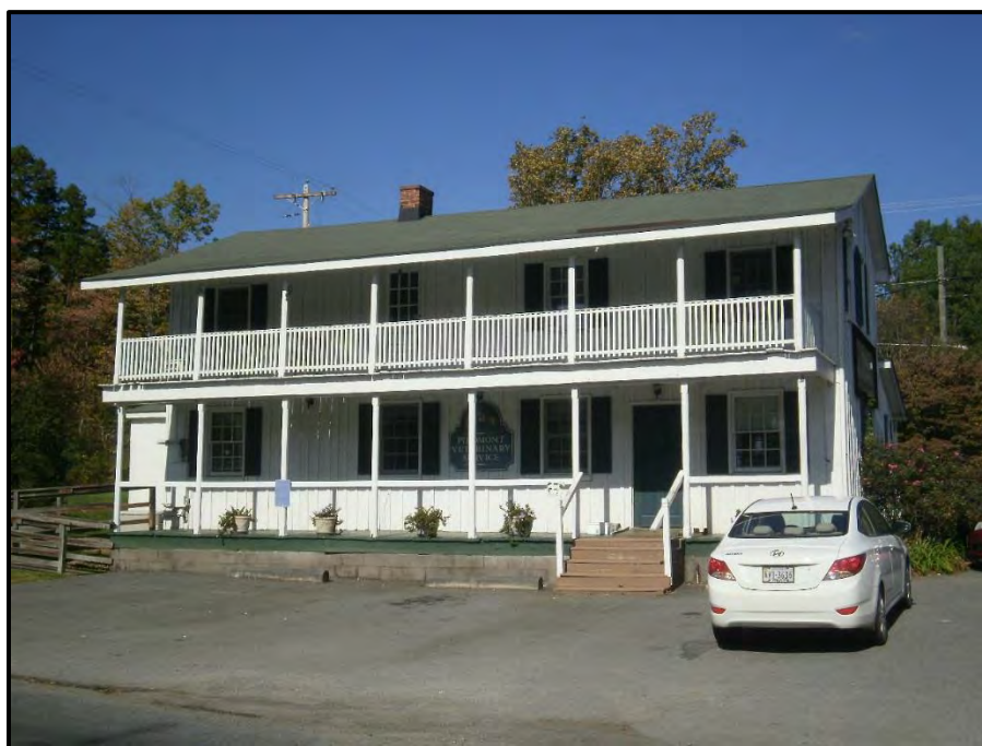
Figure 10. Store (VDHR #002-0414/002-5045-0186), 1418 Plank Road.
