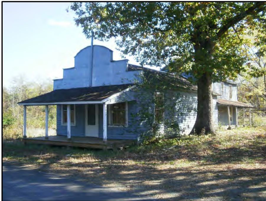
Figure 15. Old Dominion Store (VDHR #002-5045-0900), 5053 Green Creek Road.
