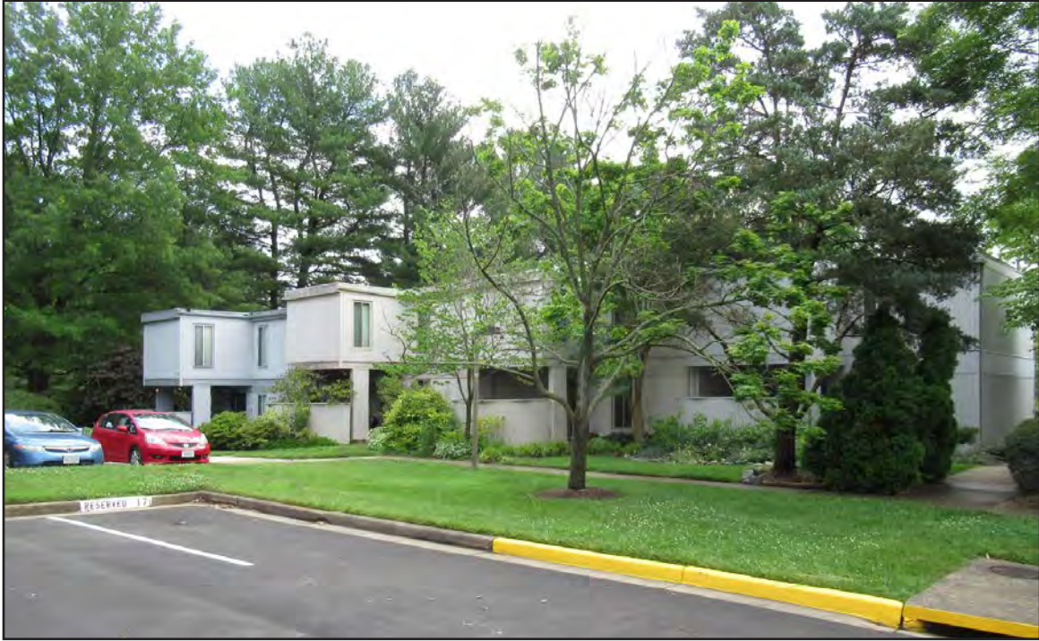
Figure 73. Fairway Cluster (029-6774), Units 1801–1807, looking east.
