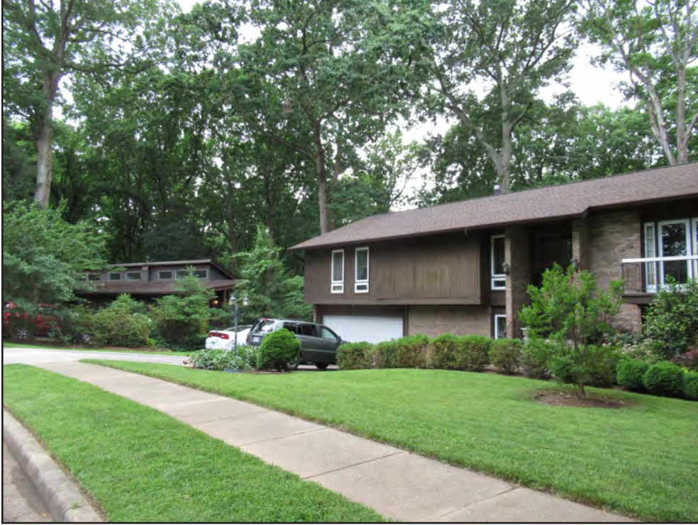
Figure 63. Ring Road Subdivisions (029-6780), looking southeast.
