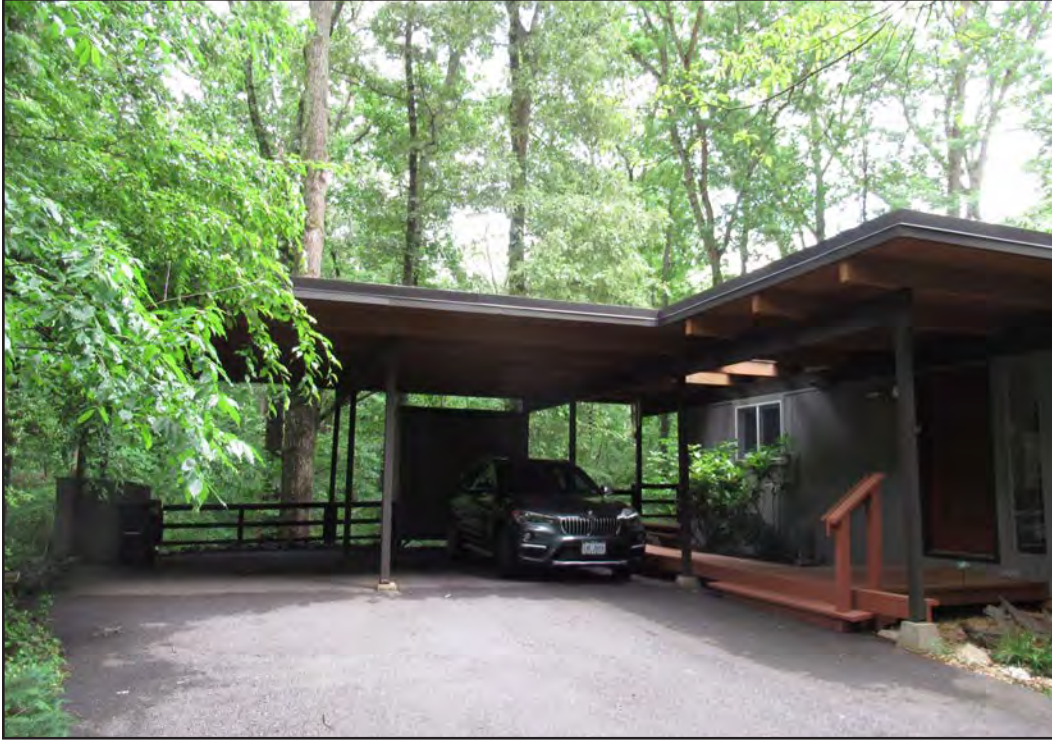
Figure 67. House, 12146 Stirrup Road (029-6755), carport and entrance.
