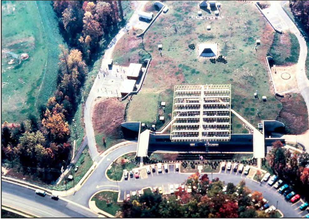
Figure 43. Aerial view of Terraset Elementary School (029-6647) after completion in 1977, showing original turf-covered roof
