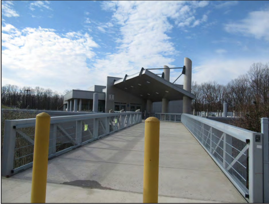
Figure 47. Terraset Elementary School (029-6647), bridge leading to entrance.
