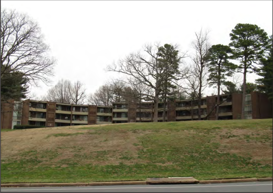
Figure 64. Cameron Crescent Apartments (029-6650), southeast building, looking north.
