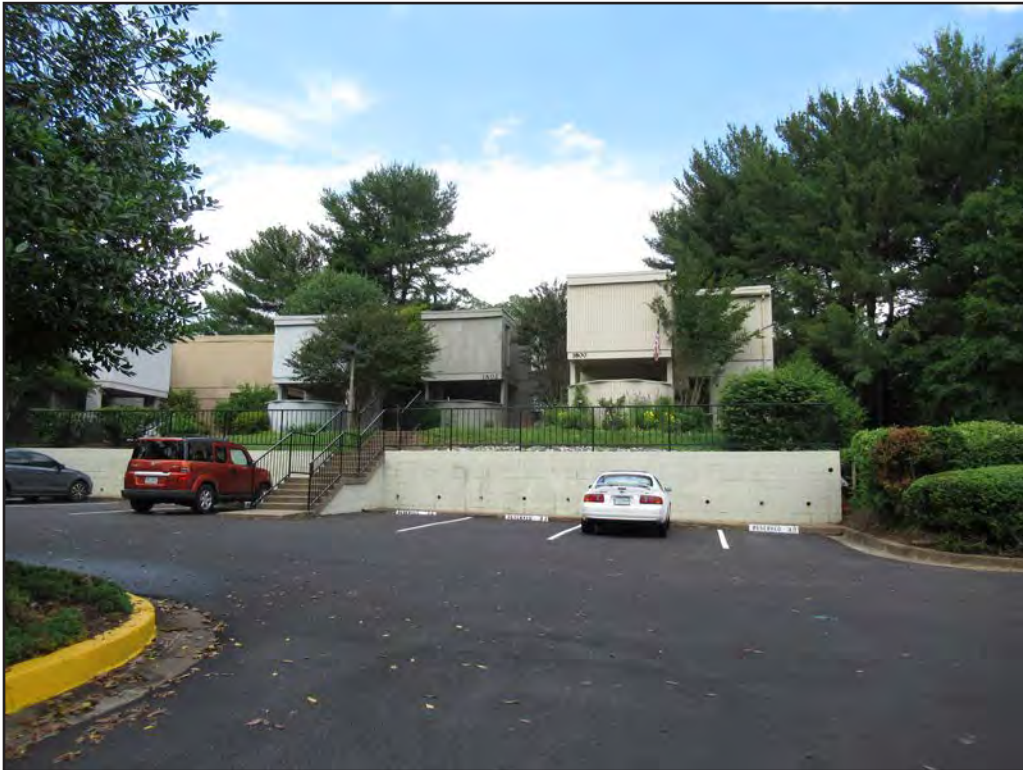
Figure 74. Fairway Cluster (029-6774), Units 1800–1804, looking northwest.
