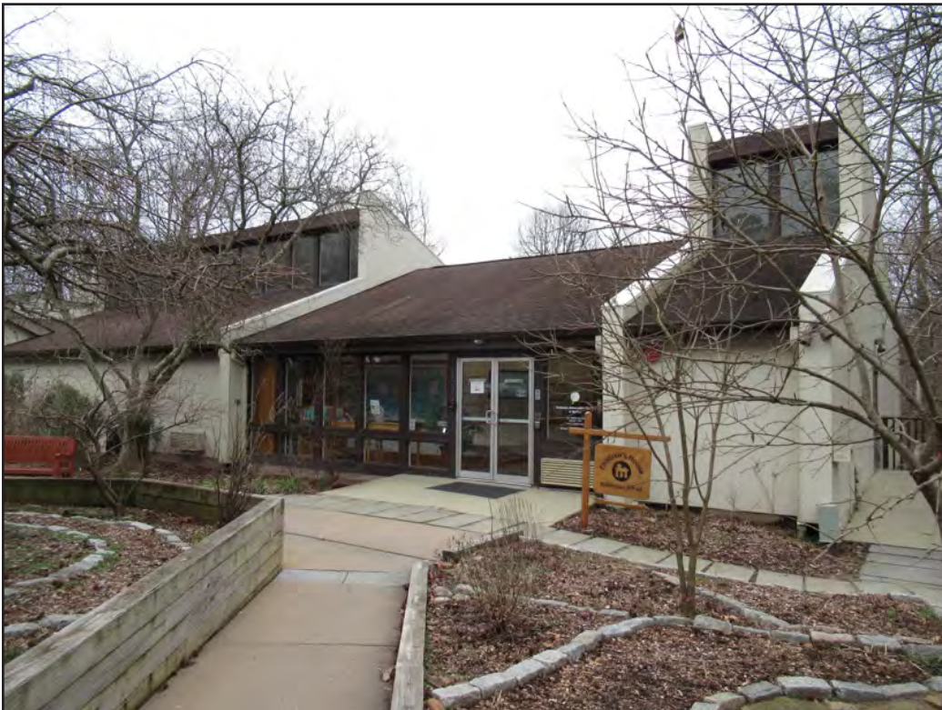
Figure 49. Wiehle Avenue Unitarian Universalist Church (029-6651), west end of facade.
