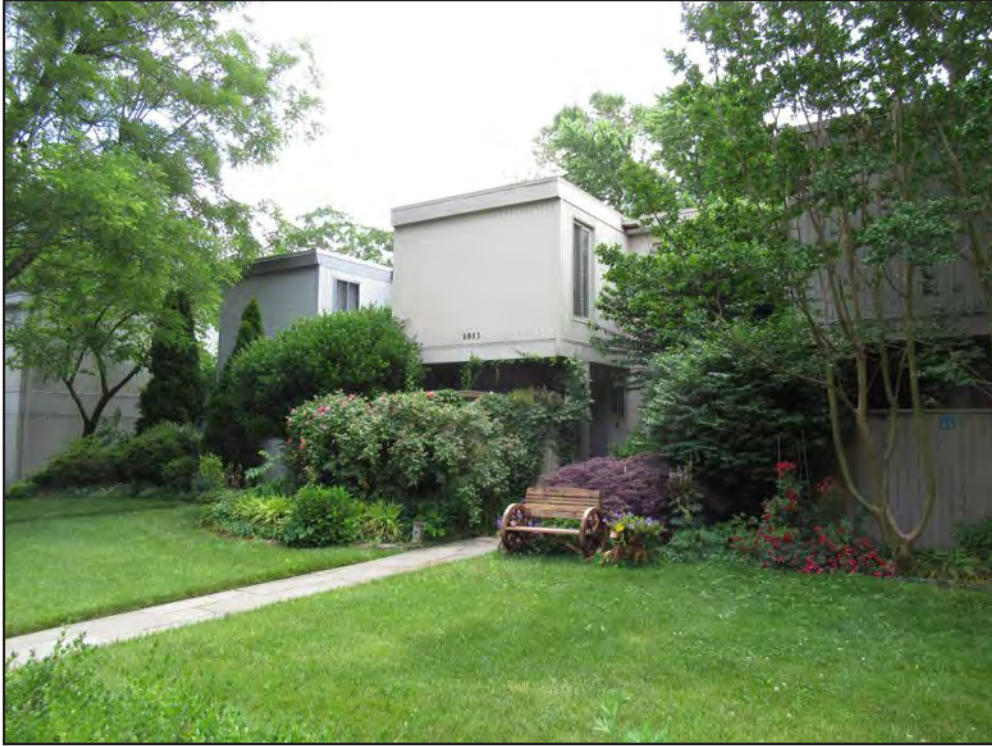
Figure 75. Fairway Cluster (029-6774), Units 1809–1813, looking east.
