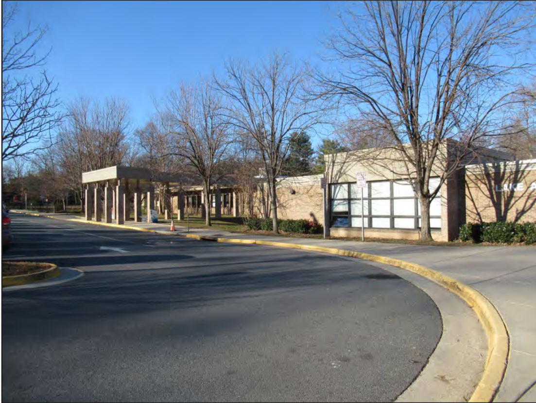
Figure 30. Lake Anne Elementary School (029-6642), northeast elevation (facade).
