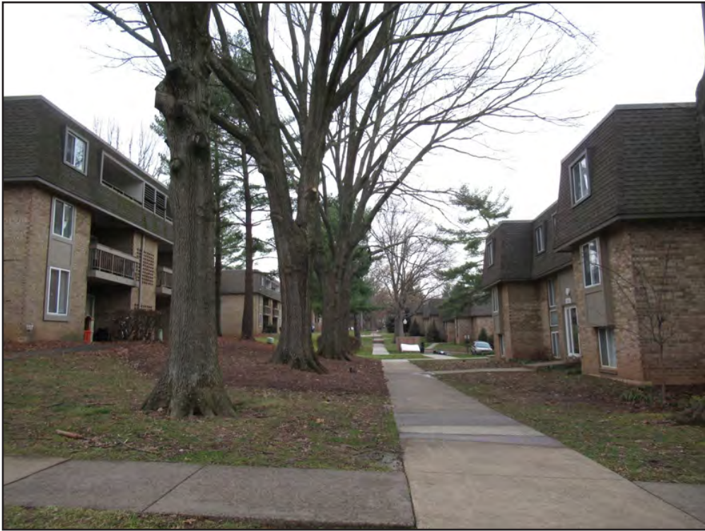
Figure 59. Fairway Apartments (029-6652), West Center Court, looking west.
