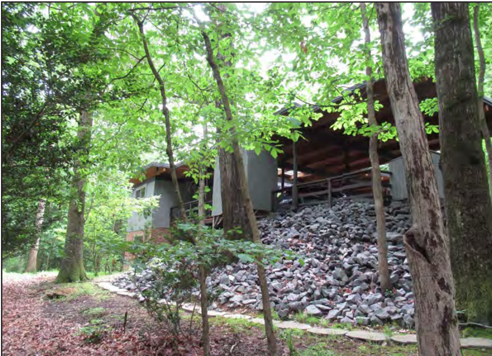
Figure 68. House, 12146 Stirrup Road (029-6755), northeast corner.
