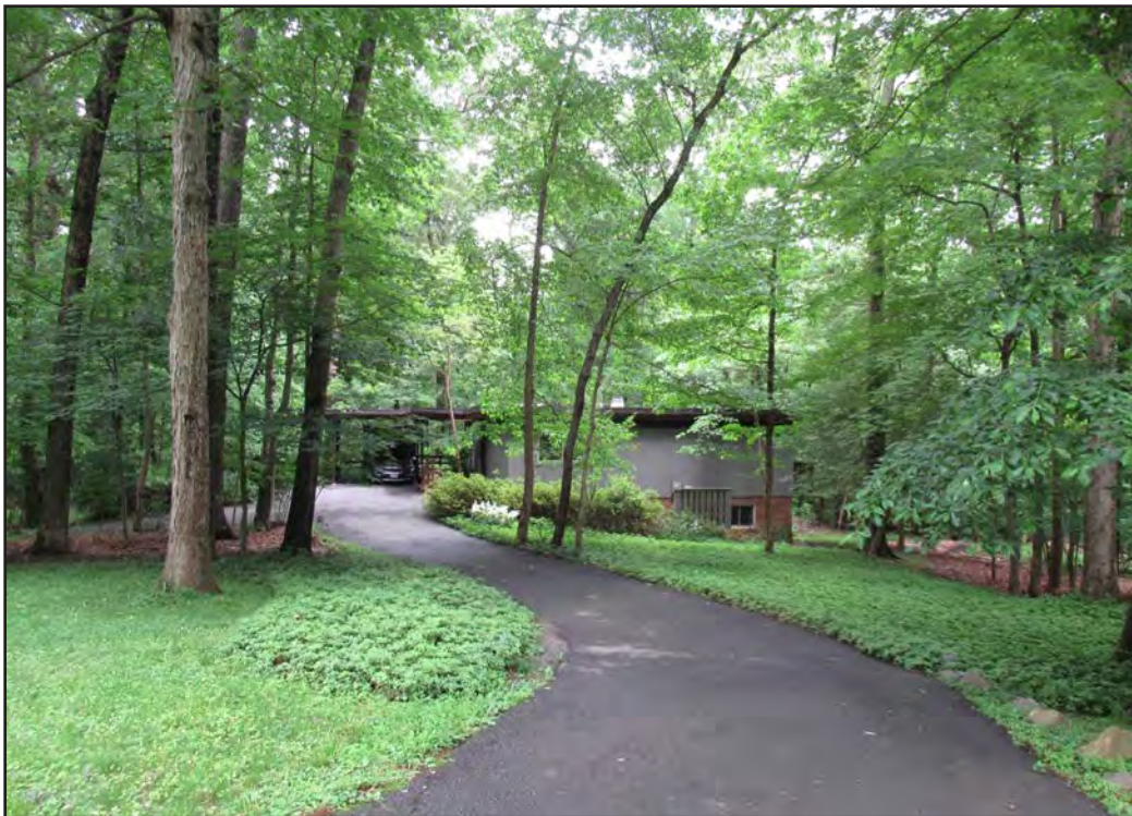
Figure 66. House, 12146 Stirrup Road (029-6755), driveway and west elevation.
