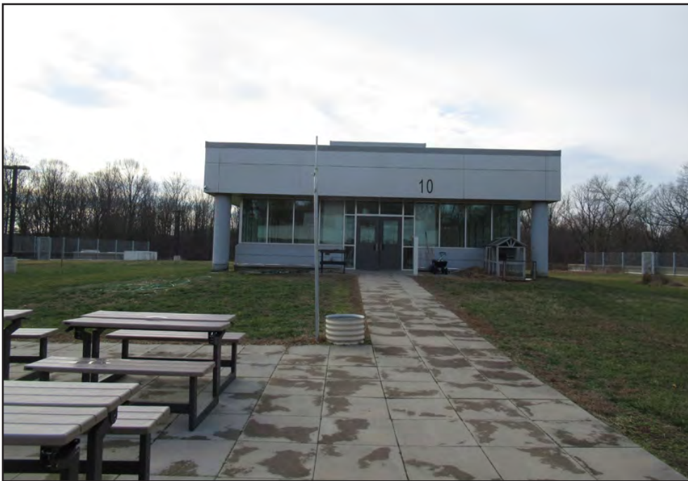
Figure 46. Terraset Elementary School (029-6647), roof, looking south.
