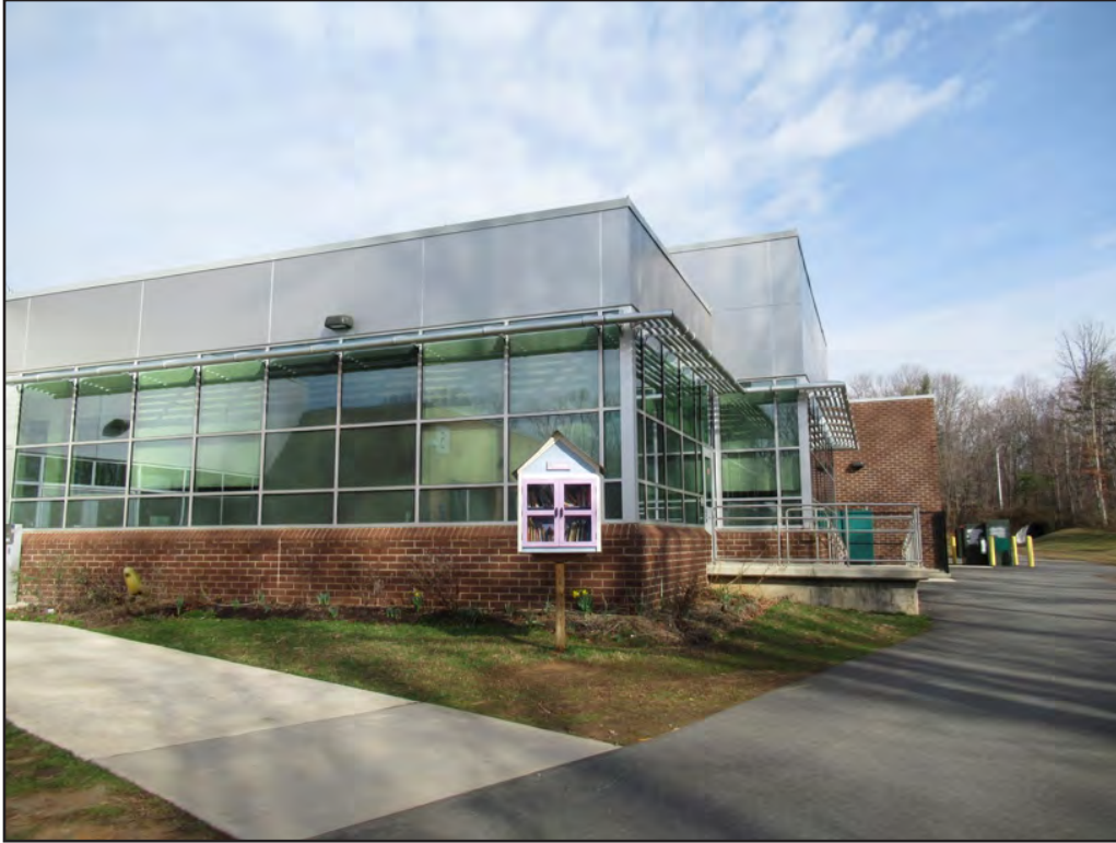
Figure 45. Terraset Elementary School (029-6647), east elevation, looking north.
