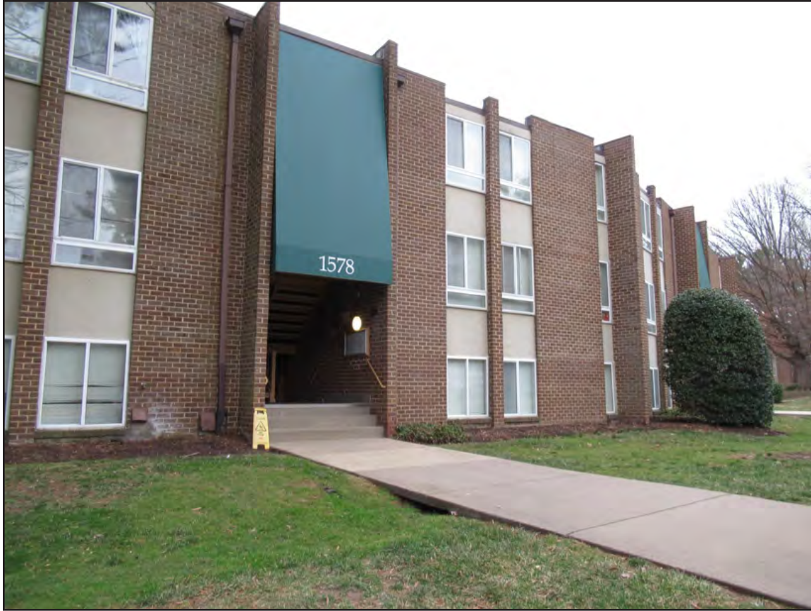
Figure 65. Cameron Crescent Apartments (029-6650), southwest building, southeast entrance.
