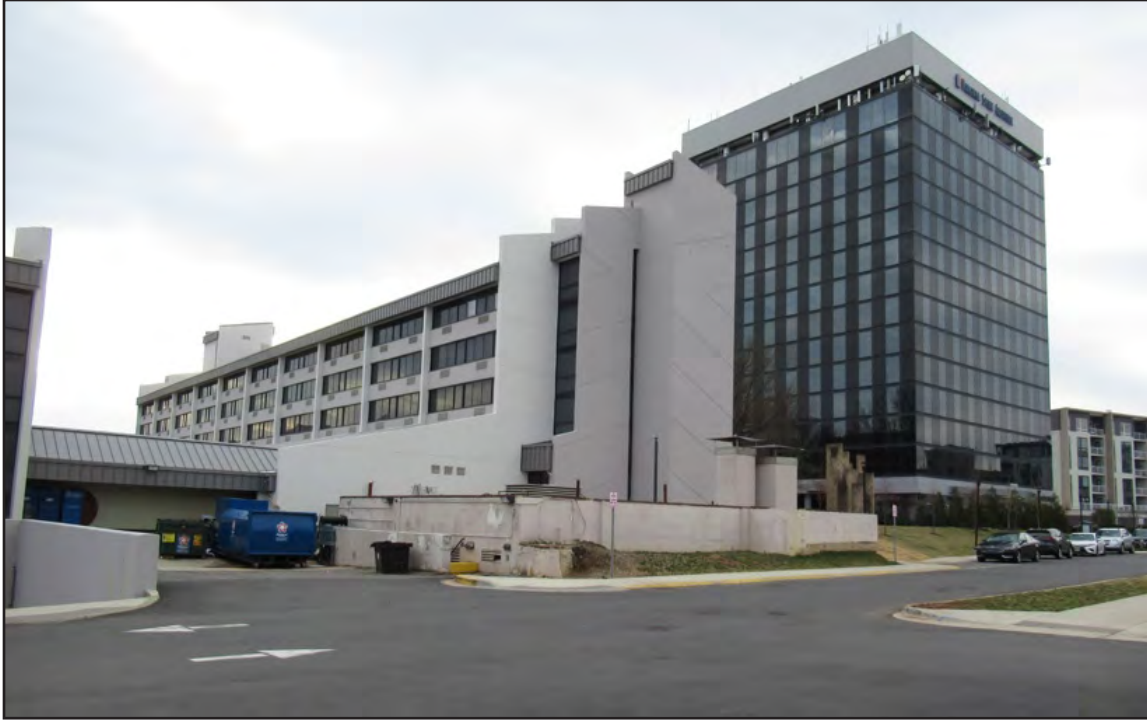
Figure 38. Sheraton Reston Hotel (029-6646), southwest corner.
