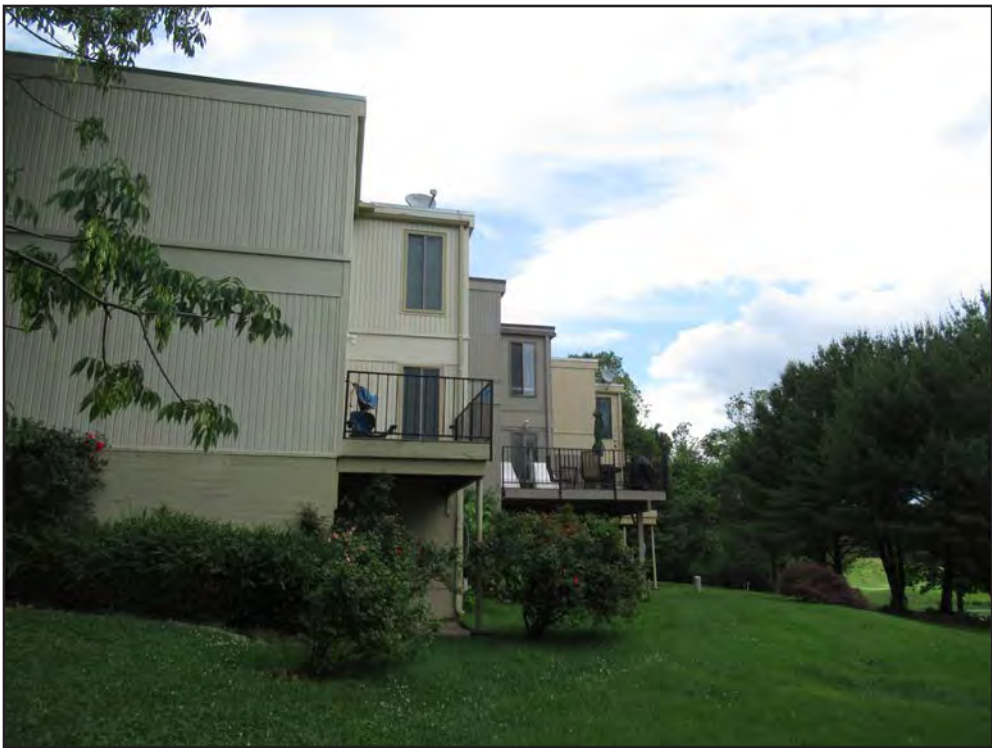
Figure 76. Fairway Cluster (029-6774), Units 1819–1823, looking east.
