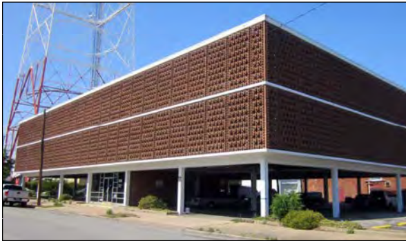
Tower Building, City of Richmond DHR File No. 127-6136-0004 VLR, NRHP 2017
