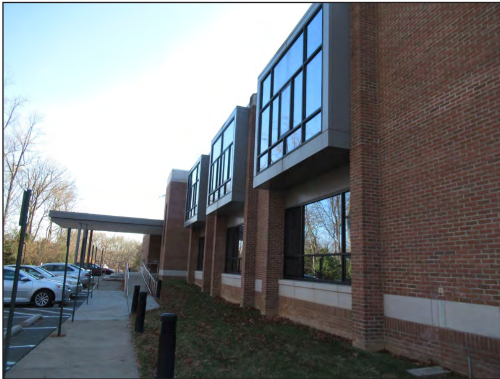
Figure 28. United Christian Parish (029-6444), north elevation, looking east
