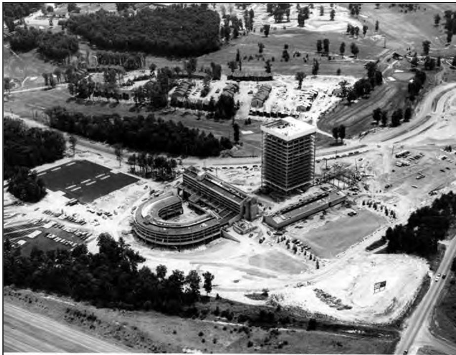
Figure 37. Aerial view of Sheraton Reston Hotel (029-6646) and Reston International Center (029-6753), during construction 1969-1972.
