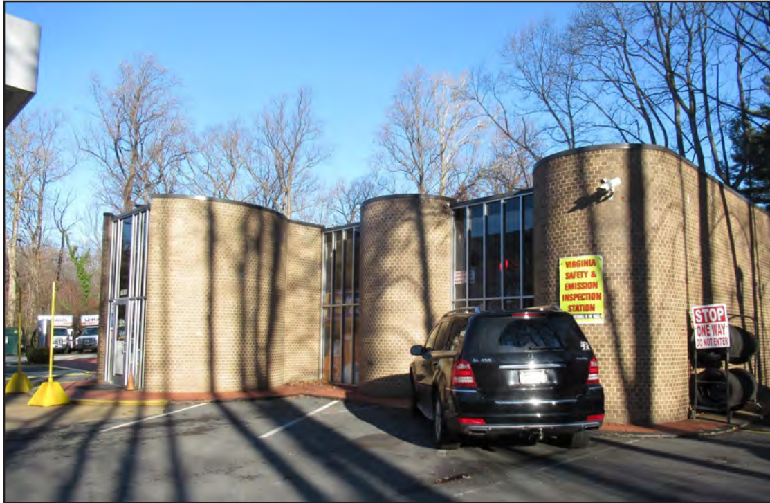
Figure 25. Lake Anne Gas Station, south corner.
