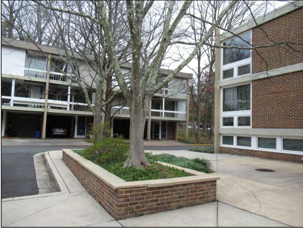
Figure 51. Hickory Cluster (029-6648), north portion of courtyard, looking east.
