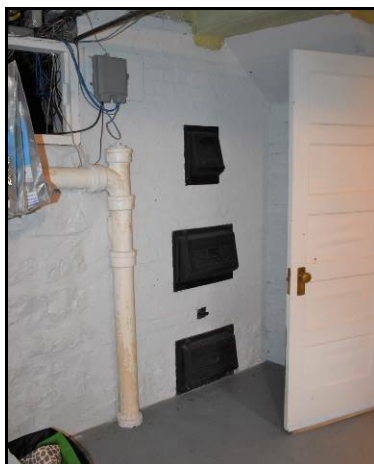
Figure 5. Former incinerator access in basement.
