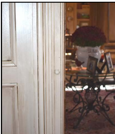
Figure 4. Detail showing call button located in living room door surround.
