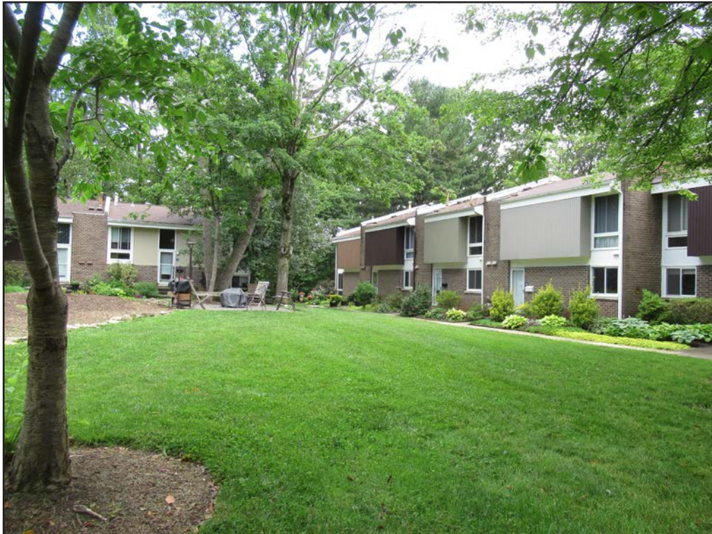
Figure 70. Wainwright Cluster (029-6768), middle cluster, looking northeast.
