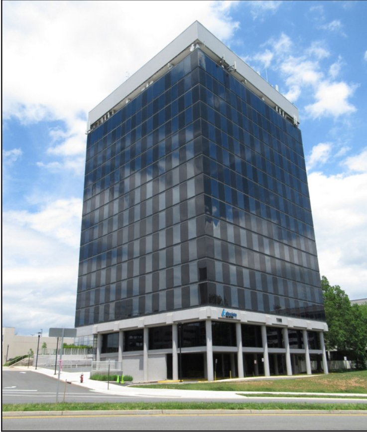
Figure 40. Reston International Center (029-6753), south corner.
