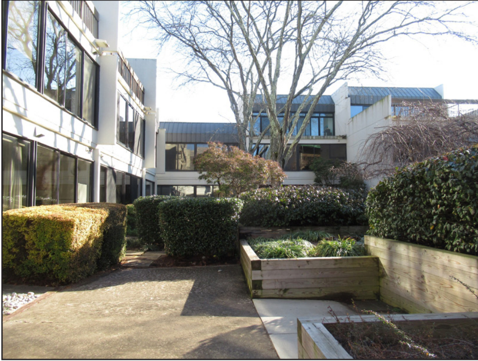
Figure 35. The Atrium (029-6645), courtyard, looking north.
