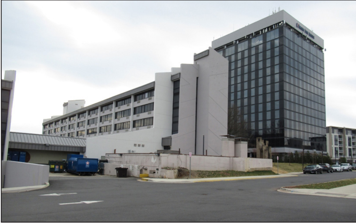
Figure 38. Sheraton Reston Hotel (029-6646), southwest corner.
