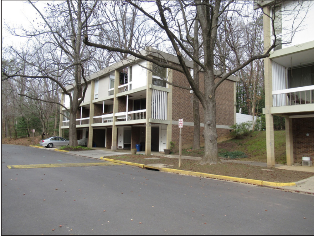
Figure 50. Hickory Cluster (029-6648), north portion of courtyard, looking northeast.
