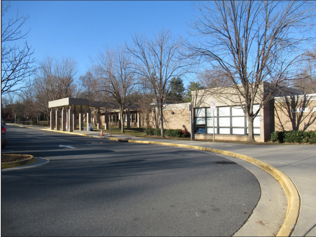
Figure 30. Lake Anne Elementary School (029-6642), northeast elevation (facade).
