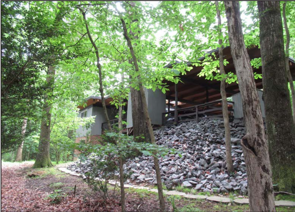
Figure 68. House, 12146 Stirrup Road (029-6755), northeast corner.
