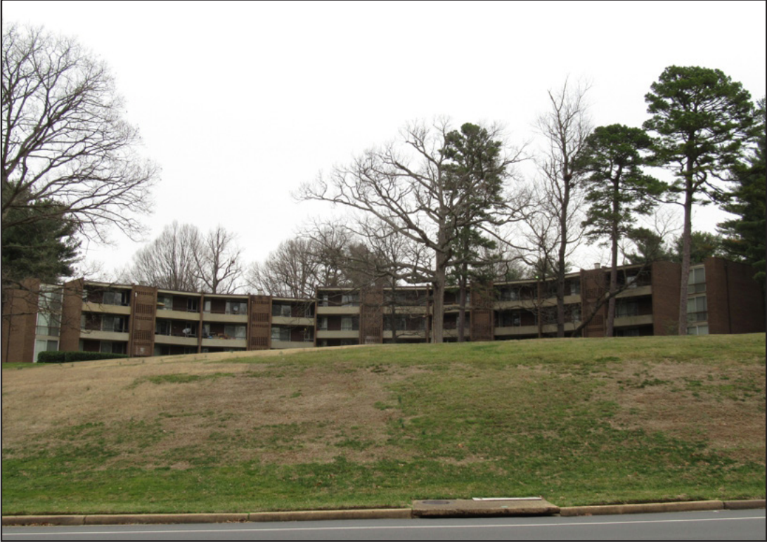
Figure 64. Cameron Crescent Apartments (029-6650), southeast building, looking north.
