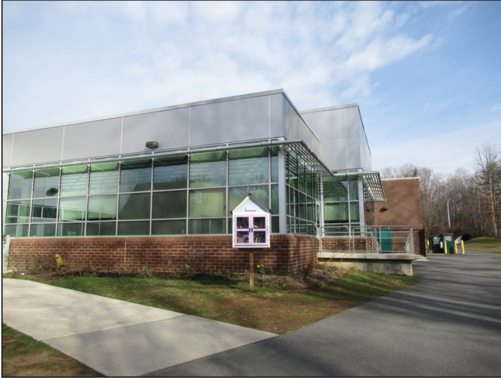
Figure 45. Terraset Elementary School (029-6647), east elevation, looking north.
