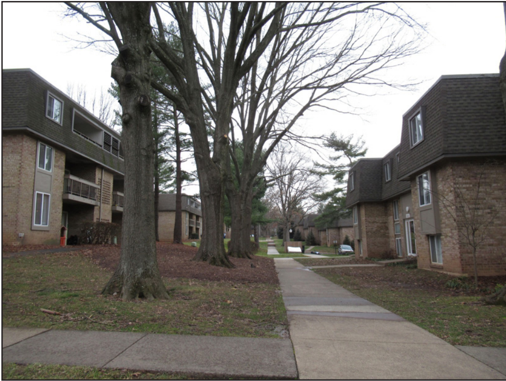
Figure 59. Fairway Apartments (029-6652), West Center Court, looking west.
