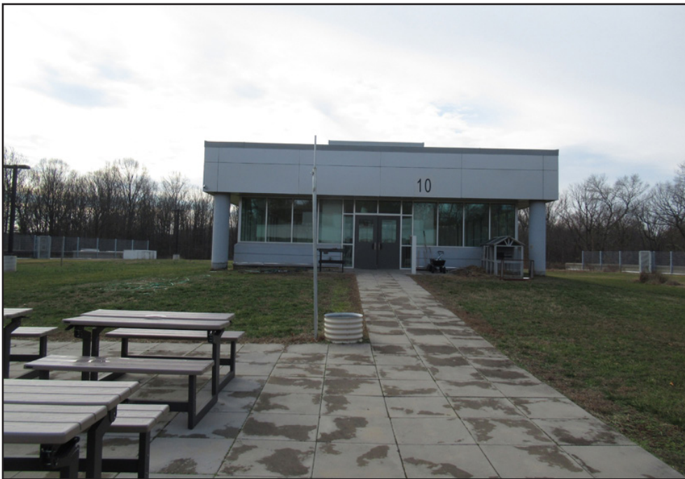
Figure 46. Terraset Elementary School (029-6647), roof, looking south.
