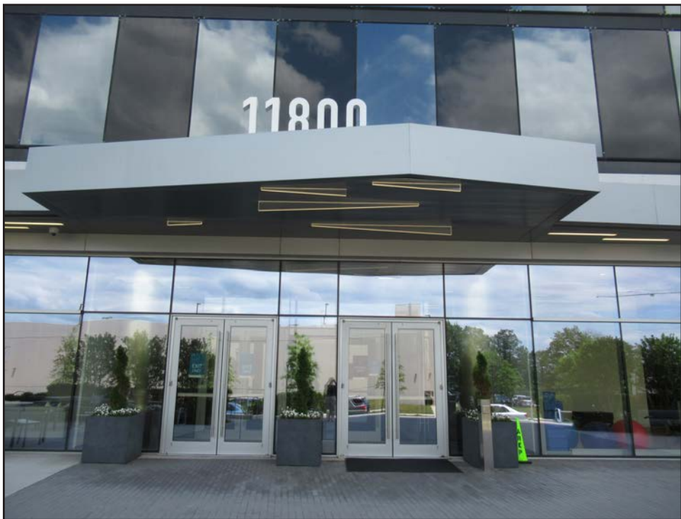
Figure 41. Reston International Center (029-6753), entrance.
