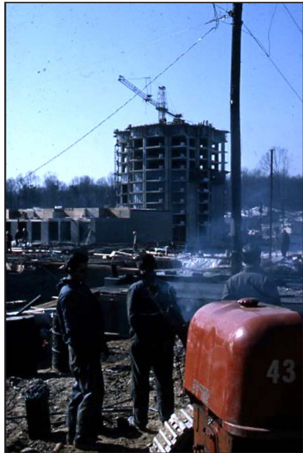
Figure 17. Heron House high-rise apartment building under construction in 1964 (George Mason University Libraries [GMUL] item ID C0001B113_01).
