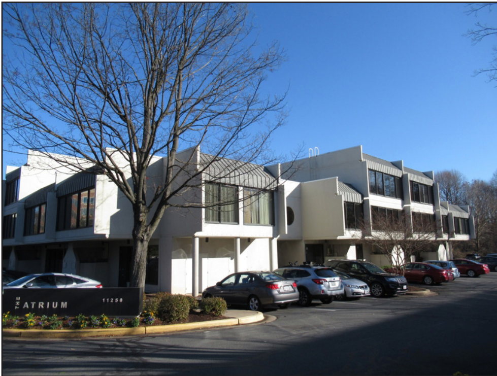
Figure 36. The Atrium (029-6645), southwest corner.
