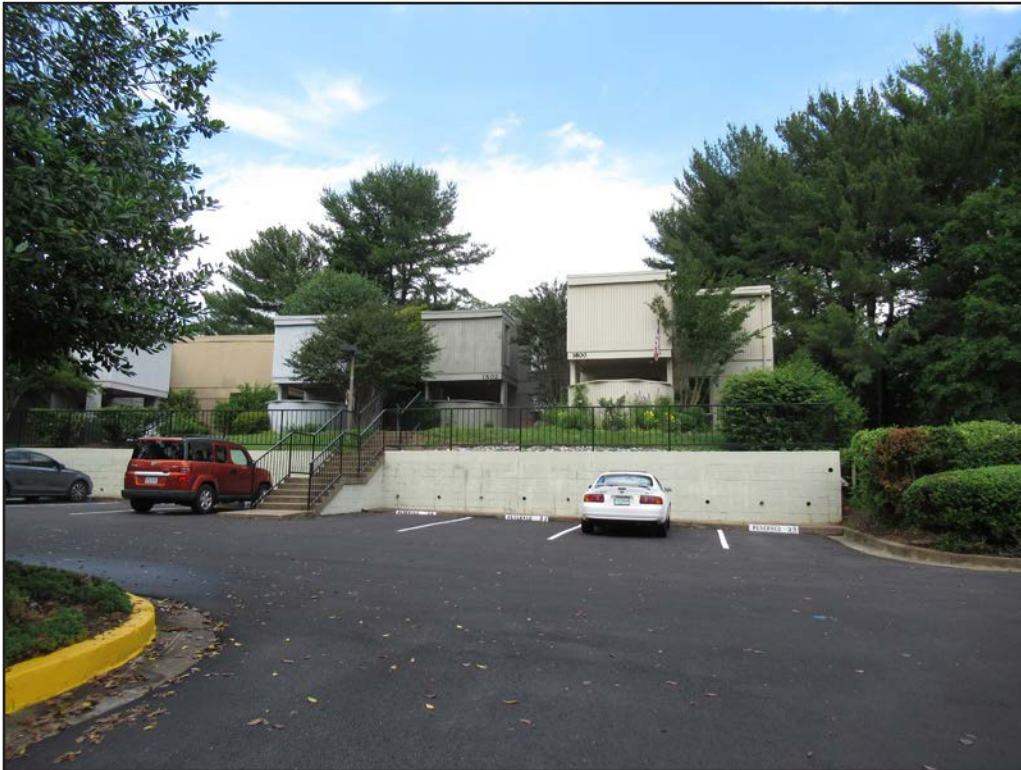
Figure 74. Fairway Cluster (029-6774), Units 1800–1804, looking northwest.
