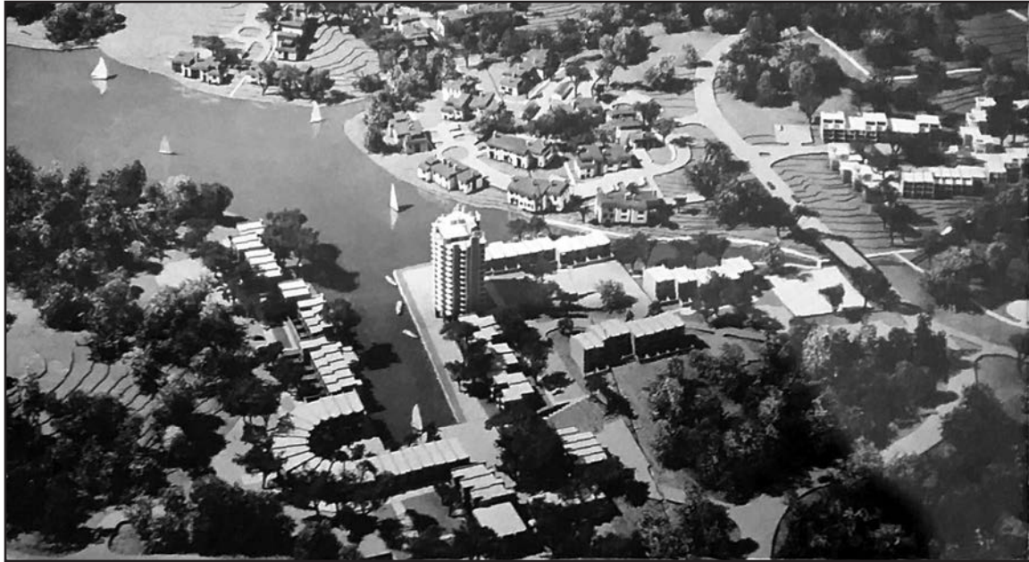
Figure 15. Detail view of a 50 foot to 1 inch scale model of Lake Anne Village presented by Robert Simon's team at a Fairfax County planning hearing (Reston Historic Trust & Museum).
