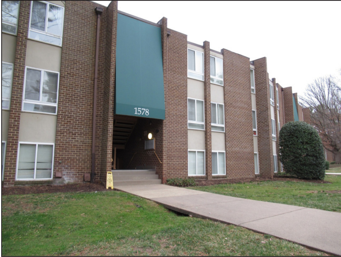
Figure 65. Cameron Crescent Apartments (029-6650), southwest building, southeast entrance.
