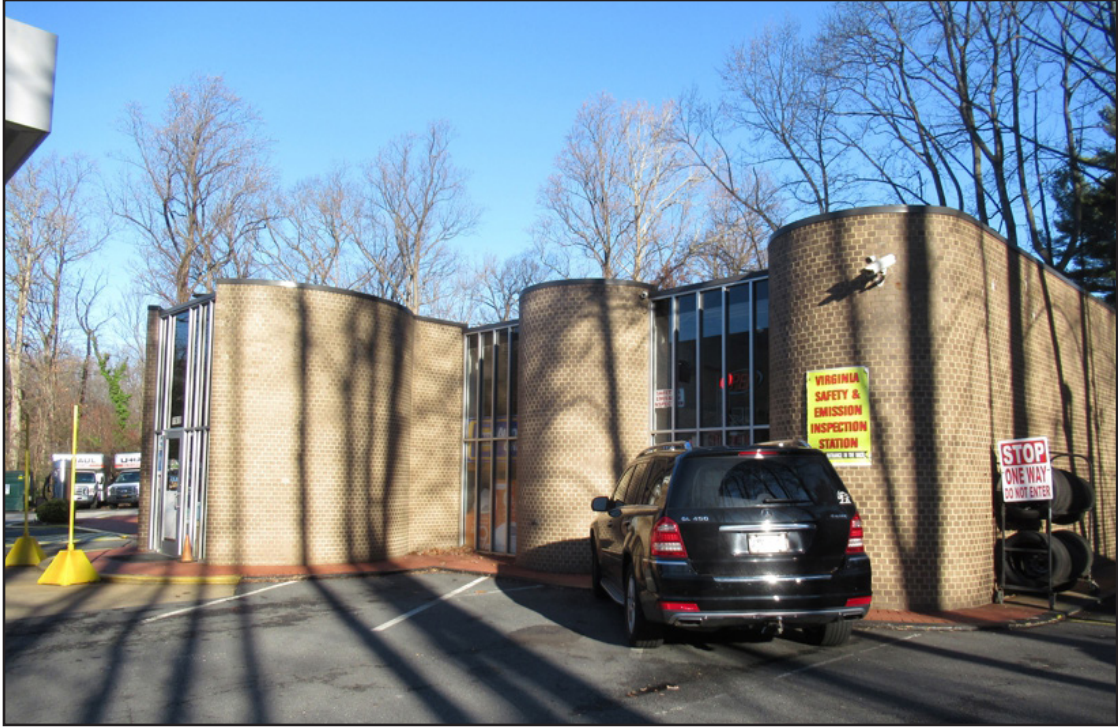
Figure 25. Lake Anne Gas Station, south corner.
