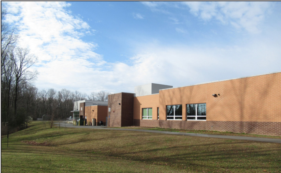
Figure 44. Terraset Elementary School (029-6647), east elevation.
