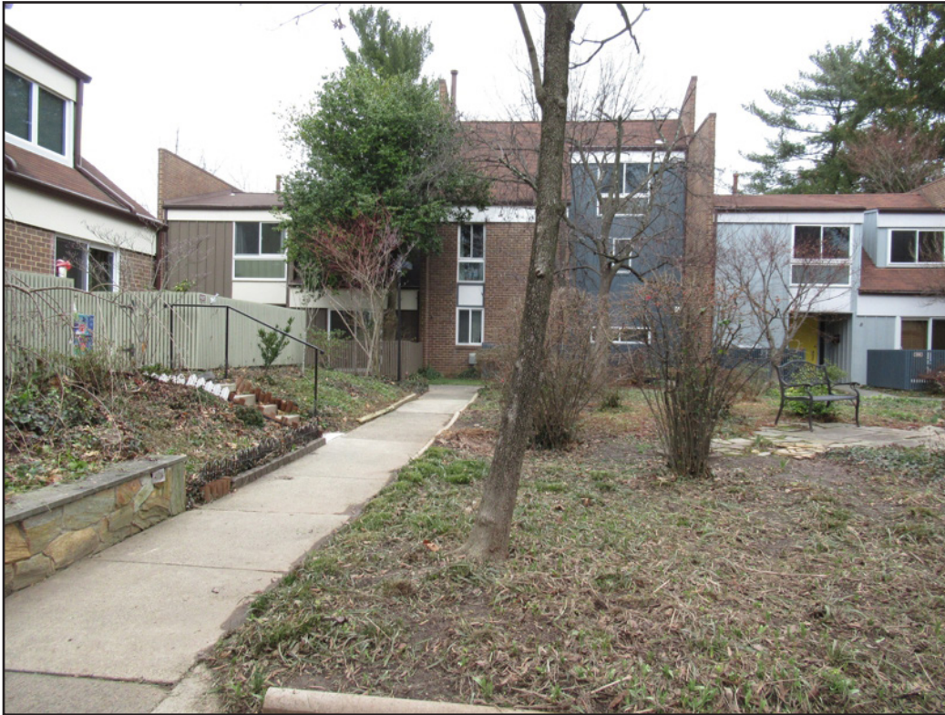
Figure 61. Golf Course Island Cluster (029-6653), southeast section, looking north.
