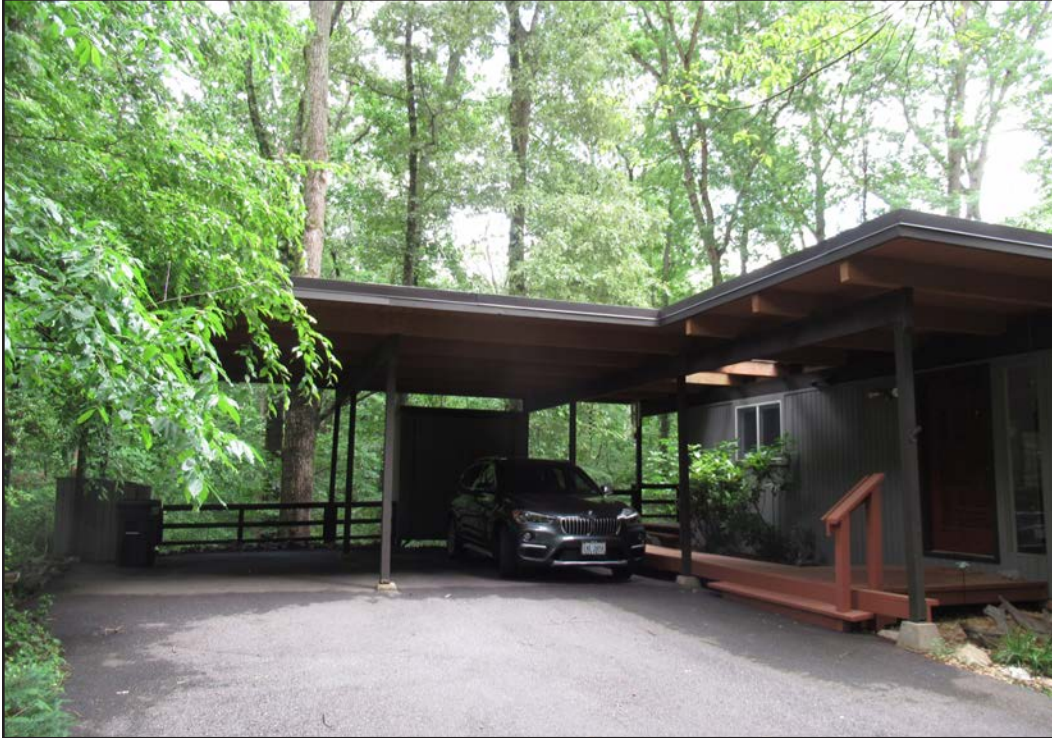
Figure 67. House, 12146 Stirrup Road (029-6755), carport and entrance.
