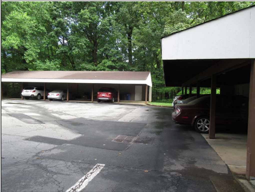
Figure 72. Wainwright Cluster (029-6768), upper cluster carports, looking northeast.
