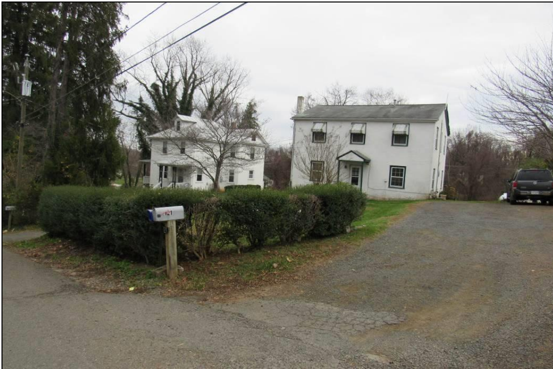
Photo 32: Houses at 121 and 131 Old Mill Lane (155-5141 and 155-5142, Respectively) in Oliver City, Looking Northeast.
