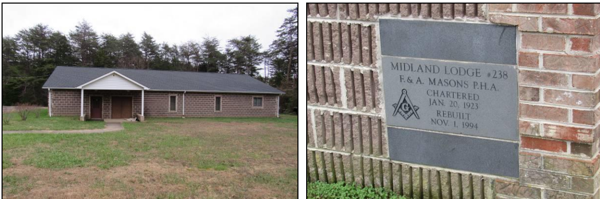
Photo 13: Midland Masonic Lodge No. 238 (030-5899), Northwest Elevation (Left) and Datestone (Right).
