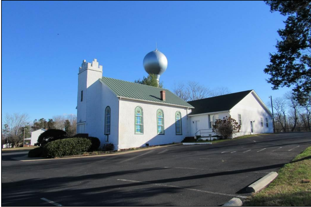
Photo 18: First Springs Baptist Church (030-0298/030-5427-0192), in Turnbull, Southwest Oblique.
