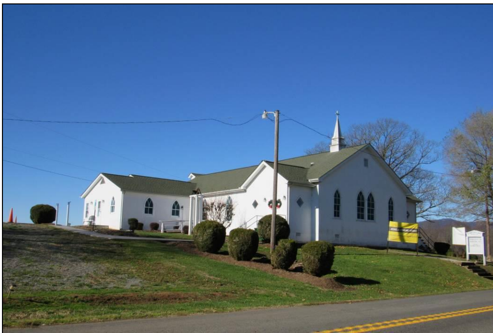
Photo 2: Mt. Morris Primitive Baptist Church (030-5893) in Hume, Southeast Oblique.
