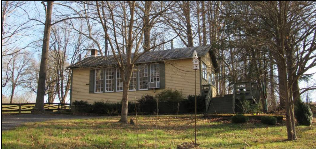
Photo 8: Delaplane School (030-5361), Northwest Oblique.
