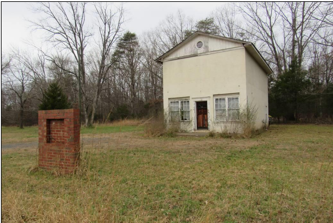
Photo 14: Store, 5228 Old Auburn Road (030-5140-0021), Southeast Oblique.
