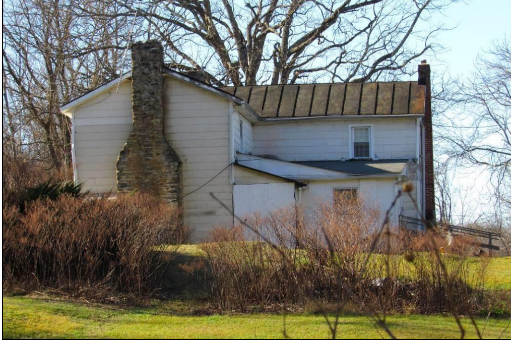
Photo 20: Gaskins House, 3702 Sage Road (030-0656) in The Sage or Sagetown, East Elevation.
