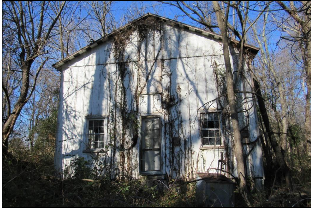
Photo 12: Mt. Olive Odd Fellows Lodge #10966 building (030-5434-0253), East Elevation.
