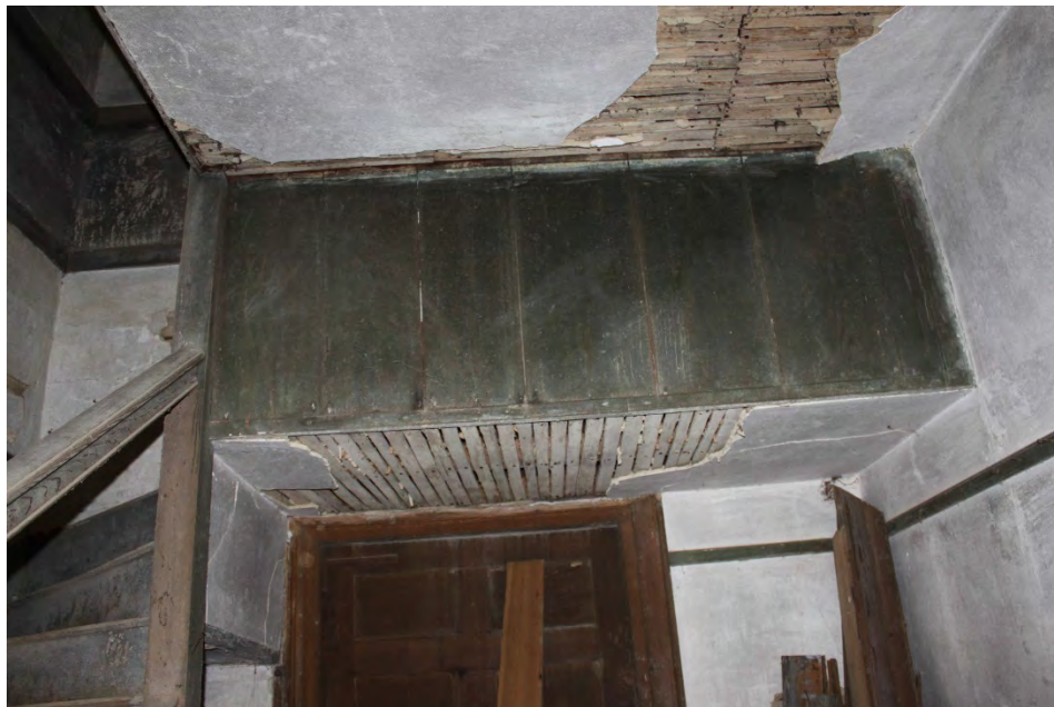
Figure 7, detail of the possibly modified stair landing from the first floor stair passage. Note the rough-cut vertical boards used as facing at the landing, Elizabeth Lipford, DHR archives photograph, 2021
