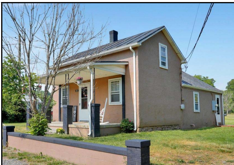
89 Gooney Alley Road. Worley and Violet Updike House (093-0241; 093-5032-0017 ).
