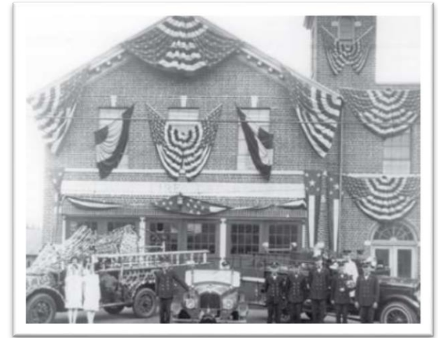
TOWN OF POTOMAC, ARLINGTON COUNTY, TOWN HALL AND FIREHOUSE, CA. 1926. DESIGNED BY FRANCIS DRISCHLER AND CONSTRUCTED BY D.E. BAYLISS.
