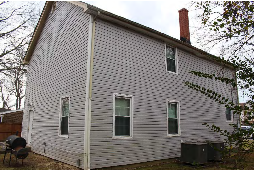
Photo 4 of 8: North and East (rear) Elevations, facing southwest
