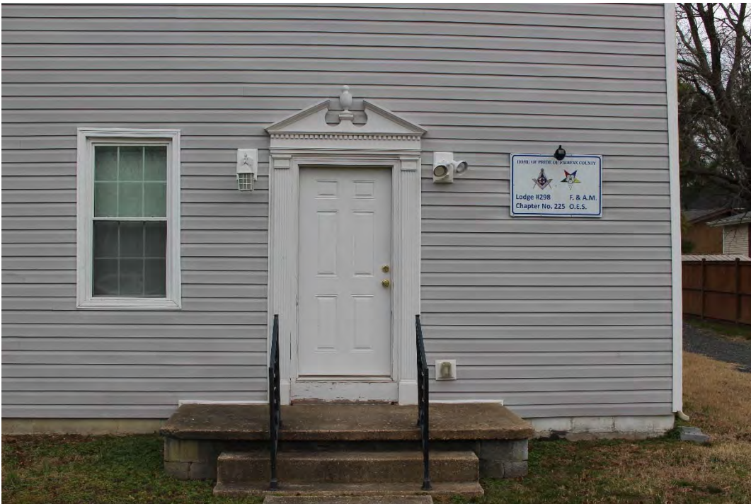
Photo 2 of 8: Main entrance detail on West Elevation, facing east
