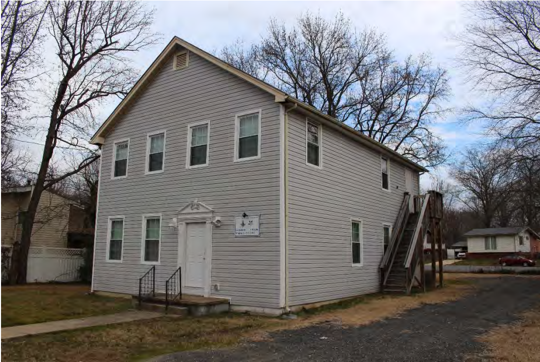
Photo 1 of 8: West (front) and South Elevations, facing northeast
