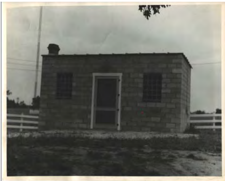
Original 1947 transmitter building and radio tower. This building is now the east wing of the 1953 station and has been parged. Photo in the collection of WSVS Pure Country Radio Station.
