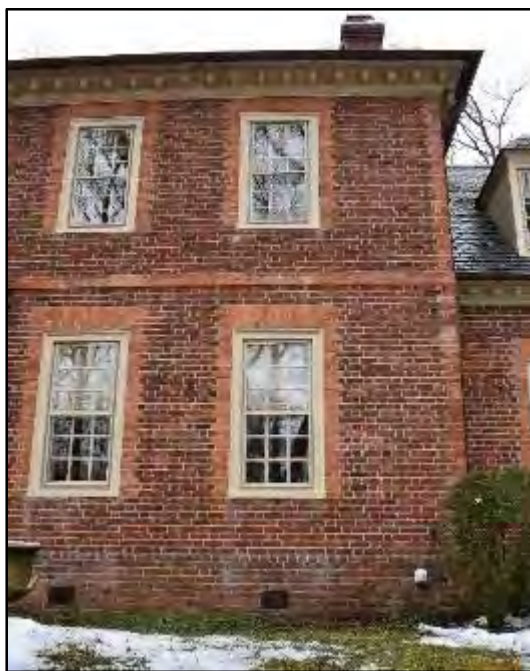
Figure 8. East elevation detail showing brickwork.
