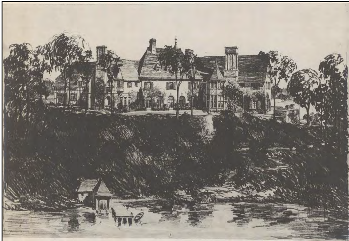
4. Sketches of the Frank D. Stranahan House, Perrysburg, Ohio. The top image is a rendering of the house’s land side (south) by architect Charles S. Schneider. The bottom image of the house is by Olmsted Brothers showing the river side of the house, embellished with gardens and landscape. The setting is notable for its similarities to the setting of Clovelly in Virginia.
