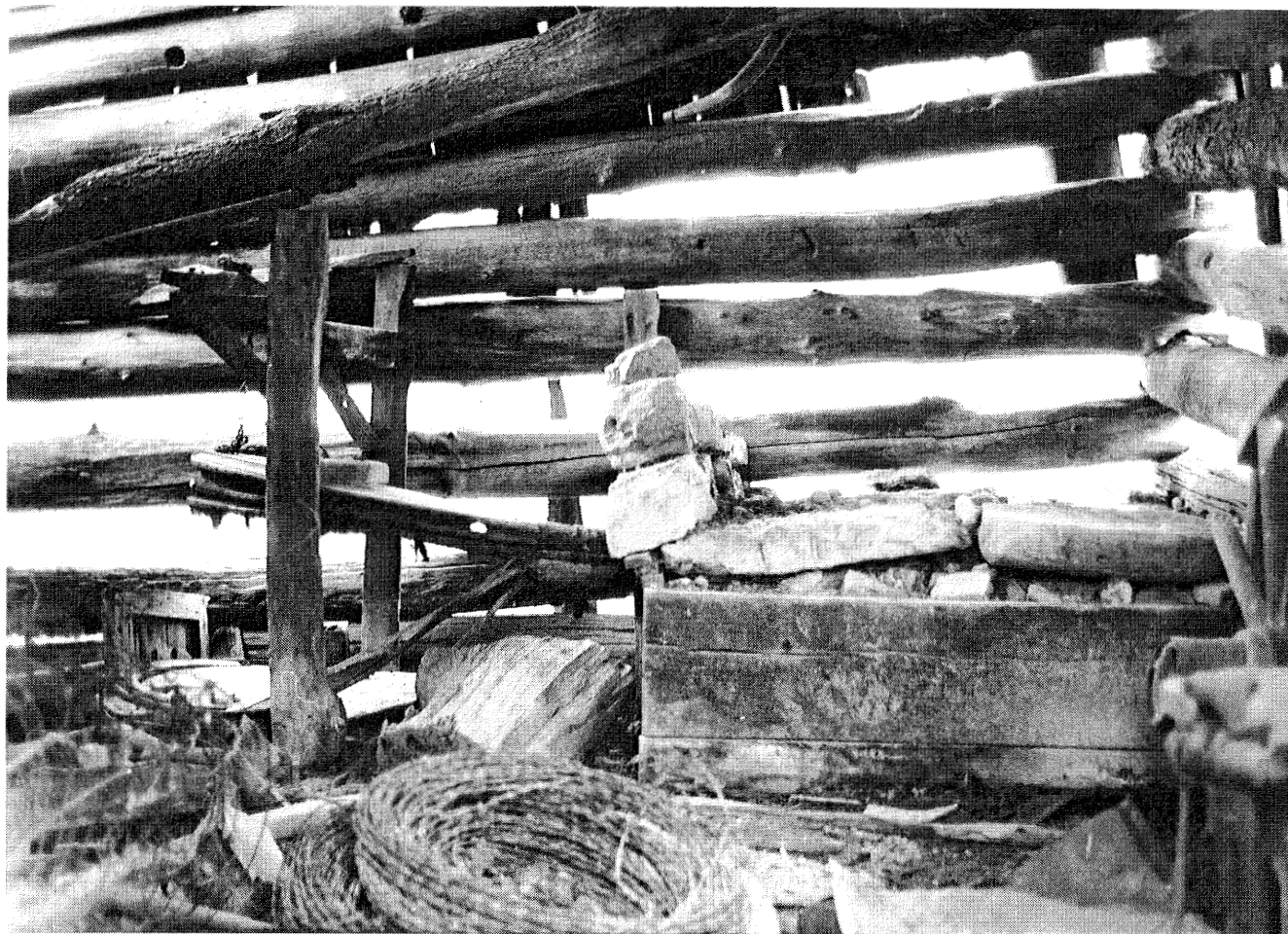
Plate 3. Bellows and forge, Woods Distillery/Blacksmith Shop.
