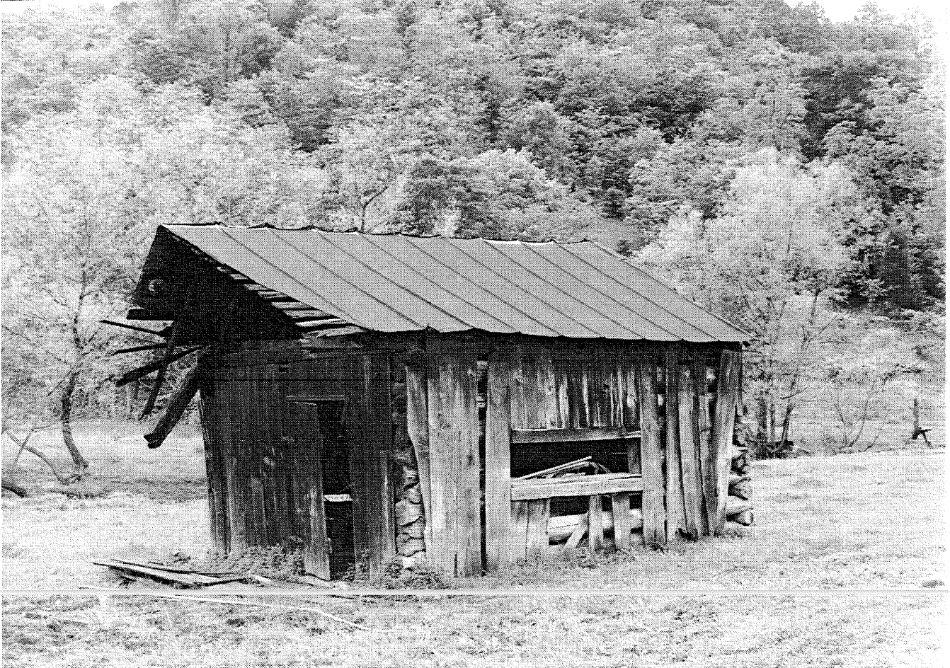
Plate 1. Exterior of the Woods Distillery/Blacksmith Shop.
