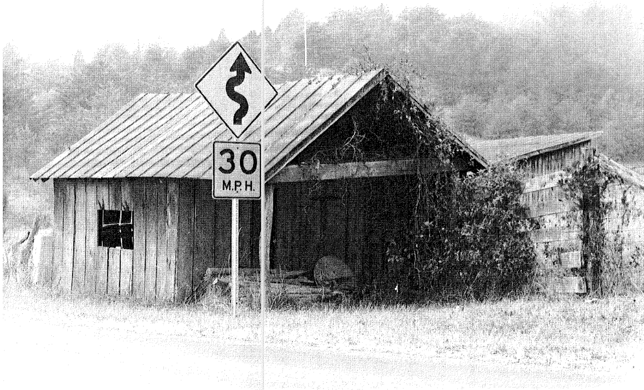
Plate 6. Exterior of the Starkey Blacksmith Shop.
