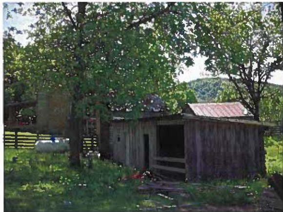
Photograph 9. A contemporary shed attached to the Smokehouse
