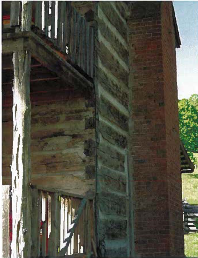
Photograph 4. Detail of the Corner Notching
