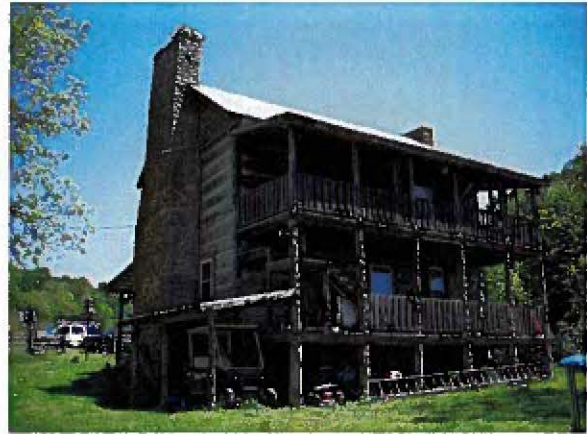
Photograph 6. A shed appended to the Rear Elevation
