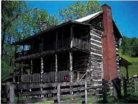
Photograph 5. The Rear Elevation features a two-story, full-width porch
