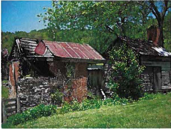
Photograph 7. The deteriorating Springhouse and the Smokehouse
