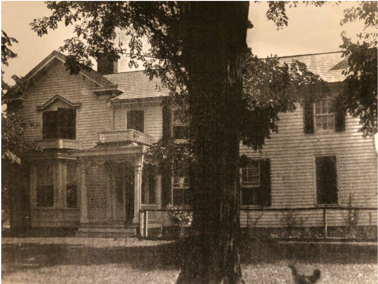
Figure 2. La Fourche, south elevation, ca. 1860.
