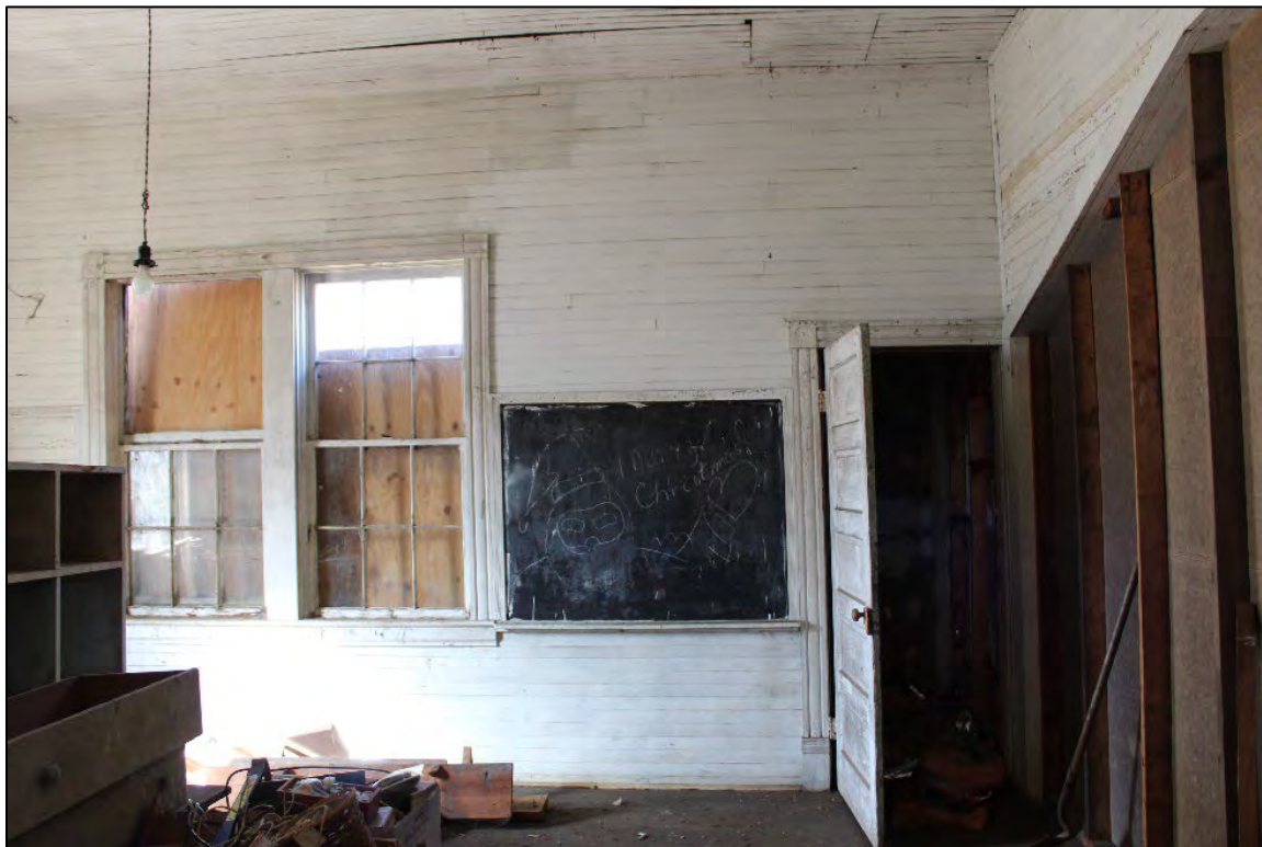
Building A, interior, south classroom, front wall. December 2021.
