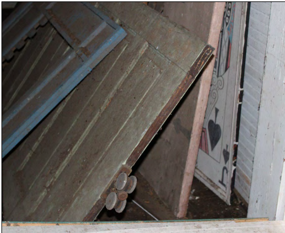
One of the original sliding doors that was used to divide the classrooms when Ms. Napier and Ms. Mitchell attended Ryan Hall in the 1950s retains the original wheeled hardware that allowed it to roll along a hanging track. This door is stored in Building A; another original door is reused in the modern partition wall in Building A but is missing the hardware. January 2022.
