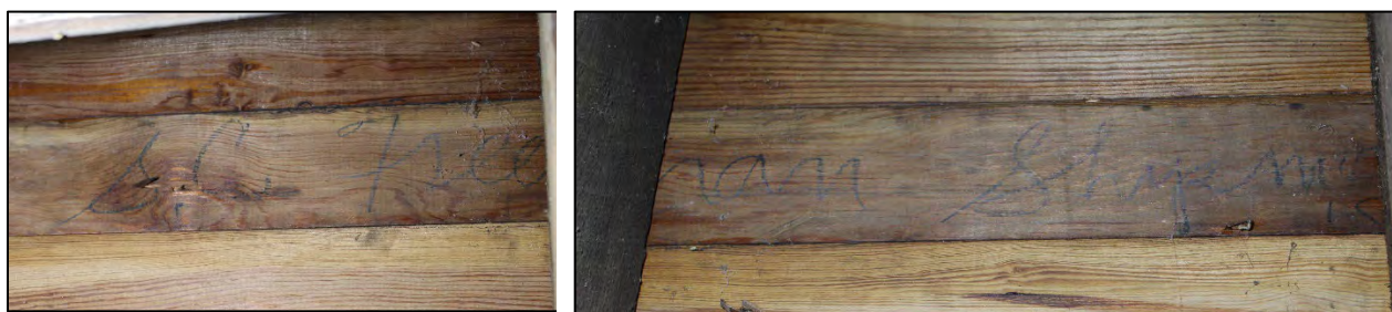
Building A, basement room, script on underside of floorboards, "S.C. Freeman Shipman". January 2022.
