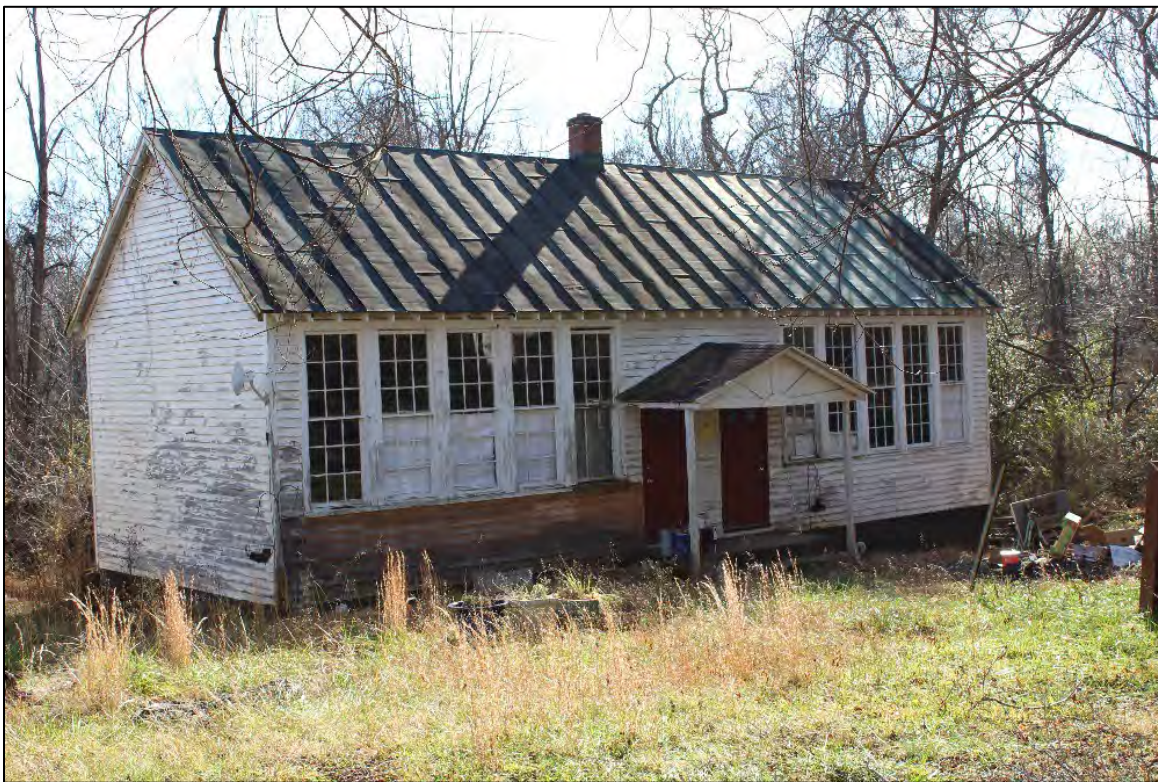
Building B, northwest oblique. December 2021.
