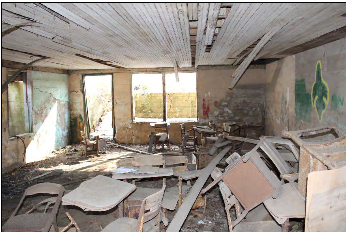
Building A, basement classroom, looking from front wall toward rear wall. Ghost of stair is visible in far right corner. January 2022.
