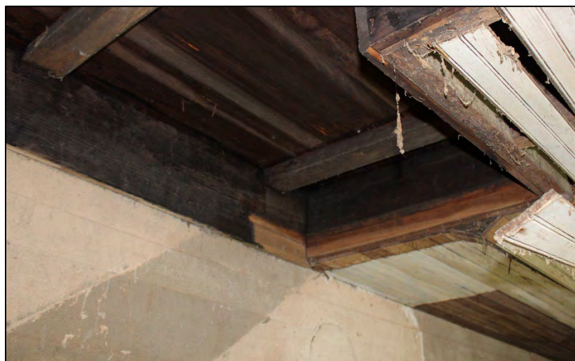
Ghost of the top step of the flight of stairs that connected the basement to the main floor. Mr. Scott used this stair to collect his lunch from where it was prepared in the basement when he attended school at Ryan Hall in the 1940s. January 2022.
