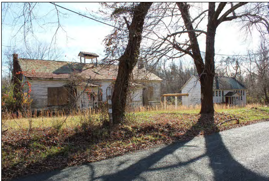
Ryan Hall Elementary School, view from Braddock Lane looking southeast, Building A on the left, Building B on the right. December 2021.
