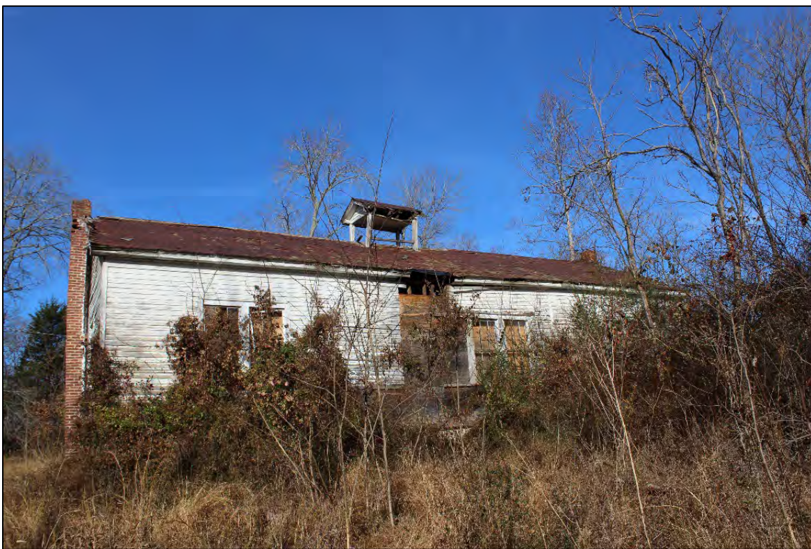
Building A, rear (east) elevation. December 2021.
