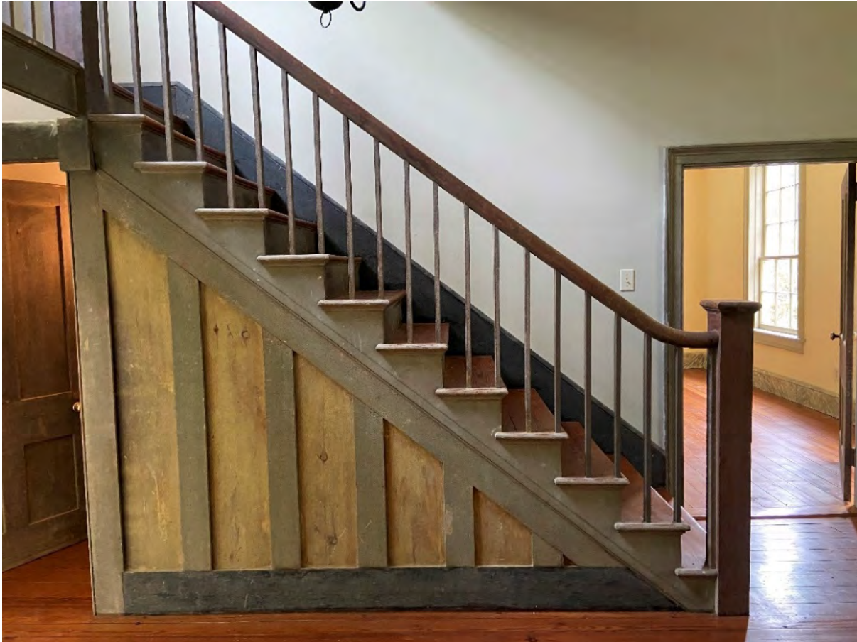
Figure 3 Central stair facing east painted with black, greenish-gray, yellow ochre, and red-brown umber.
