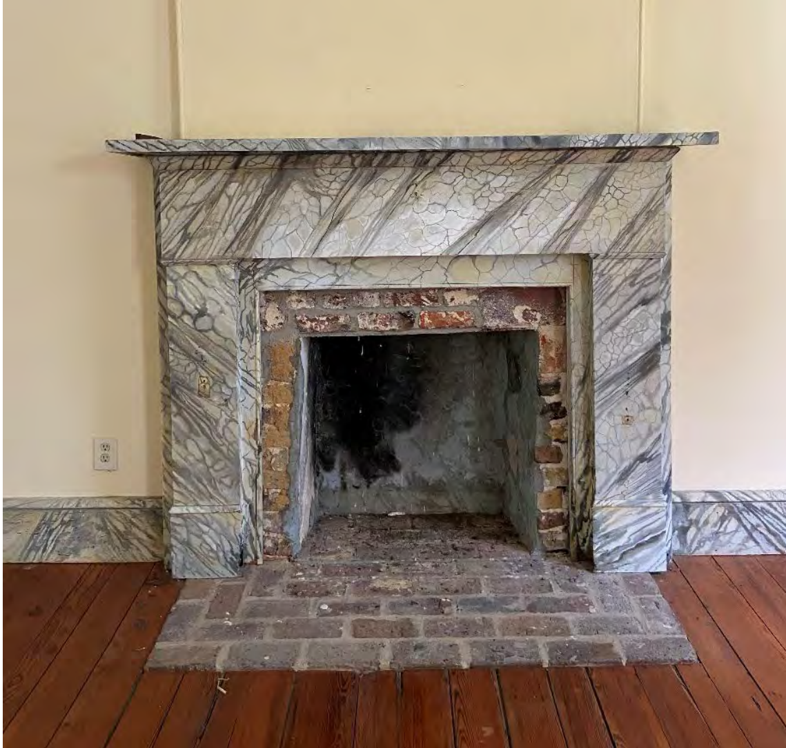
Figure 5 Decorative marbling on the mantel and baseboards in the parlor (first-floor, east room)
