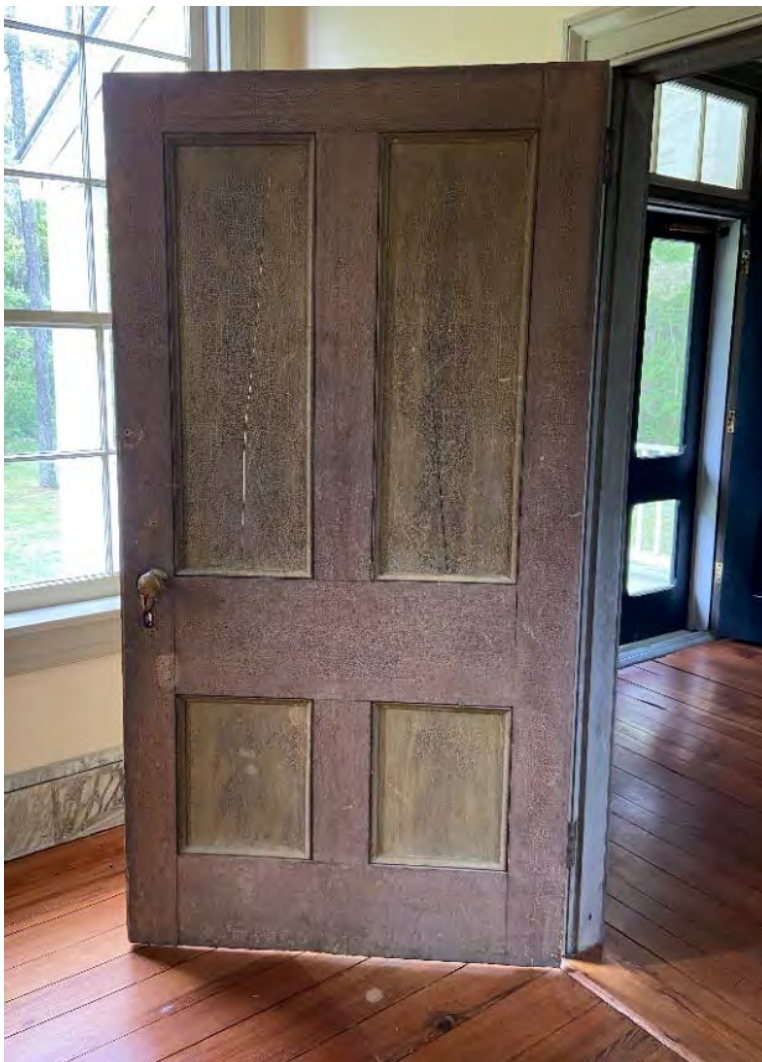
Figure 4 Typical door painted with red-brown umber stiles and rails contrasting with yellow ochre panels.
