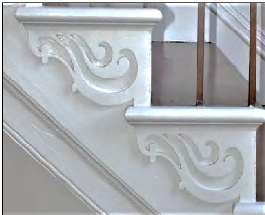
Figure 5. Stair stringer detail.
