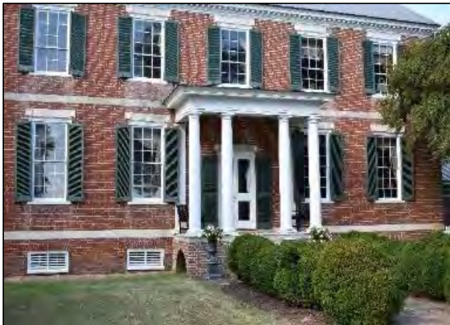
Figure 2. Detail of Chatham's south (landside) façade.
