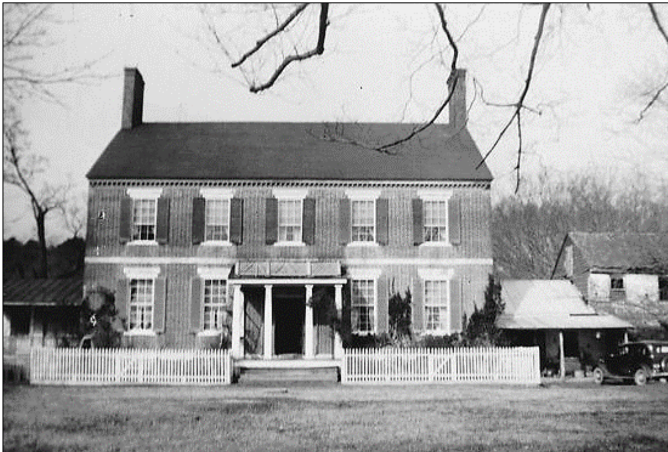
3. Chatham, looking south, [ca. 1938]. Note west end wing (doctor's office) and two-story brick east end wing are still extant. Source: Virginia Historical Inventory, Earl Van Ness and Mattie Scott, 'Chatam' (sic), NTH-20, Survey Report and Photograph, Library of Virginia, Richmond.
