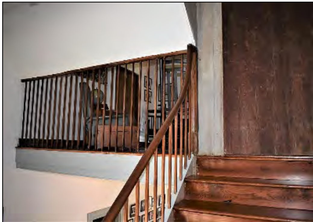
Figure 11. Third-floor ceiling extending to railing; plank door to right.
