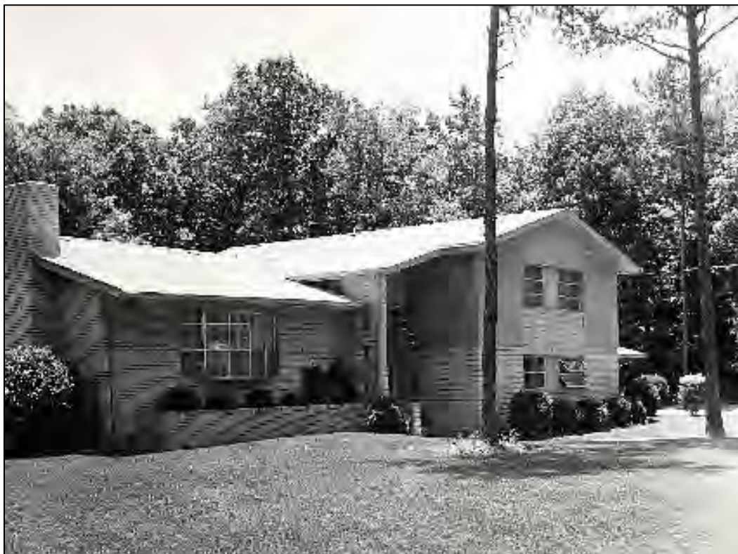
Figure 15. Split-Level house at 1001 Dulcie Avenue built for J. Hugo Madison, ca. 1963 (134-5608-0064). Photograph courtesy of Edna Hawkins Hendrix.
