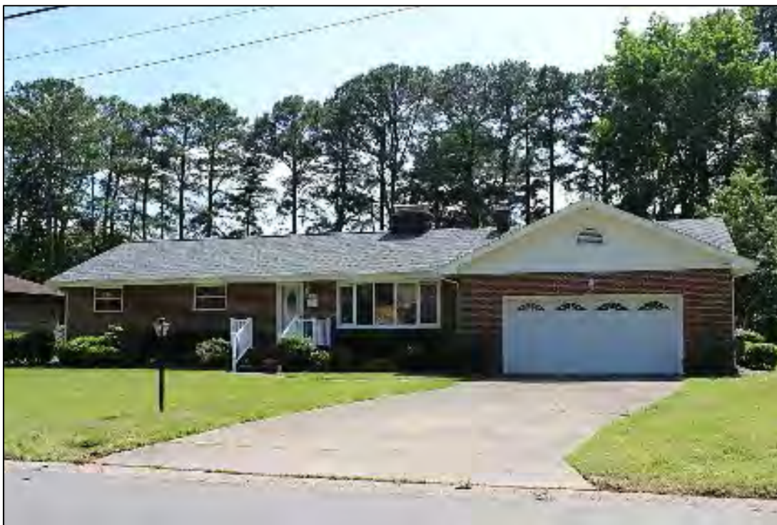
Figure 14. House built by Elmer Harris (1024 Dulcie Avenue (134-5608-0075).
