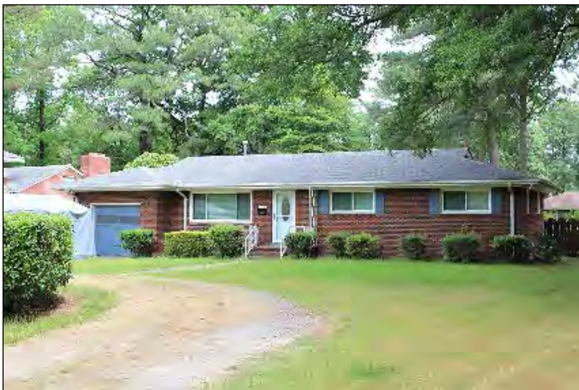
Figure 7. DeLoatch design featuring gable-on-hip roofline with projecting hip over garage (6004 Wesleyan Drive, 134-5608-0112).
