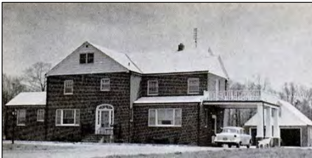
Figure 4. Dr. John T. Sydnor house, 1955, as depicted in Jet magazine (May 26:16). Note porte cochere and freestanding, two-car garage (5913 Northampton Road, 134-5608-0086).
