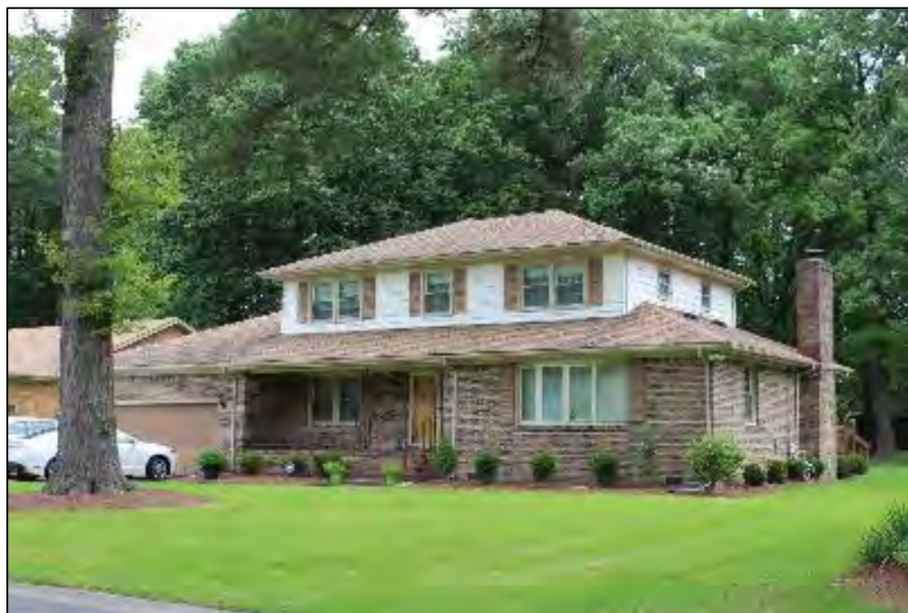
Figure 12. Munford House, built in 1969, 1025 Dulcie Avenue (134-5608-0076).
