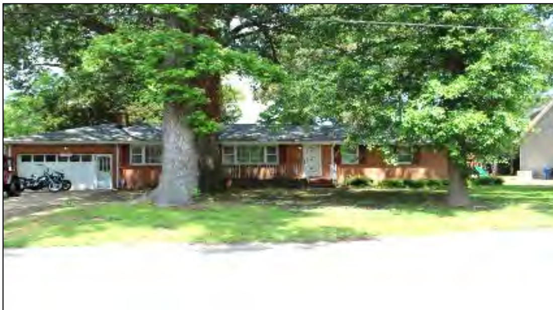
Figure 10. Shropshire House at 5908 Tajo Avenue (134-5608-0100).
