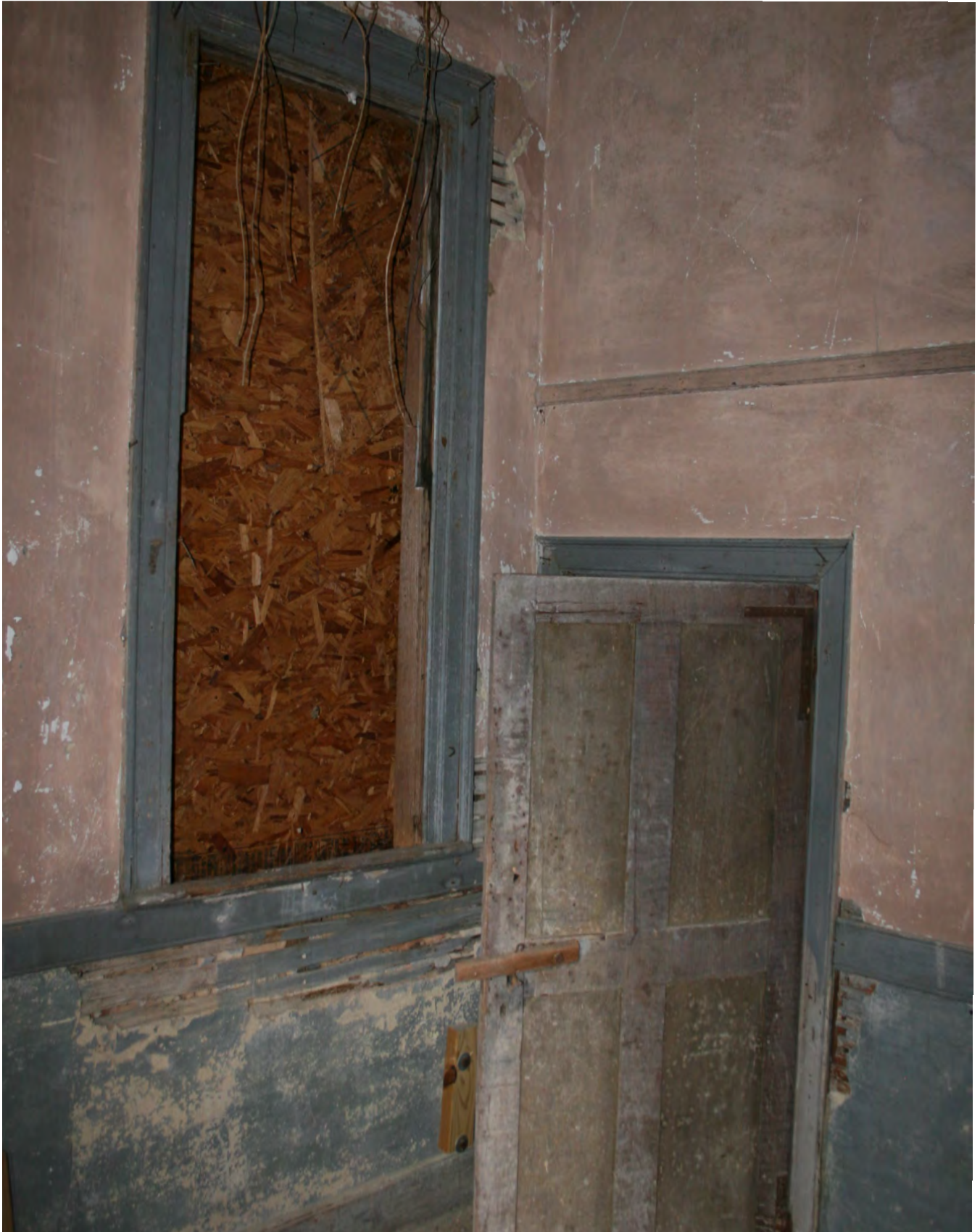
Room 2 looking northeast, 2021
