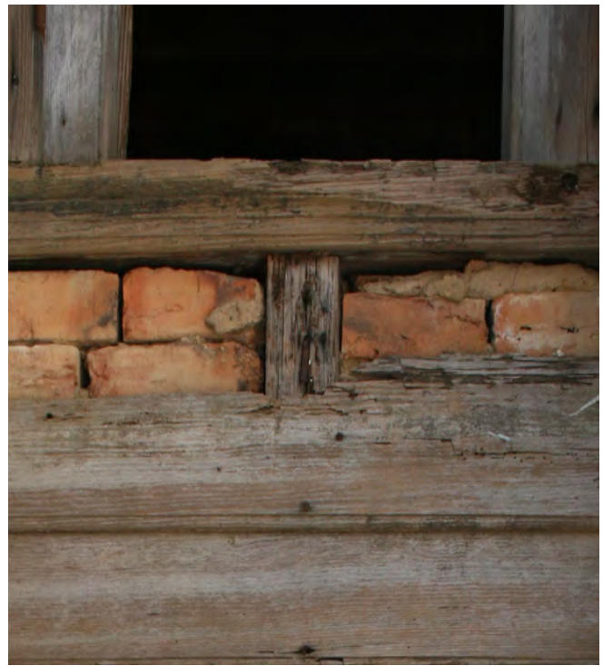
Damage to the sill on the north elevation (left) and typical brick nogging and weatherboards on the north elevation (right).
