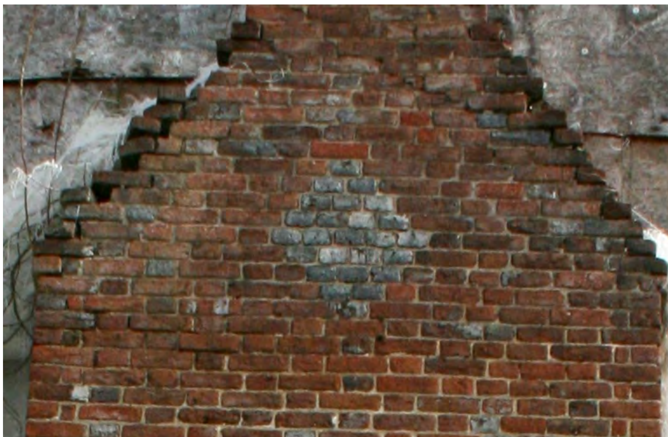
North elevation looking southeast (above) and shoulders and diaper ornament, west chimney (below), 2021.
