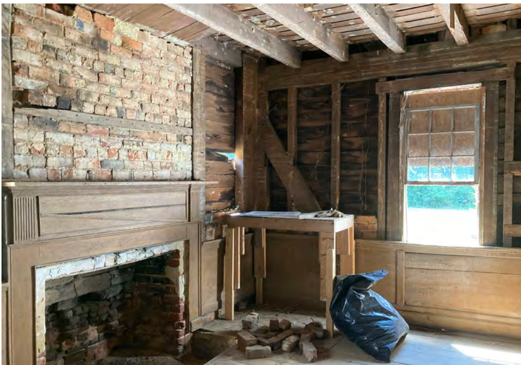
First Floor, Parlor looking southeast.
