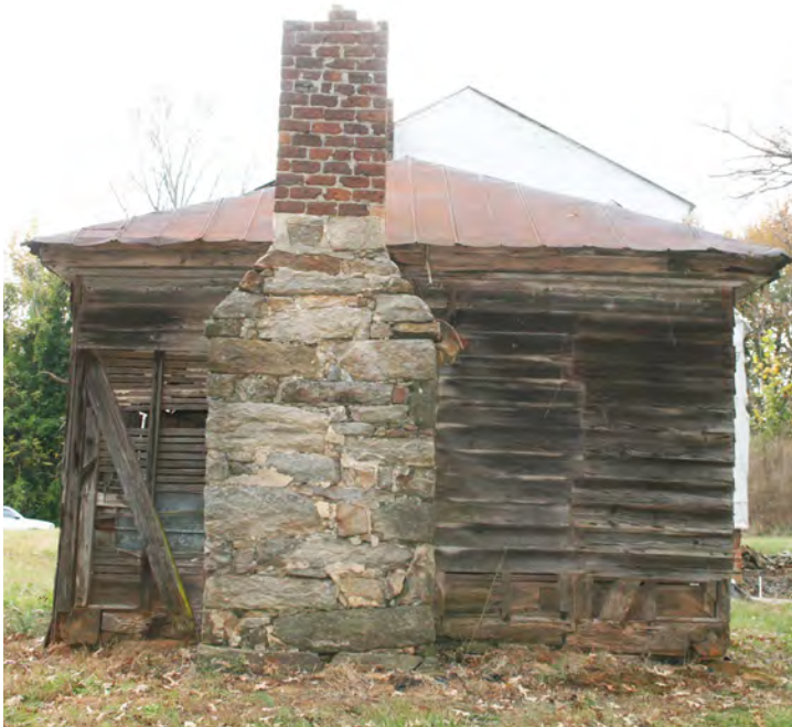
Kitchen, known today as the "Weaving House" or "Spinning House" from the east (left). Note the cut in siding, chimney posts and down braces indicating the location of larger original chimney. Stone chimney at secondary house site to east of the main house seen from northwest (right).
