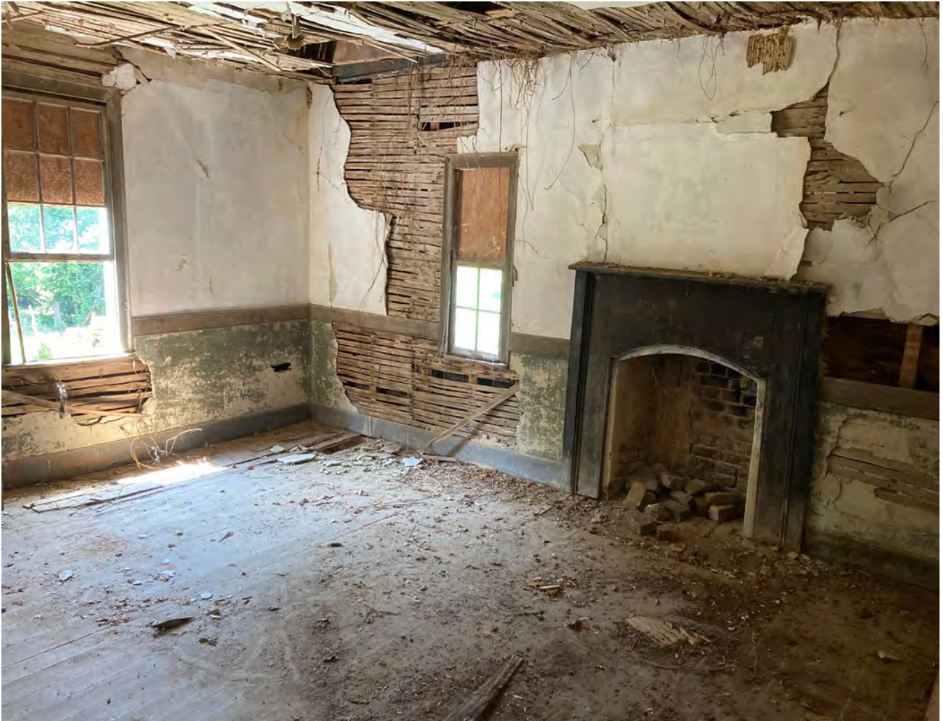
Second Floor, Chamber 1 looking southwest.
