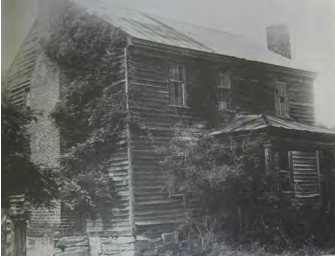
Southwest corner from the southwest showing repaired foundation, 1970s [Corker, Collection Old Brunswick Circuit Foundation].
