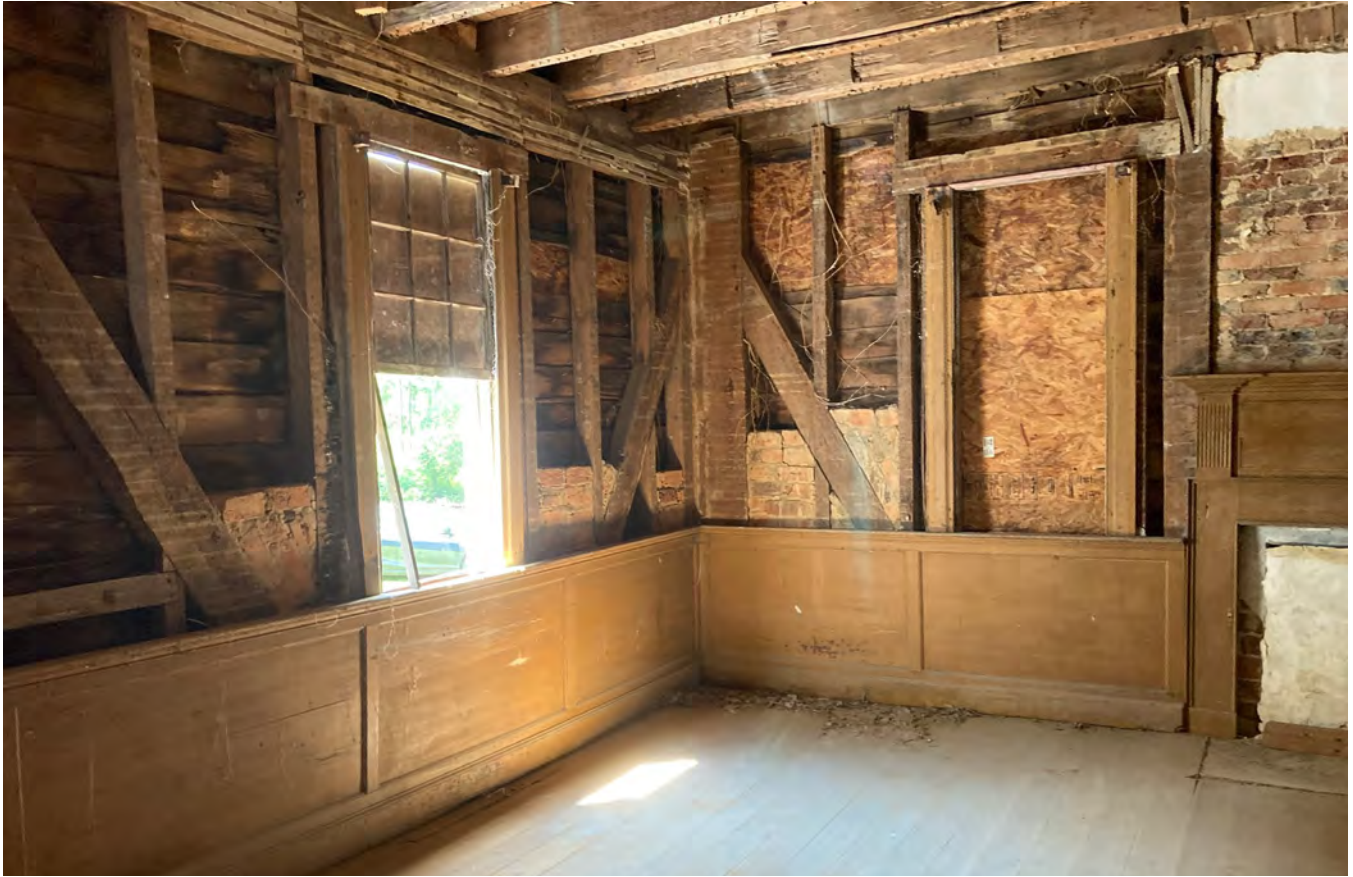
First Floor, Hall looking southwest.
