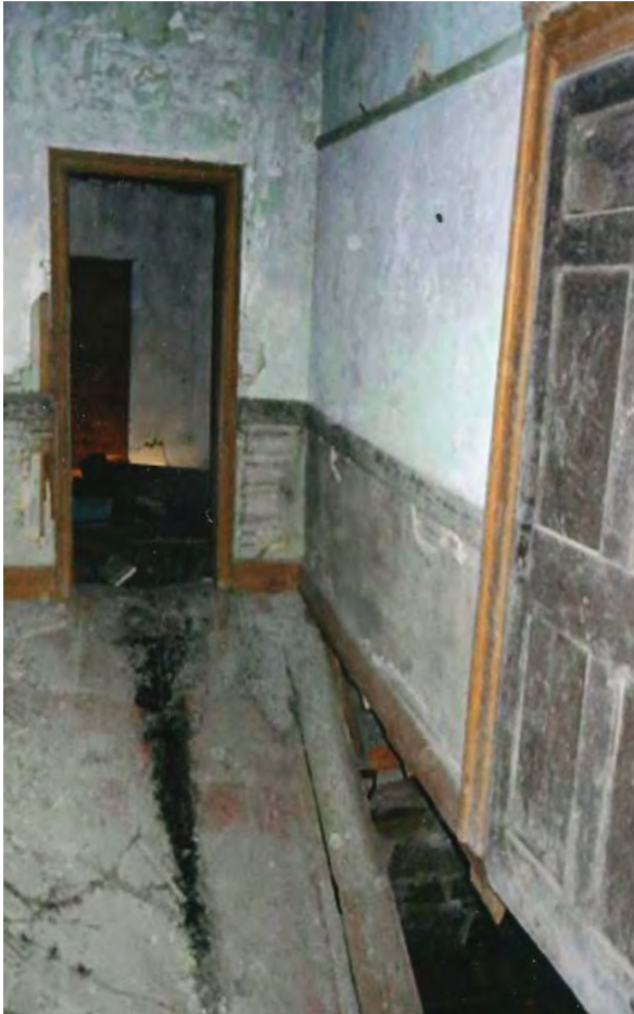
First Floor, Room 1) showing appearance before the floor was repaired c. 2013. The floor had dropped with the collapse of the rotted joists below (left). First Floor, Parlor, chimney breast showing damage to hearth, floor and fireplace interior (right).
