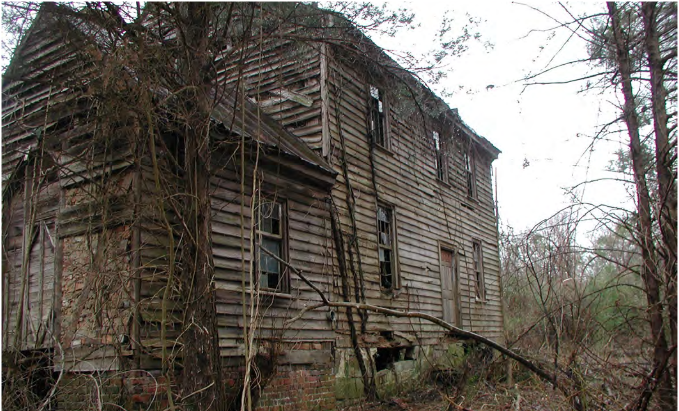
Dromgoole House, north elevation from southeast.
