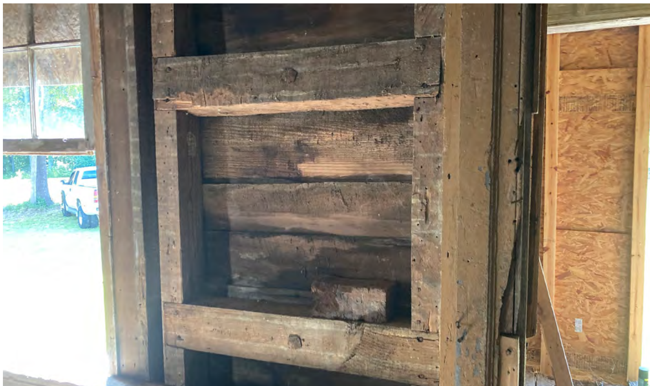
Parlor, detail showing framing and pegs attaching porch pilasters to frame looking south (above) and Parlor looking west (below), 2021.
