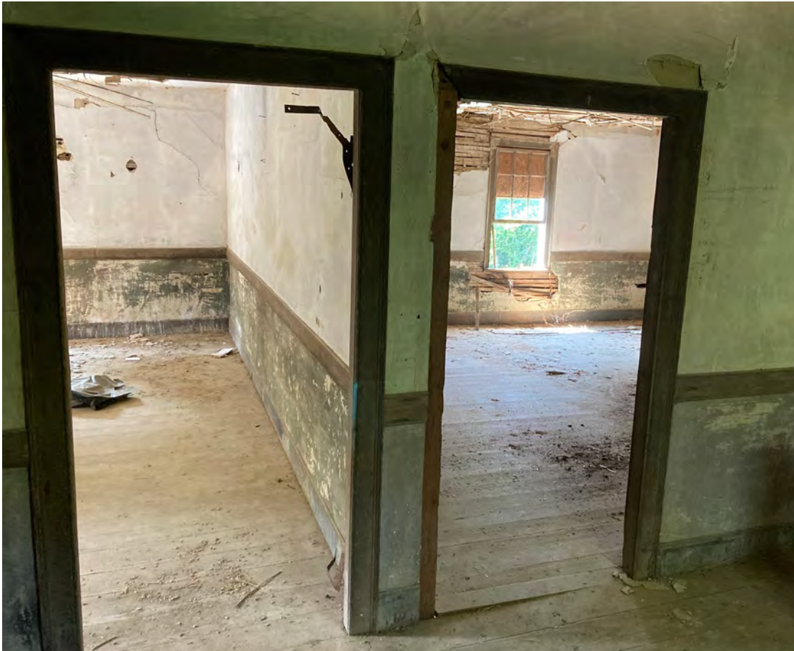
Second Floor, Chambers 1 and 2 seen from Upper Passage looking south.
