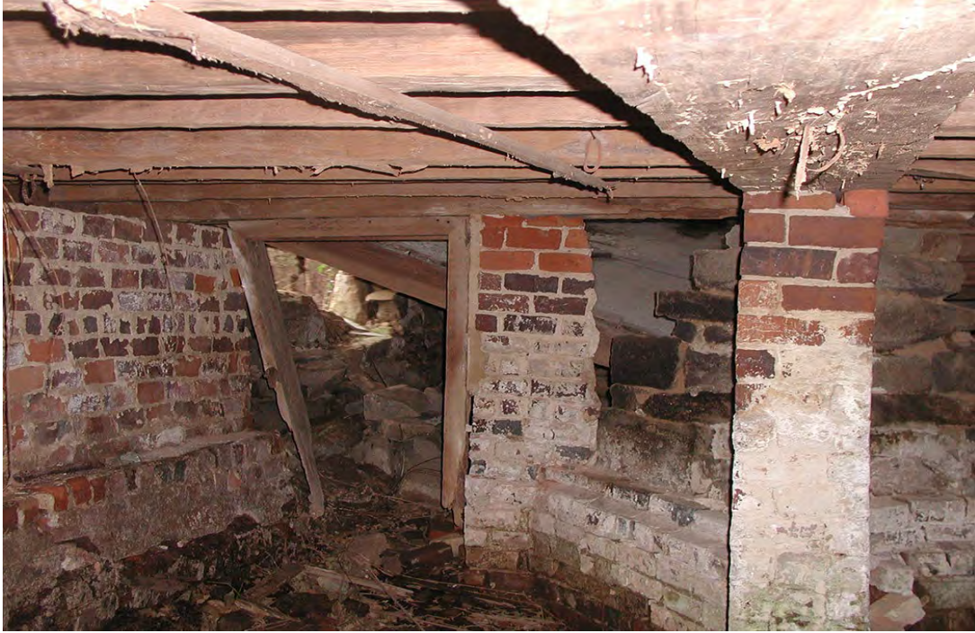
Basement- view of the north half of the Basement looking east showing the diagonal pier and added brick partition to the right. The door frame, no longer in place after the repairs of 2013, connected the room on the east side of the Basement with the room(s) on the west.
