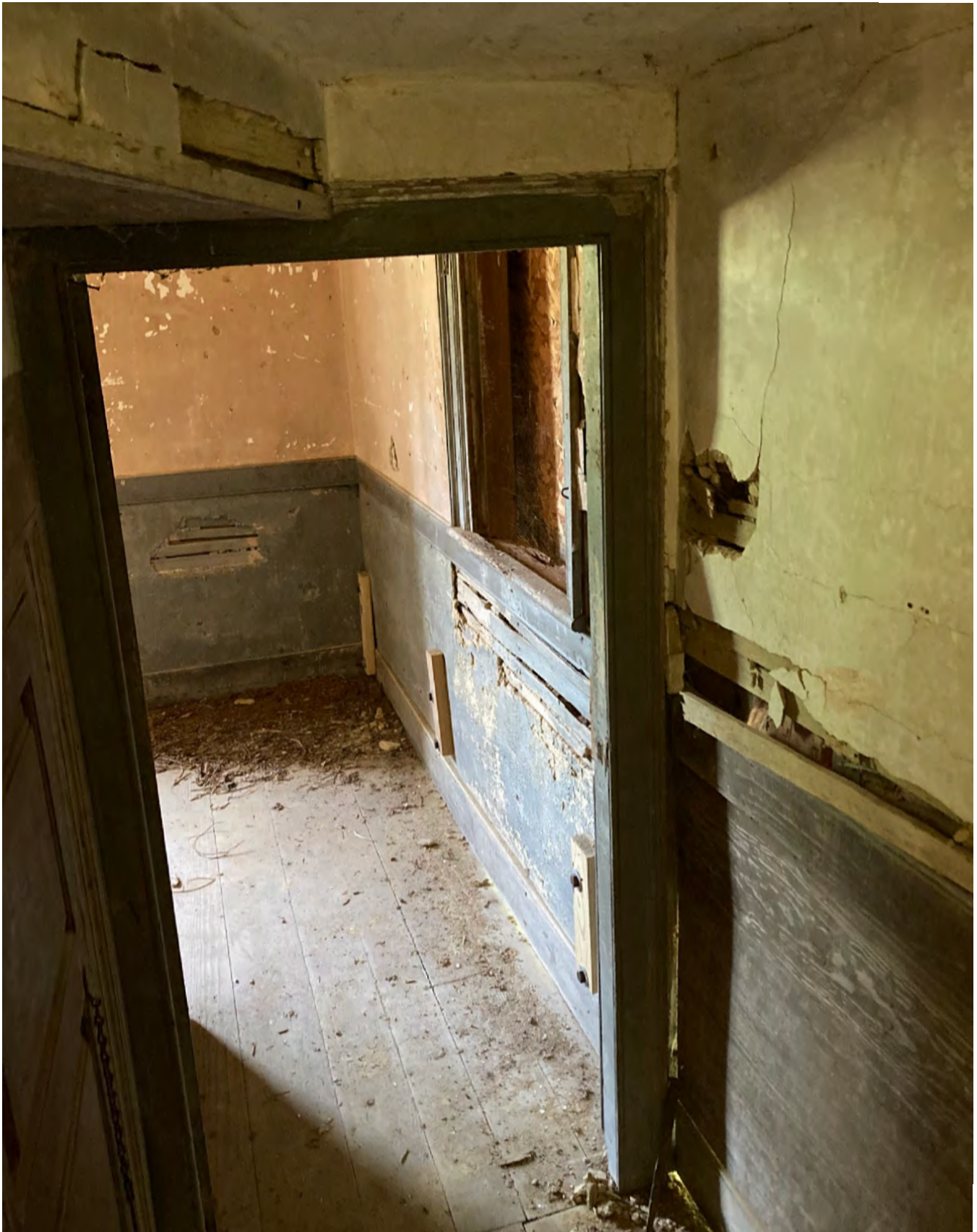
Looking west from Passage into Room 2 under stair landing.
