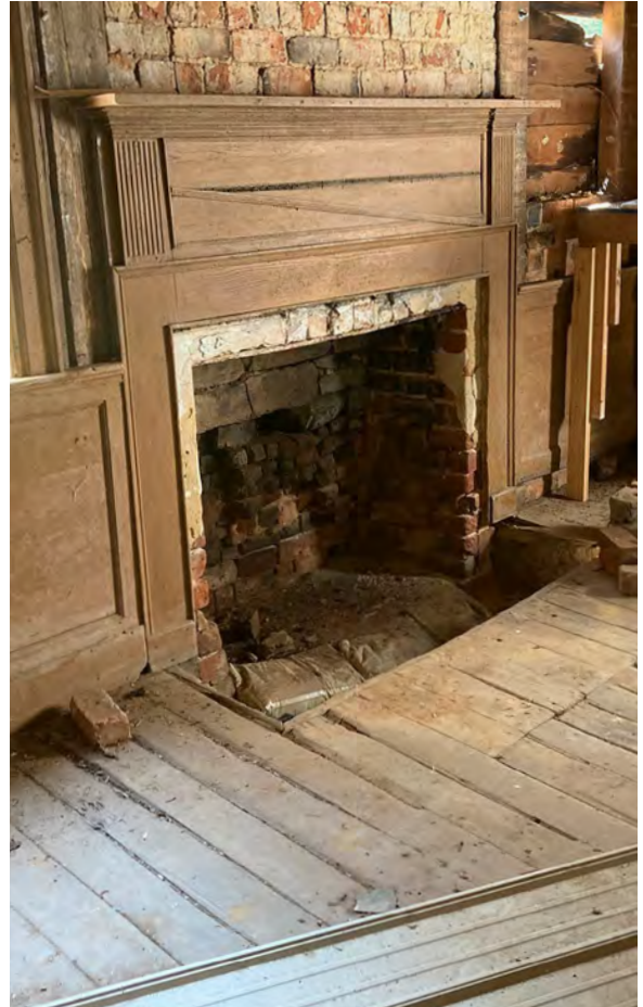
First Floor, Room 1) showing appearance before the floor was repaired c. 2013. The floor had dropped with the collapse of the rotted joists below (left). First Floor, Parlor, chimney breast showing damage to hearth, floor and fireplace interior (right).
