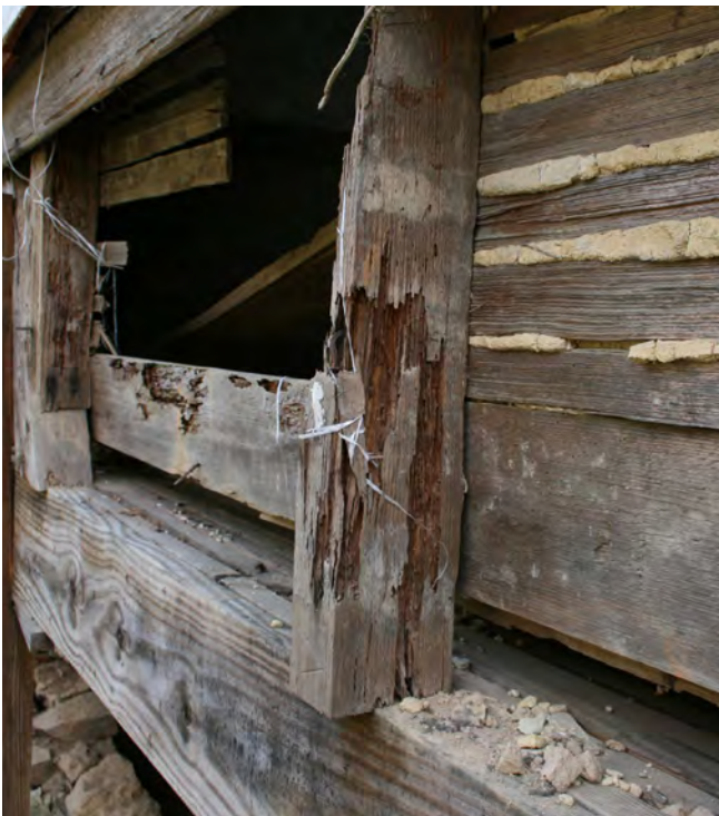
Damage to the sill on the north elevation (left) and typical brick nogging and weatherboards on the north elevation (right).
