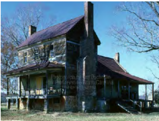
The hall-parlor form was widespread in late eighteenth century Virginia and North Carolina. For example, two such houses are found in Franklin County NC: the McLemore-Cannady House (to the left) has two doors on the primary façade for entry into each of two front rooms. [Megan Funk, Comprehensive Survey of Franklin County, 2018]
