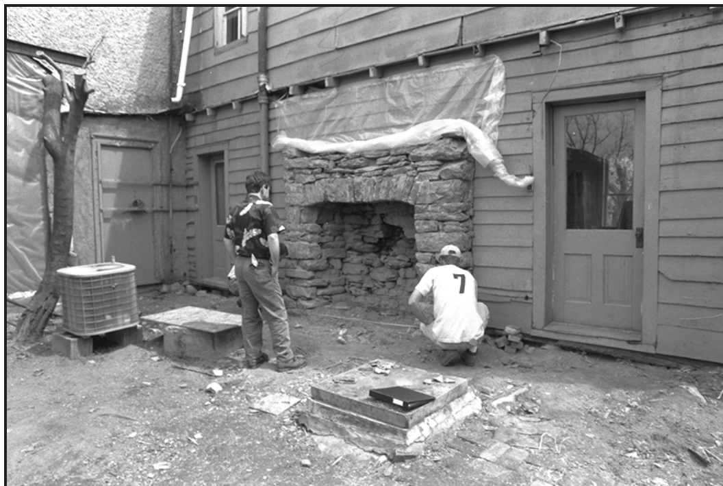
Figure 12. Site 44FK528, exterior (possible kitchen) hearth, west gable.
