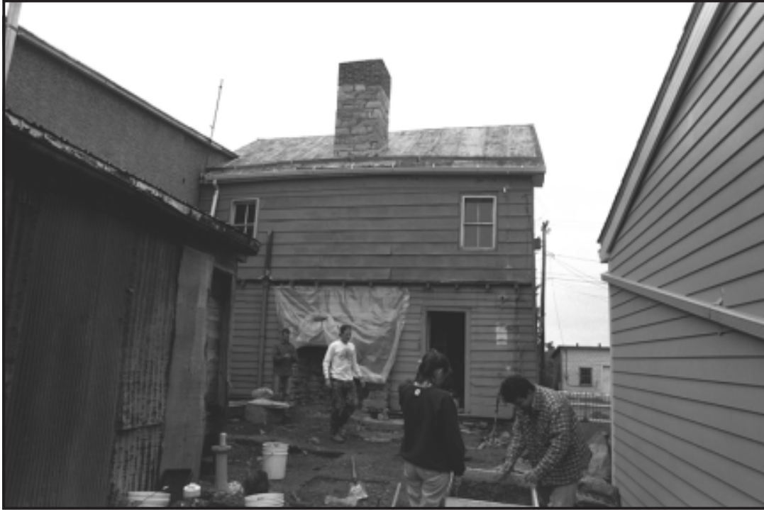
Figure 9. Andrew Pitman House, rear elevation and yard.
