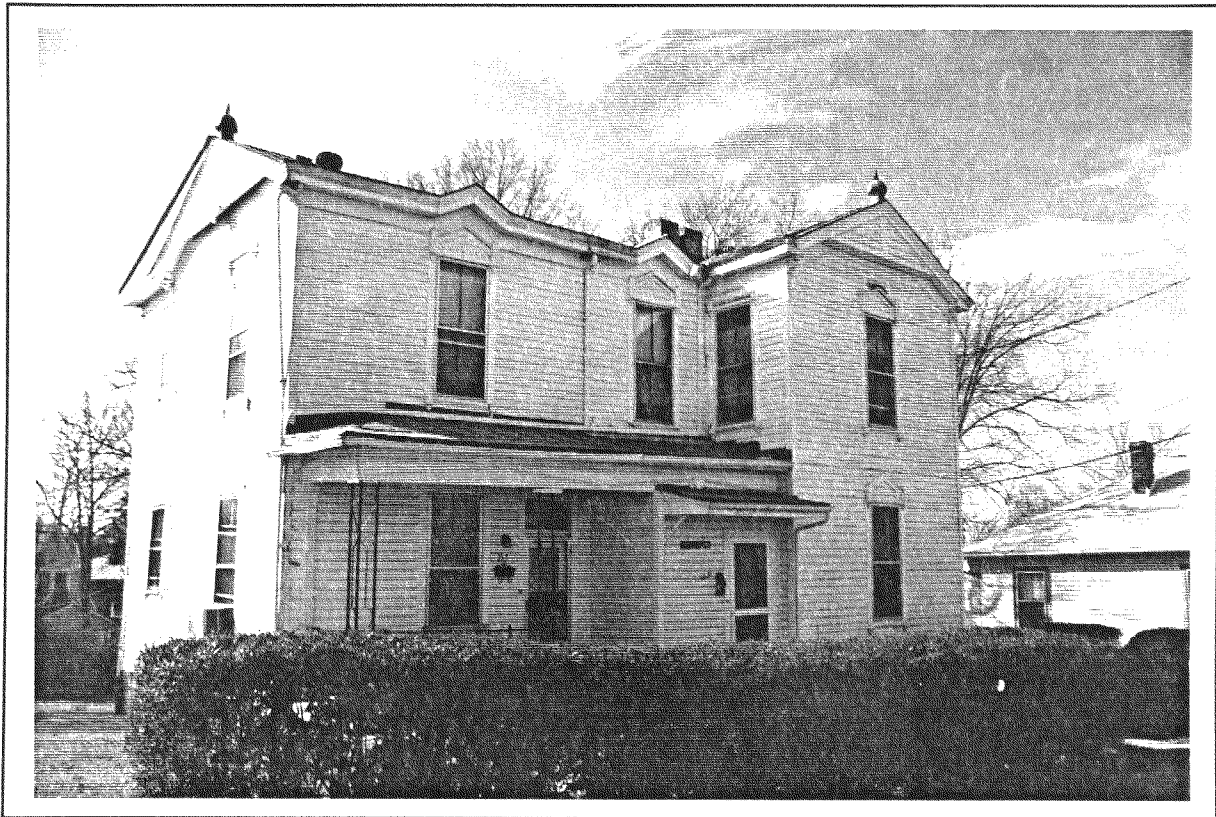
Figure 9. Sacred Heart Catholic Church Parsonage (108-221), 153 Holbrook Street.
