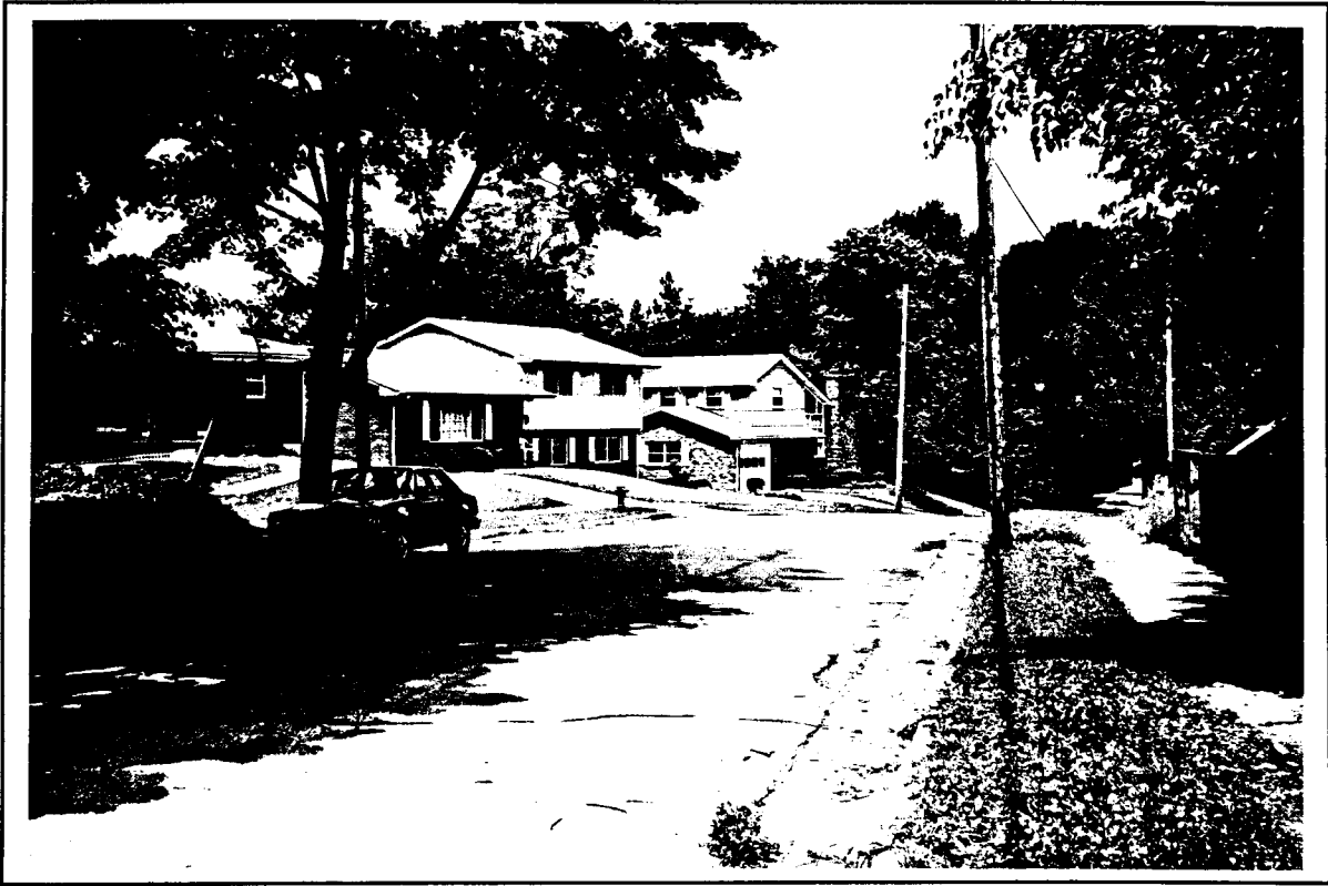
Figure 48. Example of non-contributing properties in the Holbrook-Ross study area.
