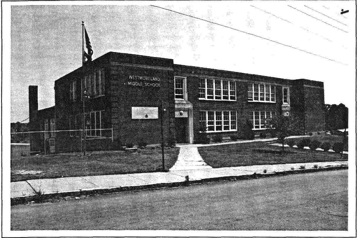
Figure 23. Westmoreland Middle School Building (108-180-001).
