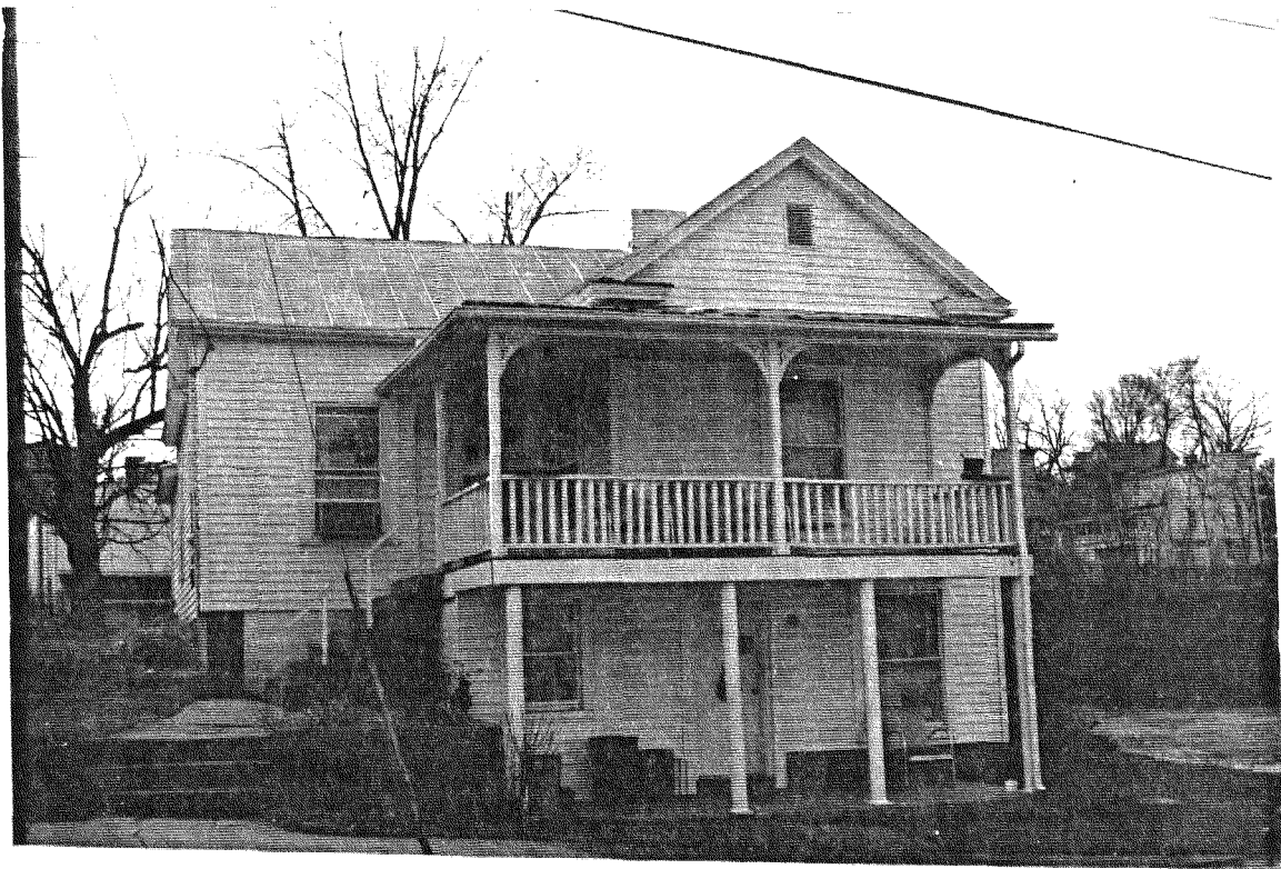
Figure 42. 317 North Floyd Street (108-0192).
