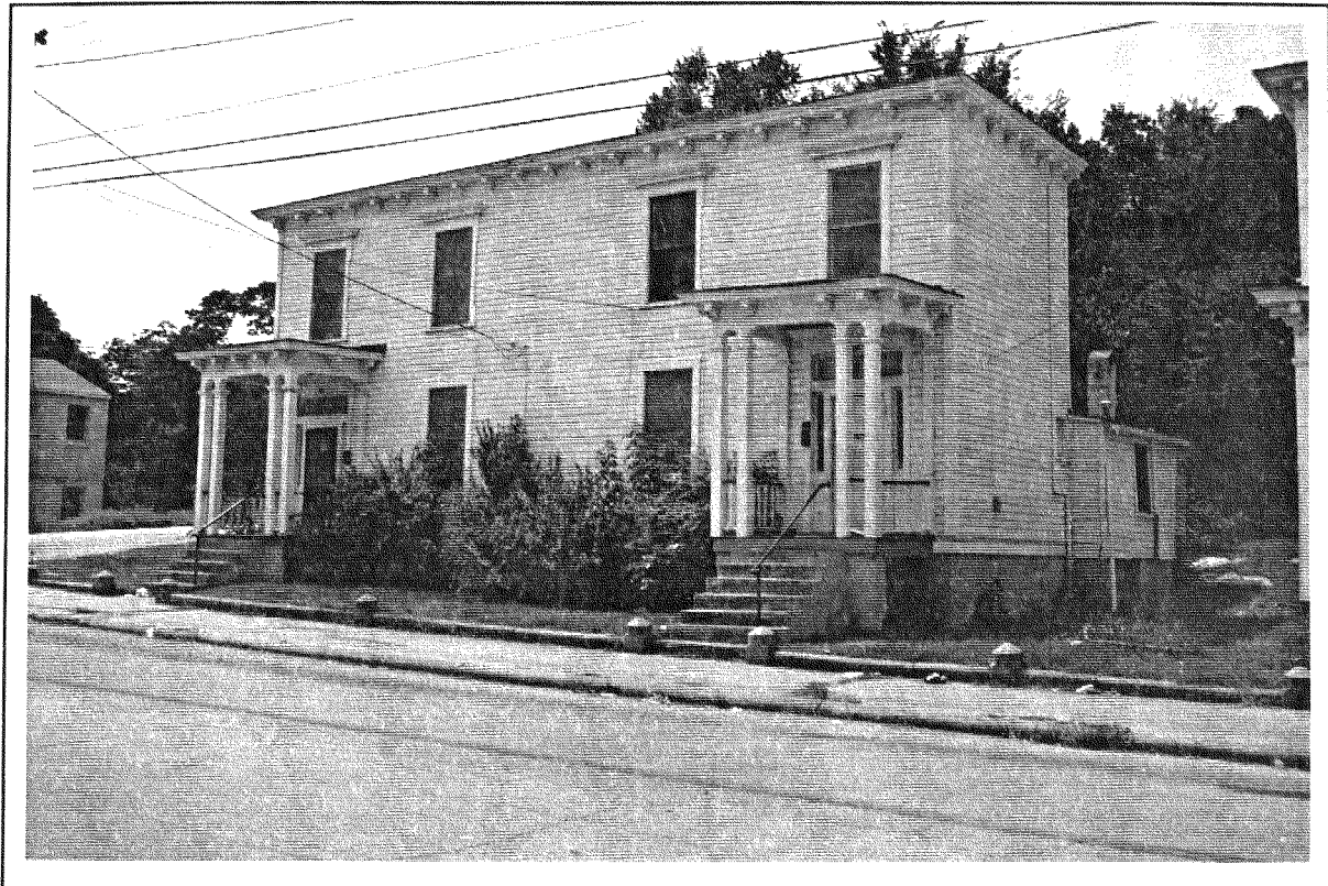
Figure 31. Example of the Italianate style. Duplex, 401-403 North Floyd (108-197).
