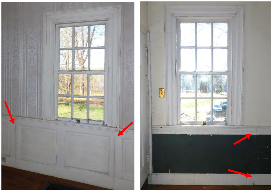
Figure 3: Break joints in the wainscot panels, chair rail, and baseboards below the windows on either end of the first and second floors of the Period I side passage indicate these areas were patched when historic doorways were infilled. Left: Period I First Floor Entry Hall, West Elevation. Right: Period I Second Floor Landing, East Elevation.
