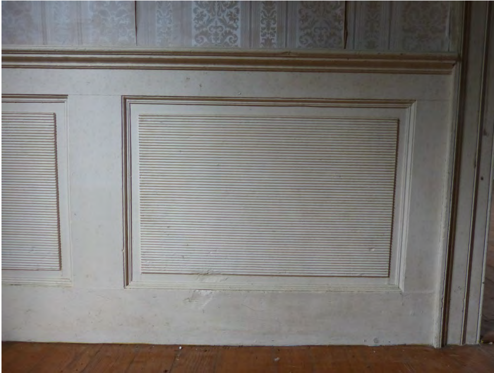
Figure 7: Period I Side Passage, reeded wainscot panels.
