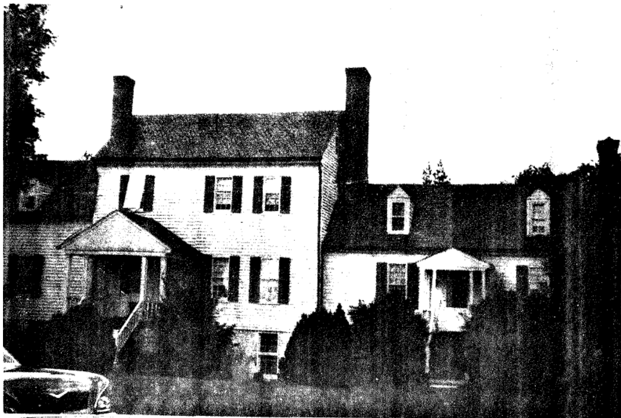
Figure 6: South Garden, 1958, facing west. HABS survey photo, courtesy of Virginia Department of Historic Resources.
