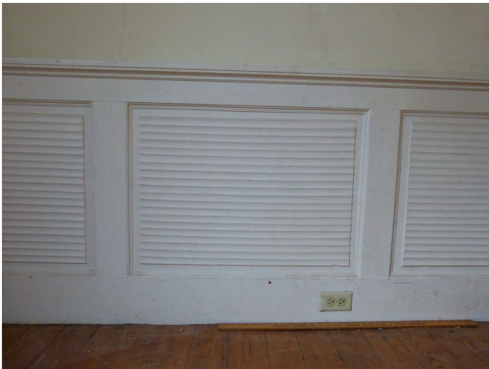
Figure 8: Period I Parlor, fluted wainscot panels.
