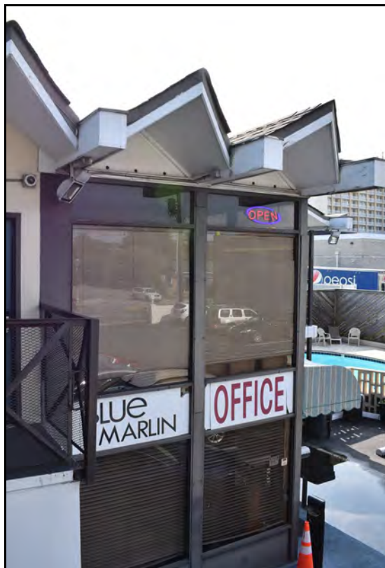
Figure 1. View of folded-plate roof over enclosed office, from second-floor level.
