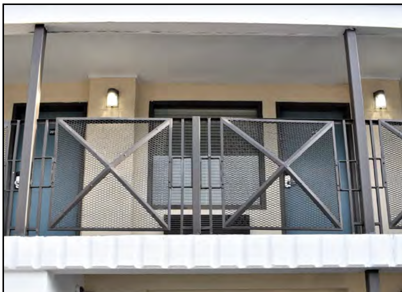
Figure 3. Detail of metal railing along second-floor balcony.
